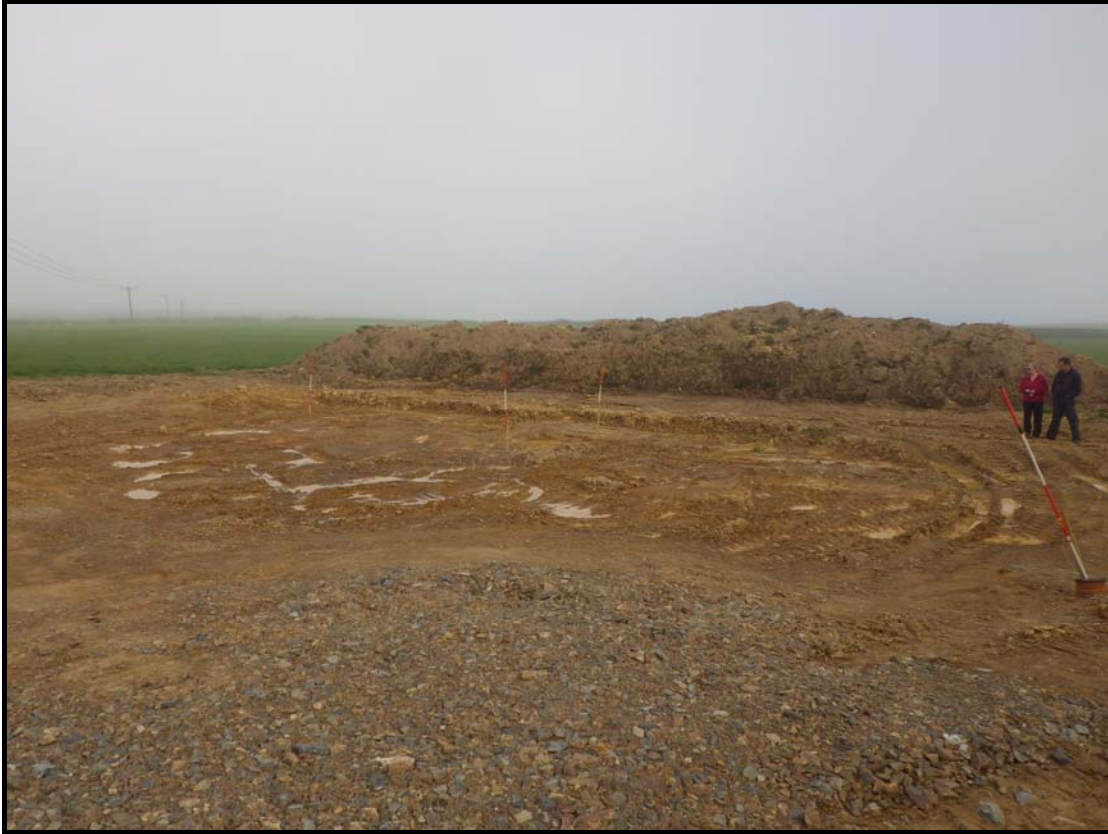
Plate 1: PZC2014_101, Area from which topsoil was removed prior to the watching brief with subsoil exposed, looking southeast.
