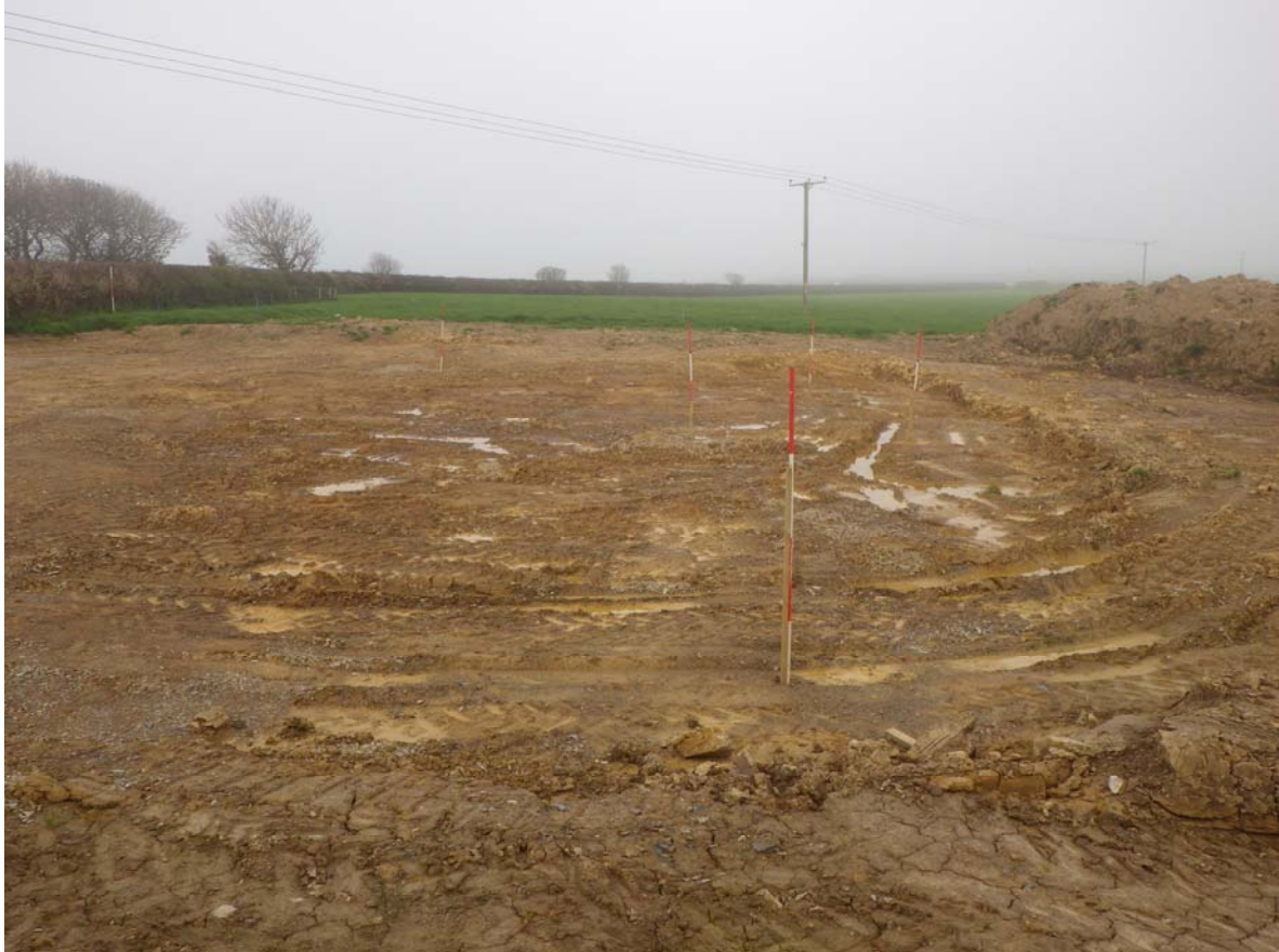
Plate 1: The groundworks undertaken prior to May 1st 2014, looking east.
