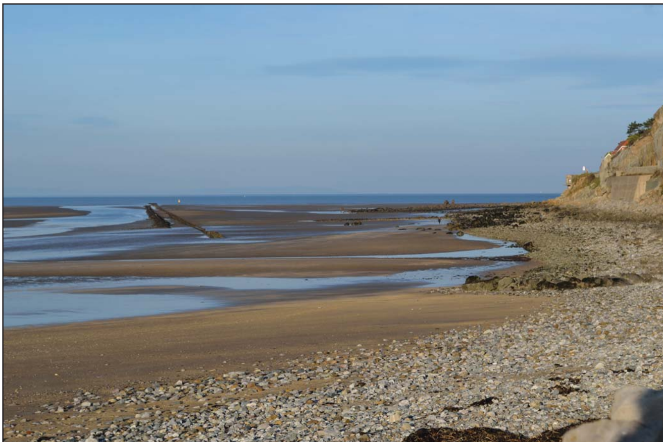
Plate 01: View of the outfall pipes from the shore; no scale: (archive reference: G2600_002).
