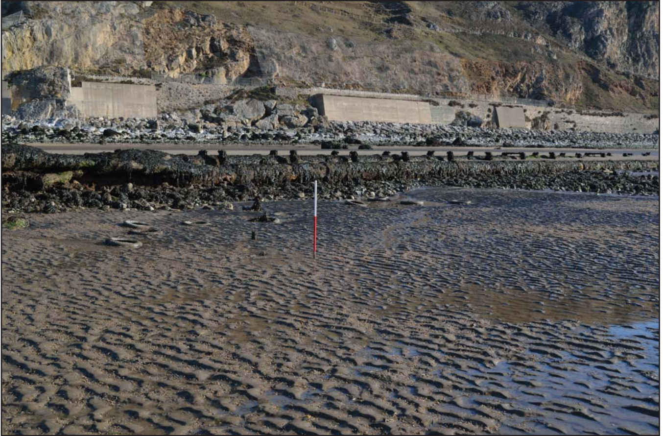
Plate 11: Possible fish trap (PRN 77164) and concrete repair; scale: 1x1m (archive reference: G2600_020).
