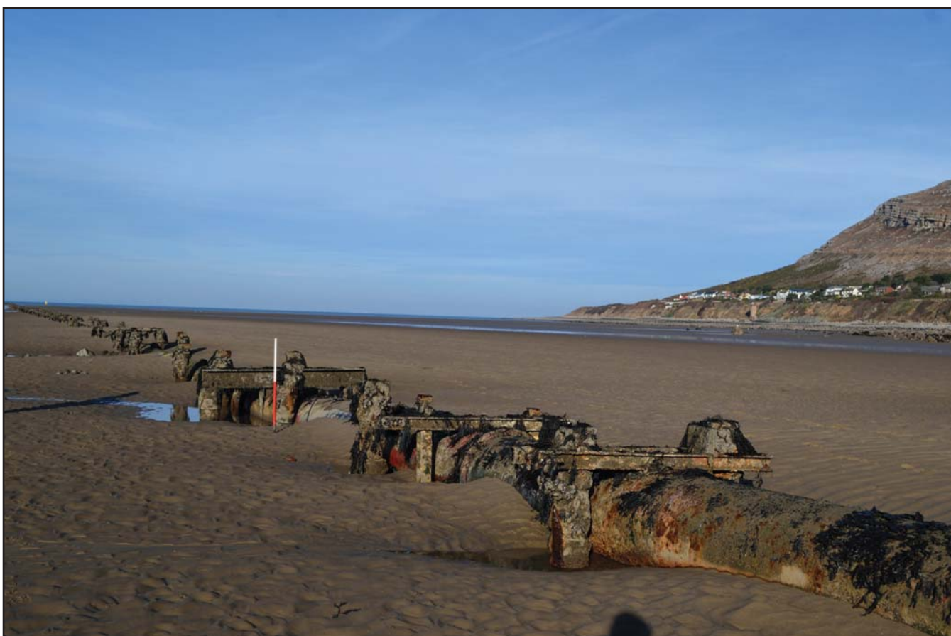
Plate 08: Location of 2013 repair to 1876 pipe; scale: 1x1m (archive reference: G2600_016).
