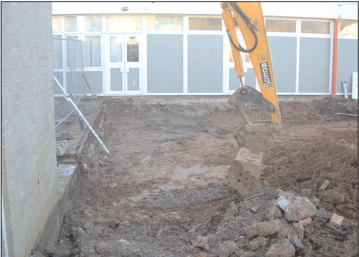
Plate 2 Looking west at excavation work next to existing school buildings
