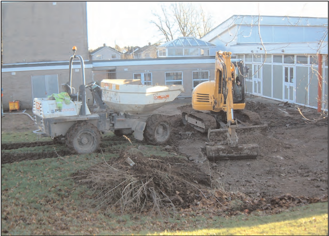
Plate 1 Looking south west at commencement of mechanical excavation work
