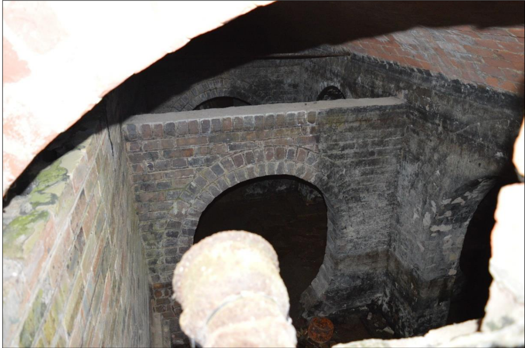
Fig. 8 The interior of the tank. Photo CPAT 4602-0012
