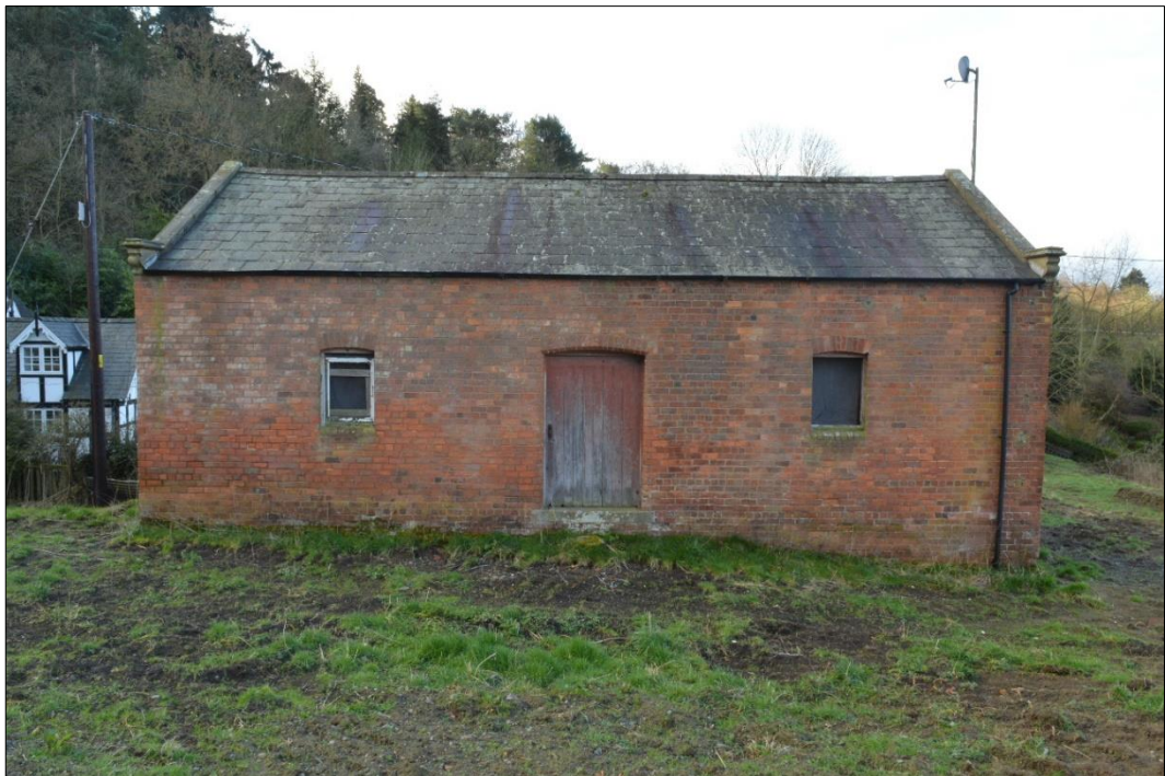
Fig. 5 The rear elevation of the Tank House. Photo CPAT 4602-0008
