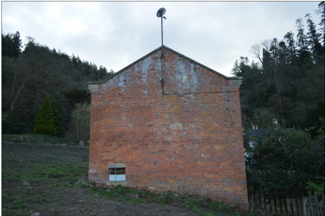
Fig. 6 The west elevation of the Tank House. Photo CPAT 4602-0005
