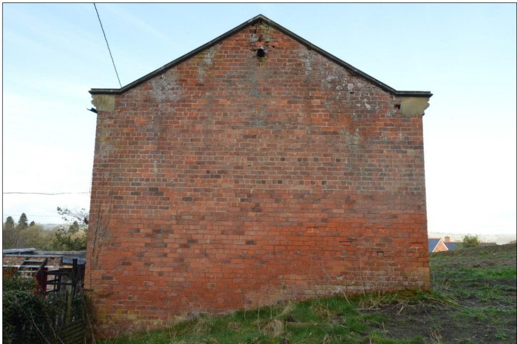
Fig. 9 The east elevation of the Tank House. Photo CPAT 4602-0009
