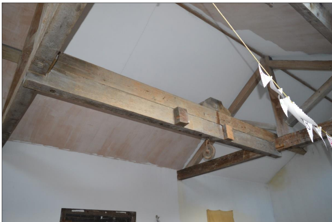
Fig. 10. CPAT Image 4602-0015 showing the beam arrangement.
