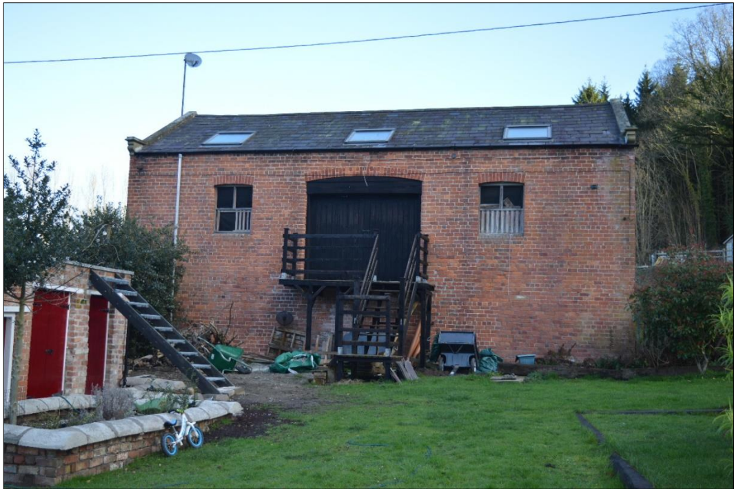
Fig. 4 The front elevation of the Tank House. Photo CPAT 4602-0001
