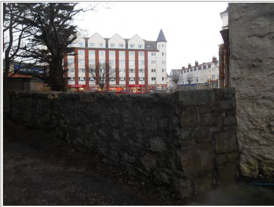
Plate 44. Detail of circuit wall.
