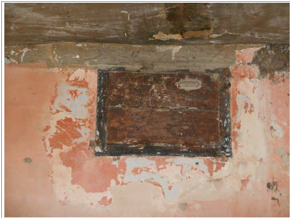
Plate 14. Possible vent, west facing wall.
