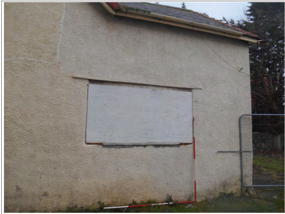
Plate 32. 1960's Window with hood. Pebble dashed wall, east facing. Scales 2 x 2m
