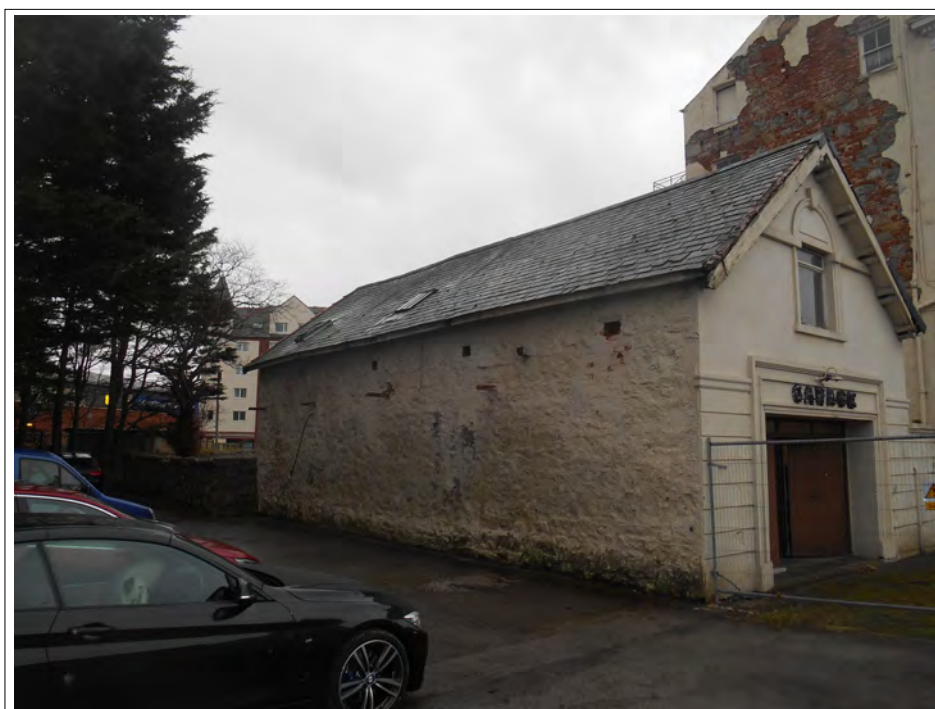
Plate 42. Detail of roof.
