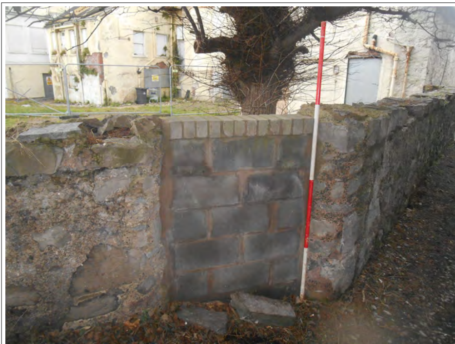
Plate 45. Modern alteration of circuit wall. Scale 2m
