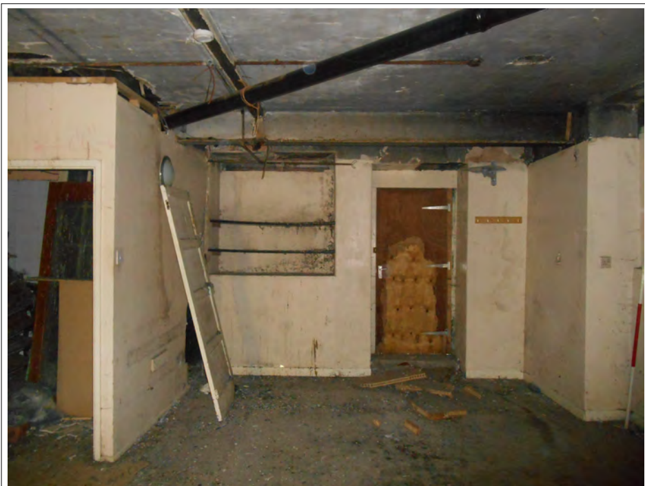
Plate 10. North facing wall. Inset blocked window transformed into shelving.
