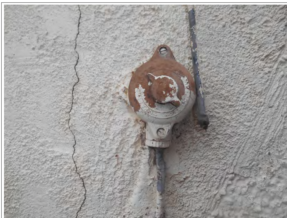
Plate 30. Detail shot of switch.
