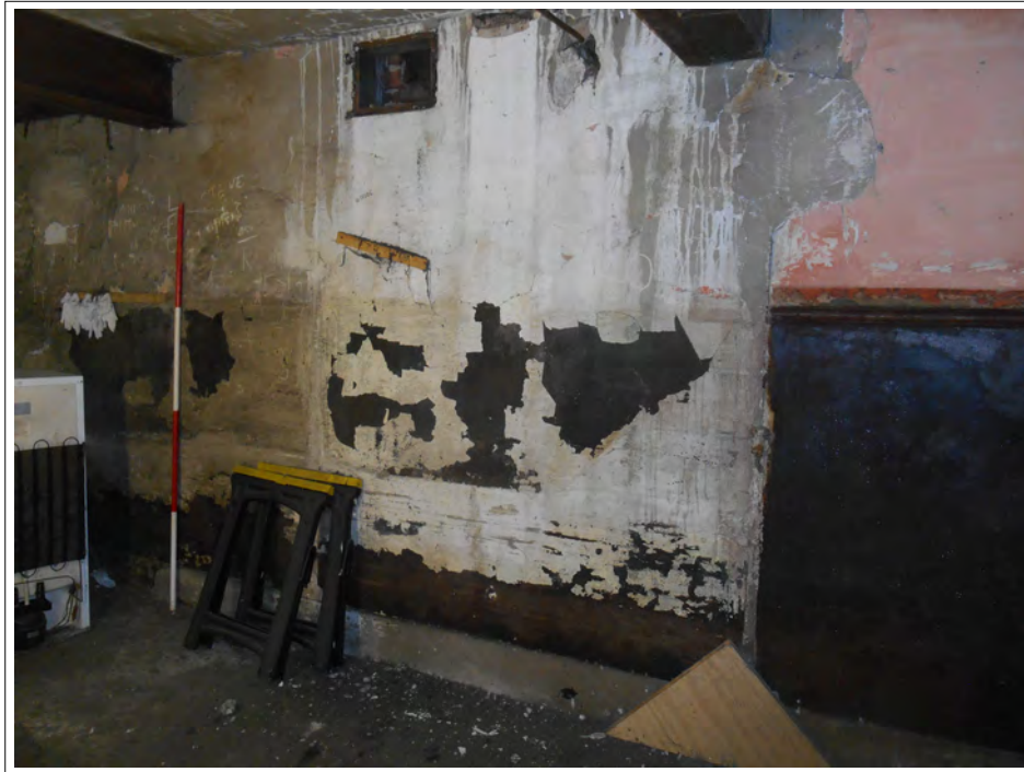
Plate 15. West facing wall. Scale 2m
