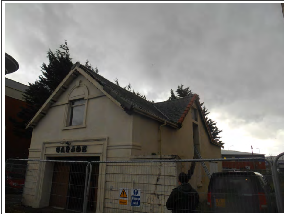
Plate 19. View of garage facade.
