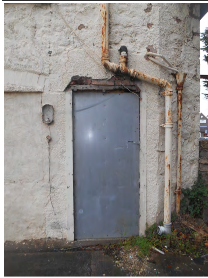
Plate 27. Detail of door associated to internal studded wall room.
