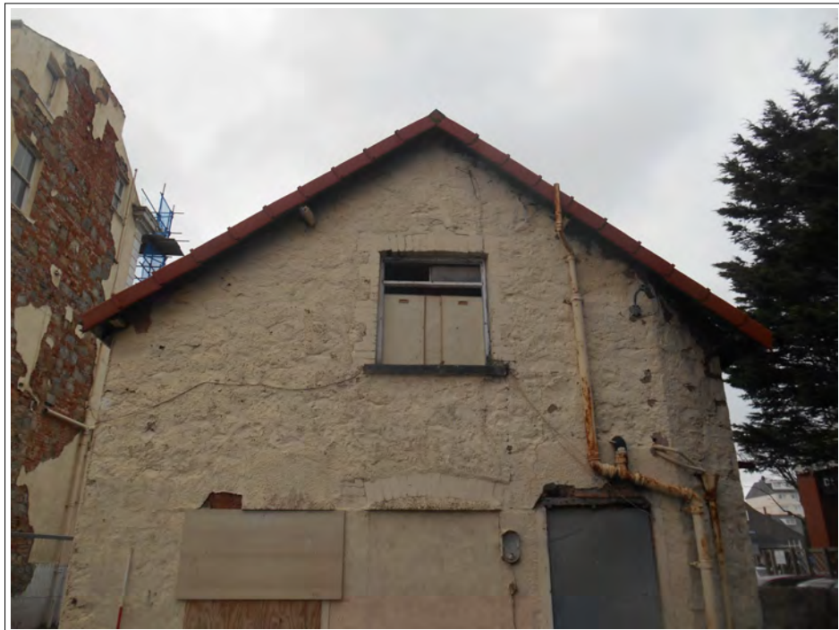
Plate 28. Detail of first floor window.
