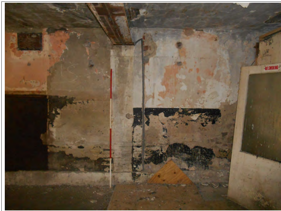
Plate 12. West facing wall. Scale 2m
