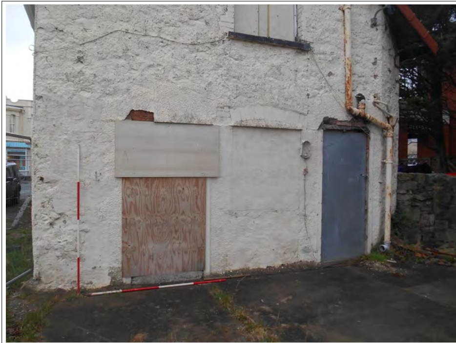
Plate 25. Detail of back entrances
