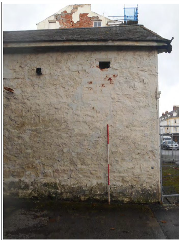
Plate 22. Detail of repair or alteration of possible window or vent. Scale 2m
