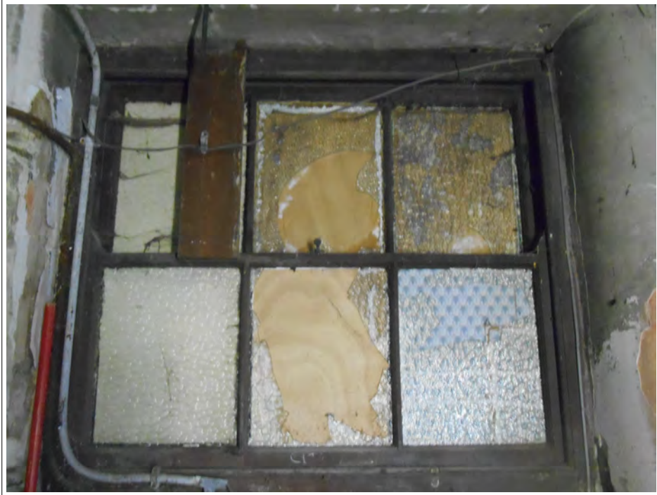
Plate 7. Detail of sash window. Eastern facing interior wall.
