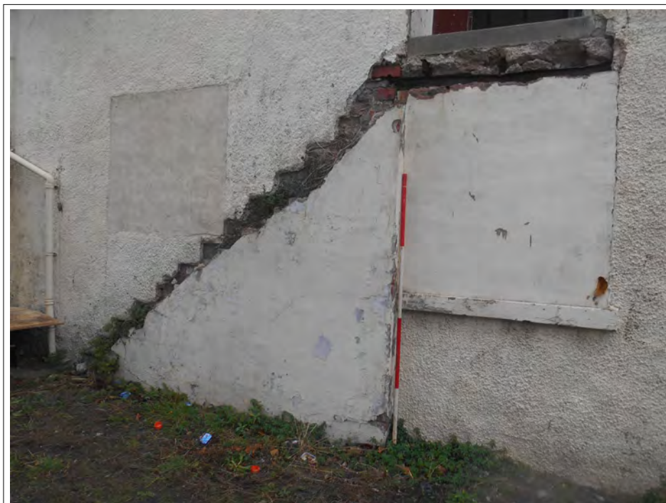
Plate 40. Detail of exterior stair case and doorway/window. Scale 2m
