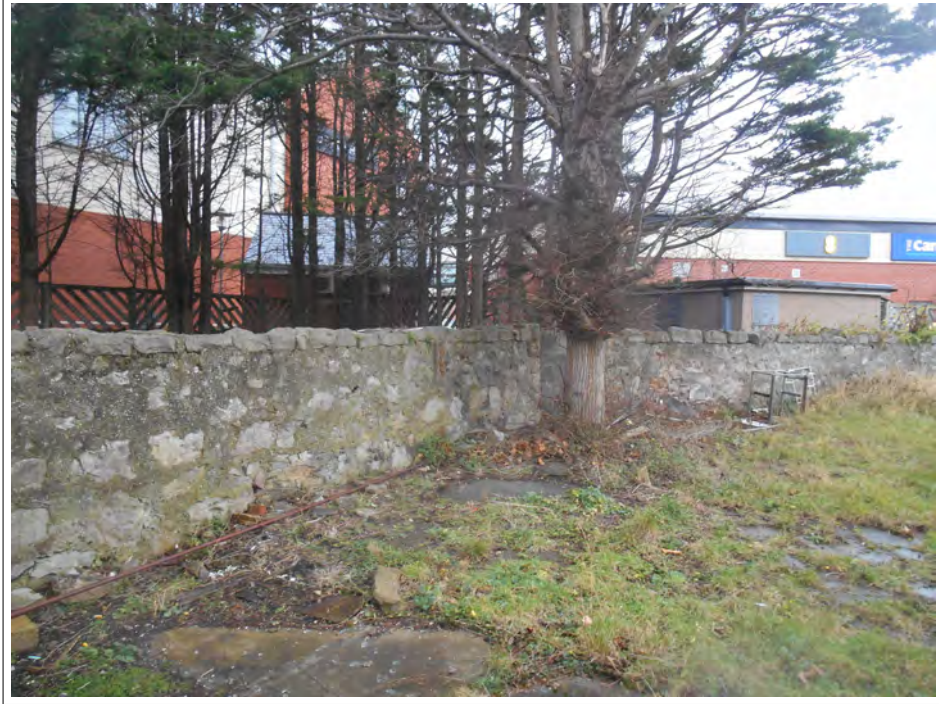
Plate 47. Detail of circuit wall viewed from back entrance.
