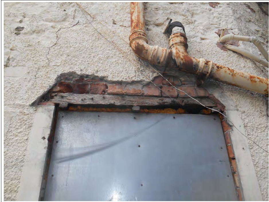
Plate 31. Detail of wooden lintel.
