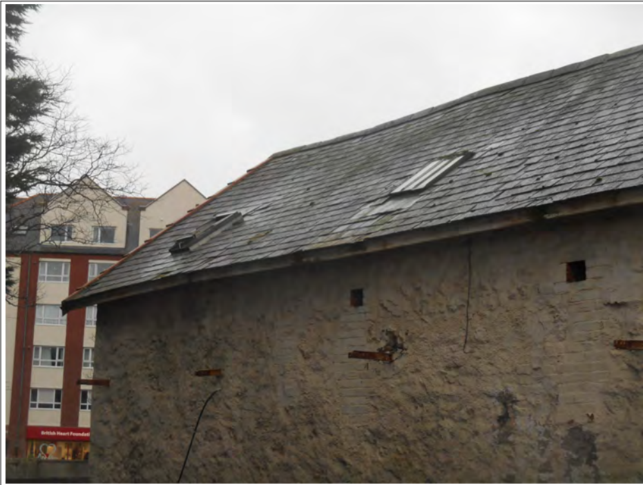
Plate 43. Detail of roof.
