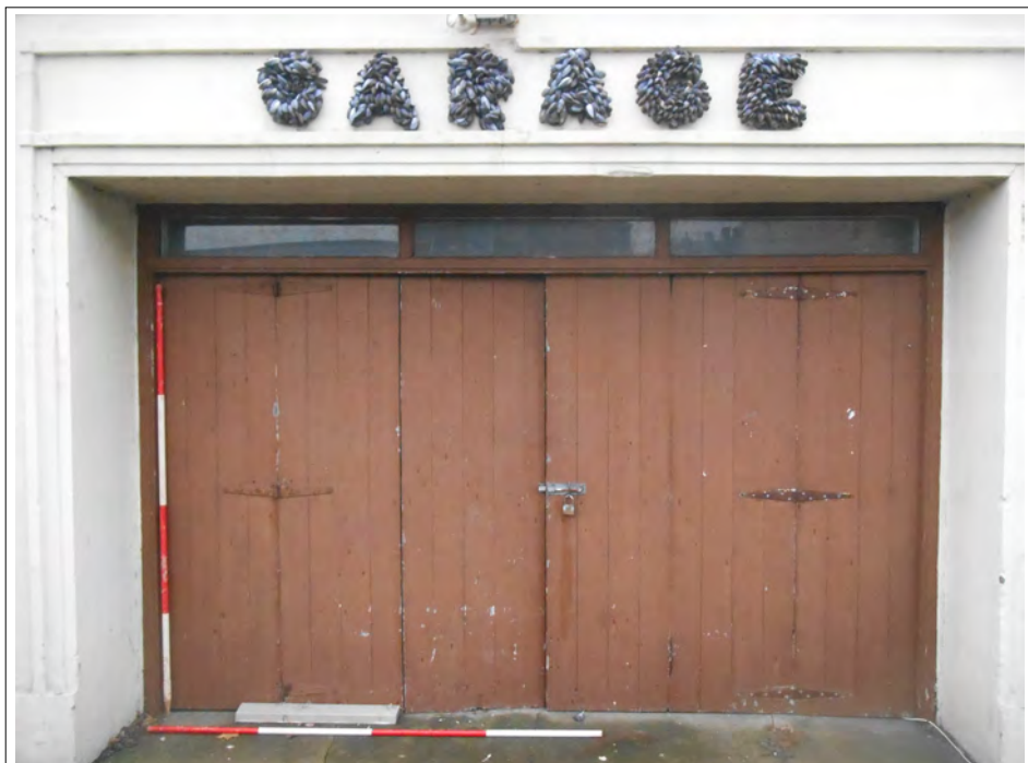
Plate 2. Main garage entrance. Looking south. Scales 2 x 2m
