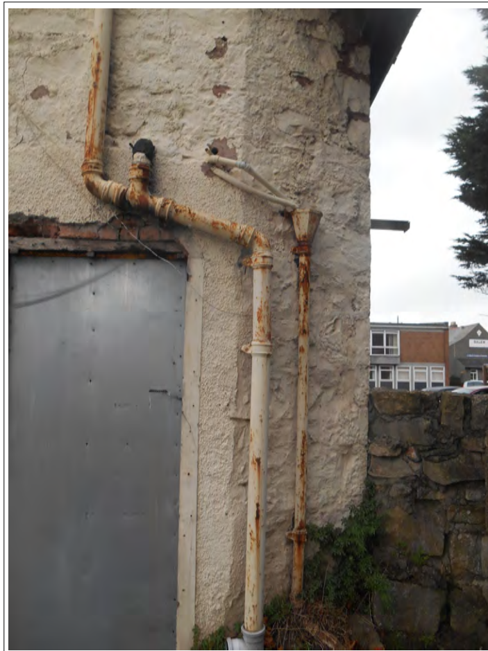
Plate 29. View of cast iron guttering.
