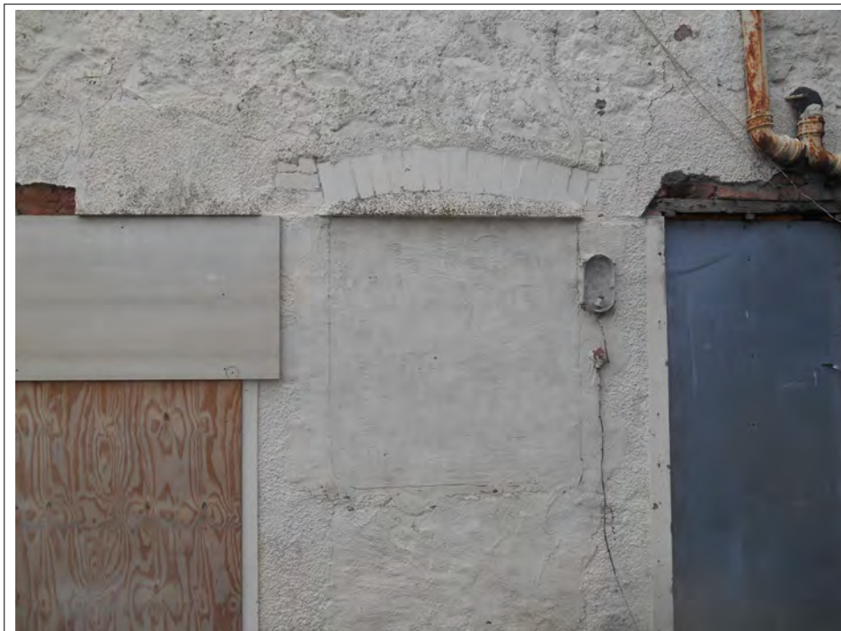
Plate 26. Detail of window hood.
