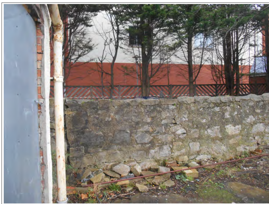
Plate 46. Circuit wall viewed from back entrance.
