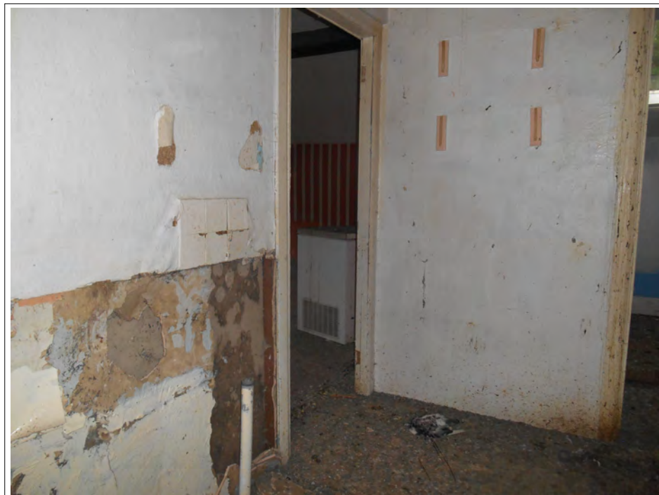
Plate 36. First floor, looking north.
