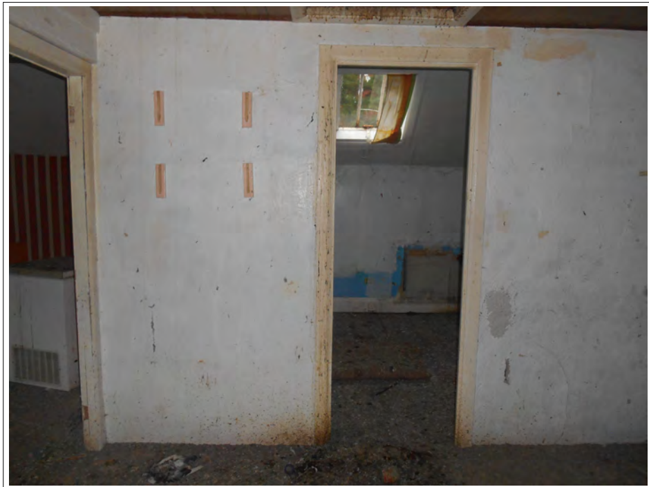
Plate 34. First floor, looking west
