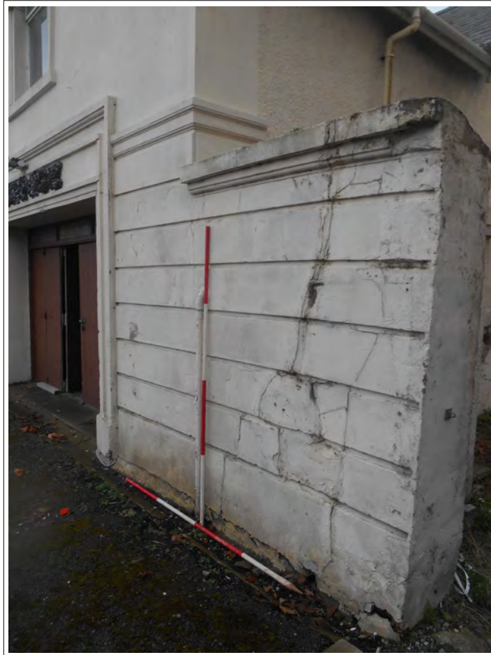
Plate 1. View of western wall of facade. Looking south. Scales 2 x 2m
