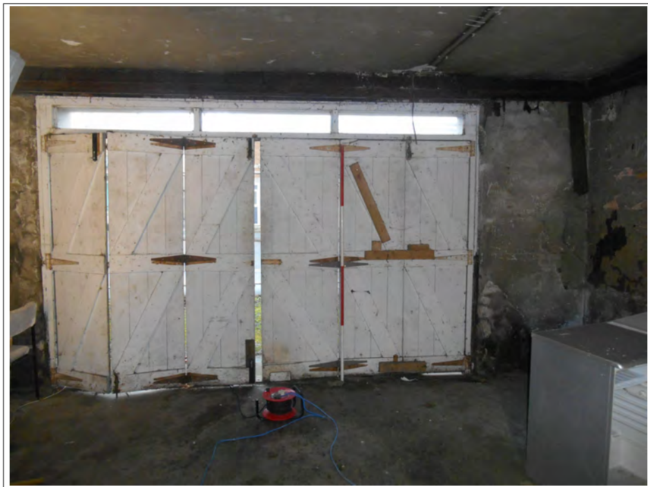
Plate 18. View of entrance from inside. Scale 2m
