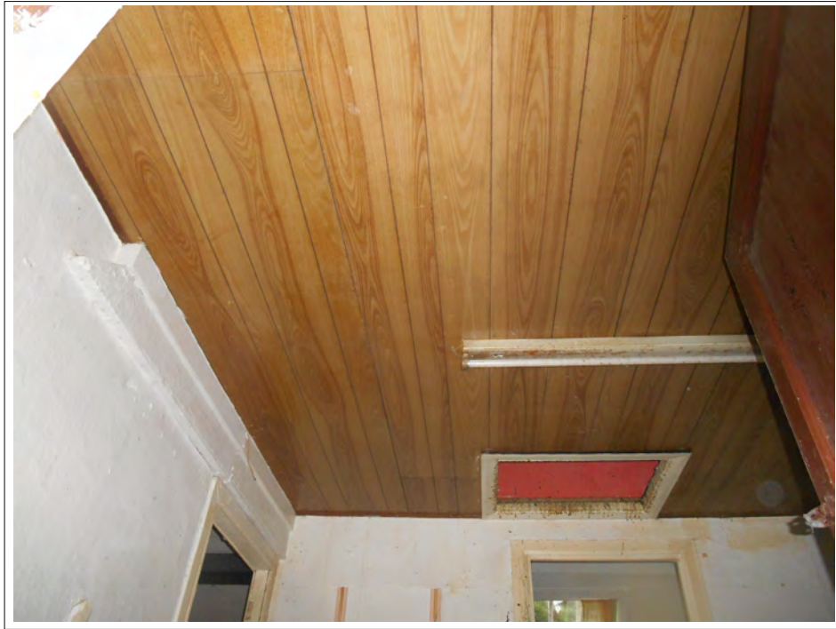
Plate 37. First floor sealing.
