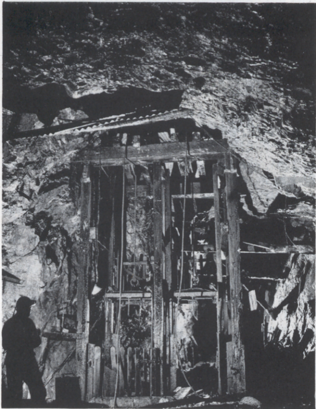
Figure 4. Underground headframe in the deep adit.
