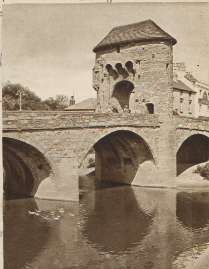
MONNOW BRIDGE, MONMOUTH
