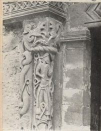
KILBECK CHURCH, DETAIL OF THE SOUTH DOOR
