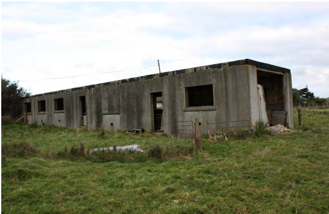
Figure 22: One of the remaining military camp buildings (NPRN 404399)
