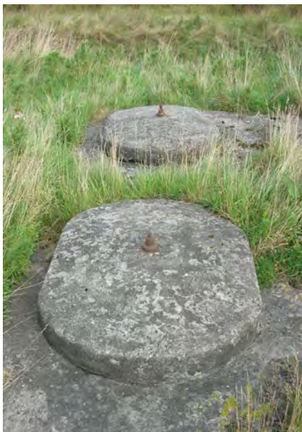
Figure 20: A camera/observation post built to a specification forwarded by the Experimental Establishment at Walton-on-the-Naze with concrete bases for Kine Theodolite or experimental radar (NPRN 408403-4, 506534)
