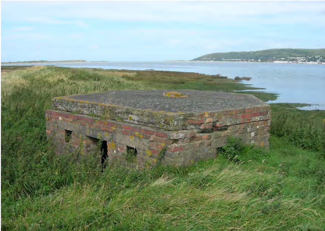
Figure 20: A camera/observation post built to a specification forwarded by the Experimental Establishment at Walton-on-the-Naze with concrete bases for Kine Theodolite or experimental radar (NPRN 408403-4, 506534)
