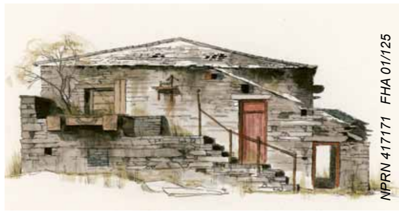
Right: Drum house to Rhiw-bach Quarry, 1981 This site sketch, dated 23 March 1981, shows the drum house at the top of the second incline taking slate trams to and from Rhiw-bach quarry, Blaenau Ffestiniog. It is an example of the use of slate waste to build sturdy structures.
