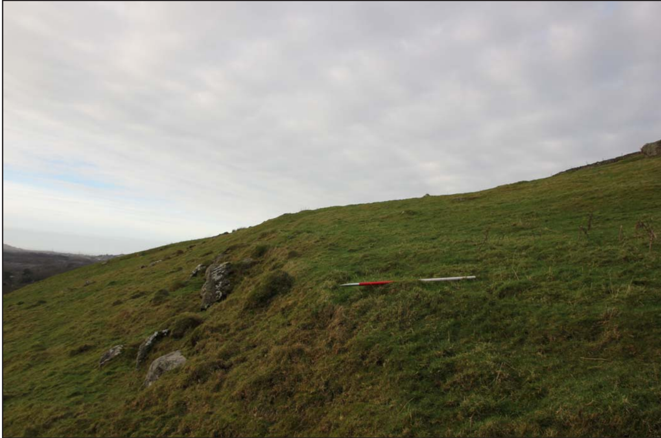
Plate 01: Relict revetment wall and trackway (feature 4), from the east. Scale 1.0m.
