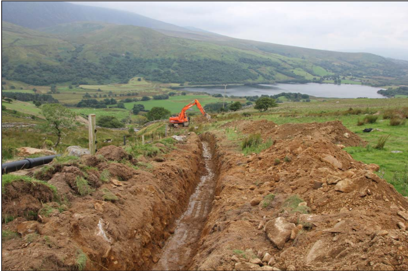
Plate 04: New hydro-electric pipeline trench, from the northeast.
