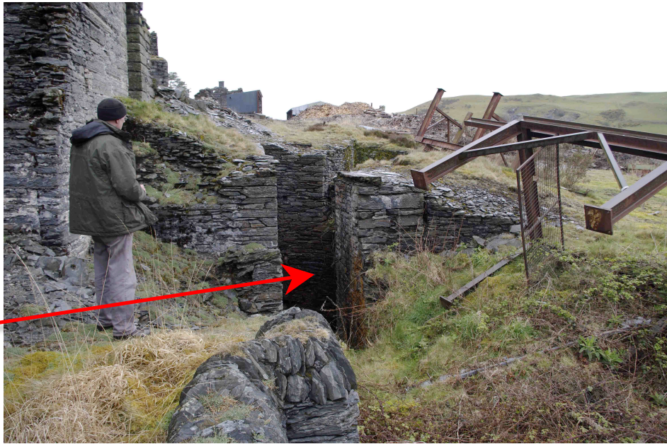
Photo No 3: View of shaft
