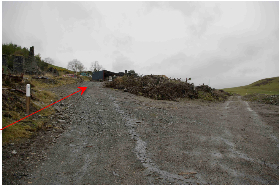
Photo No 1: View taken looking north-east from the diversion point. The diversion to the right is a safe route, the route straight on is the unsafe route passing the dangerous area on the left. The post in the left foreground has an arrow pointing to the route to the right but on the right-hand side of the post is an arrow pointing to the unsafe route.
