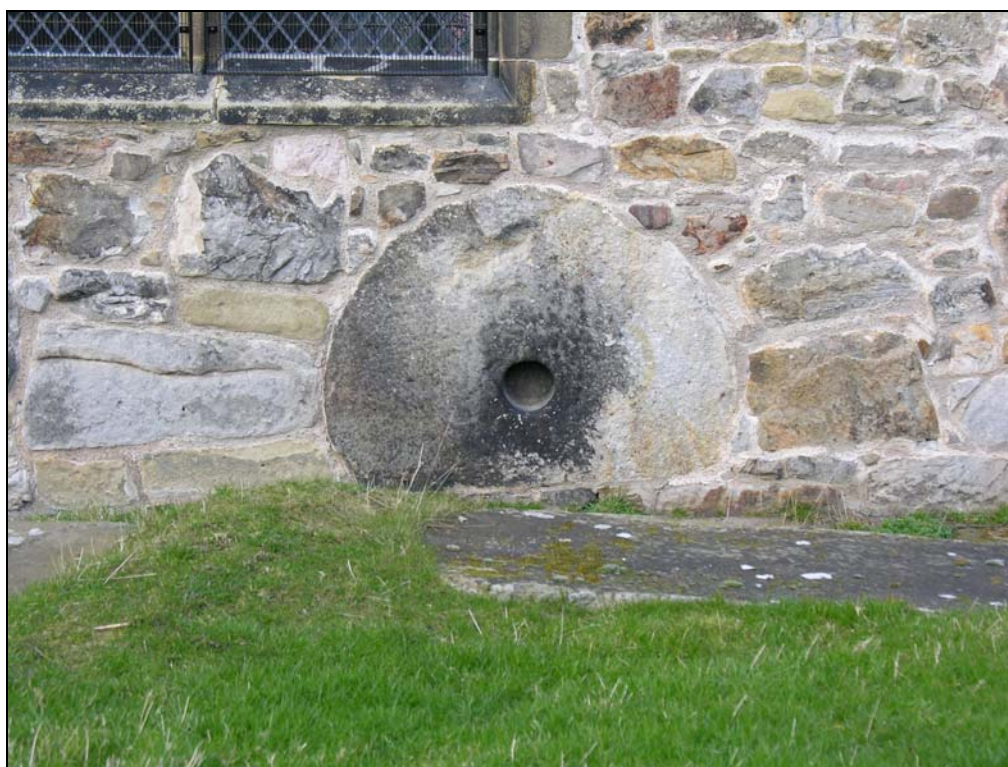
Fig 12: the south wall of Hope Church nr Wrexham exhibiting the secondary use of a millstone. © R J Silvester
