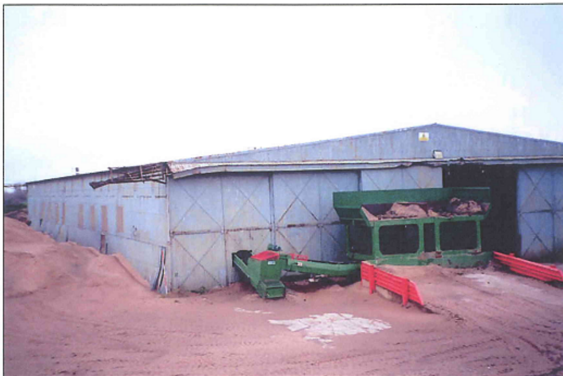
Plate 3: Bellman hangar at the former RAF Wrexham. Photo CPAT 900.9
