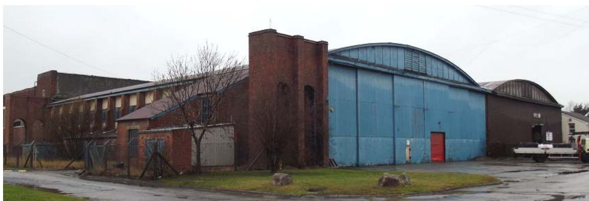
Plate 2: Listed General Service Shed (Belfast Truss Hangar) at the former RAF Sealand. Photo CPAT 3391-0042
