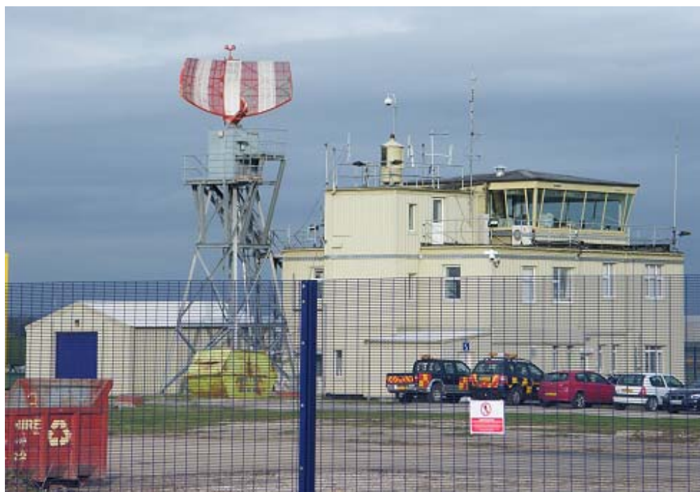
Plate 1: Fire Tender Shelter (L) and Control Tower at the former RAF Hawarden. Photo CPAT 3391-0121
