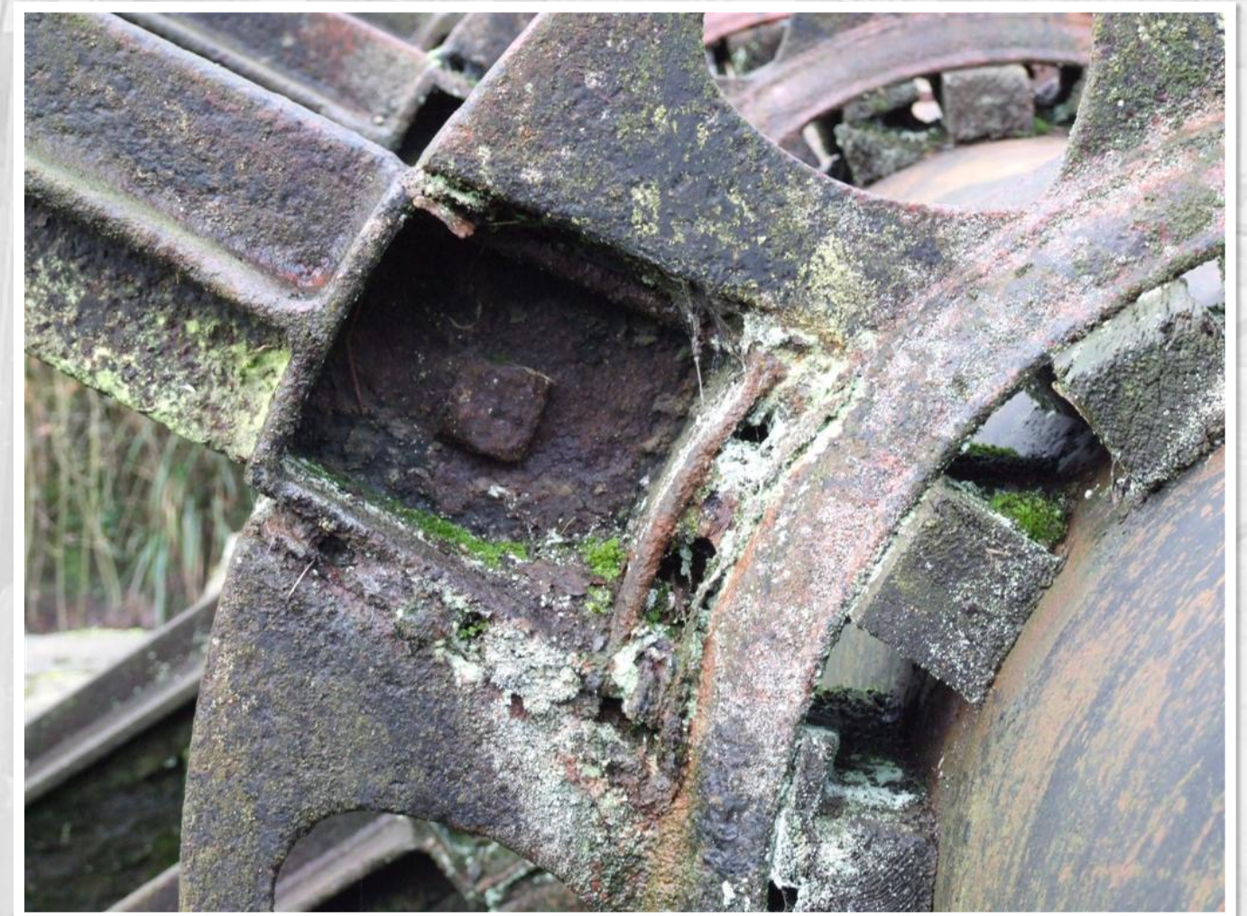
Fig 4 14/01/2009 Enlarged view showing the condition of the Wheel hub and shaft.
