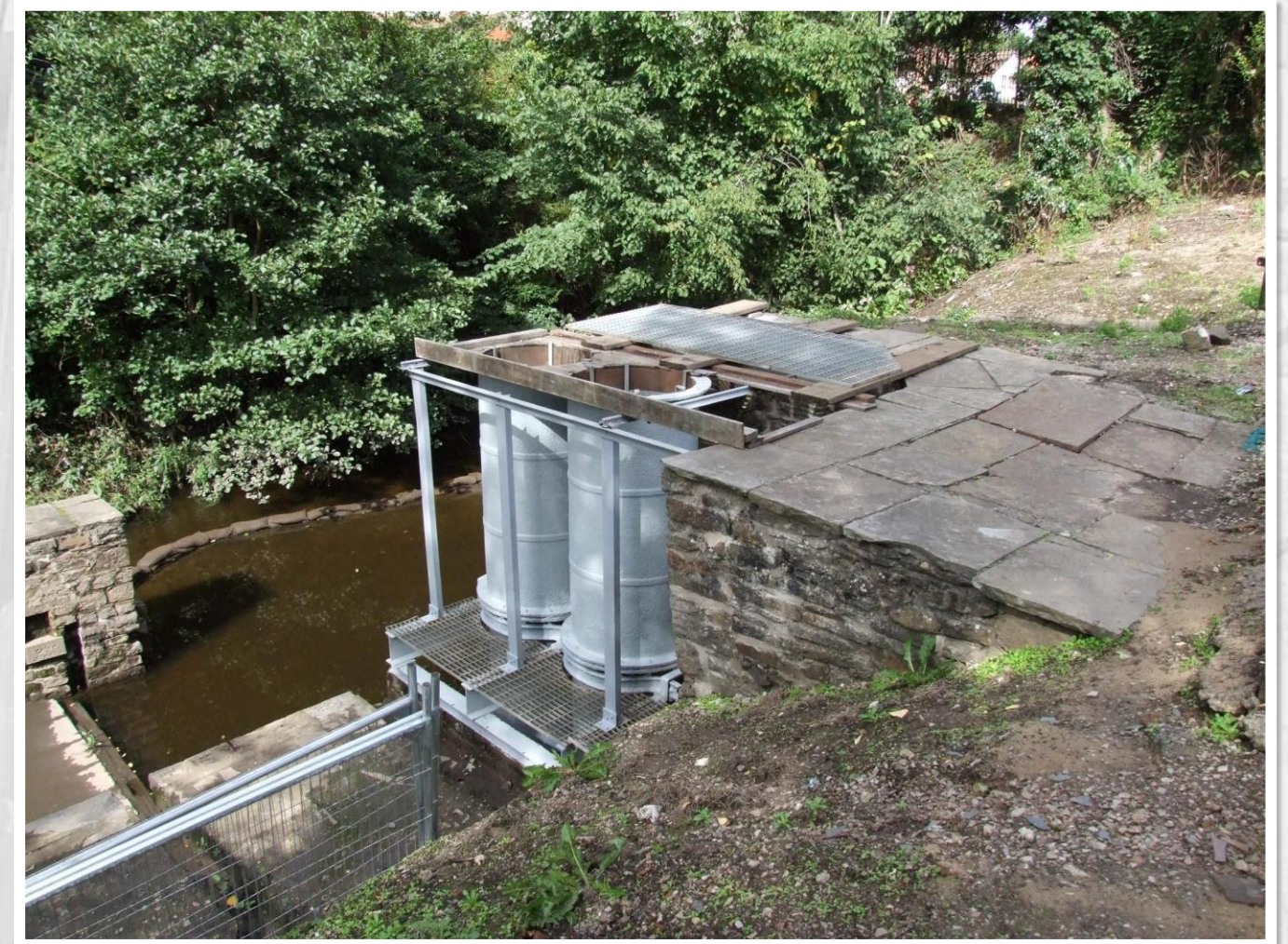
Fig 20 15/09/2010 Pump cylinders following cleaning by hand and coat of primer ready for decoration.
