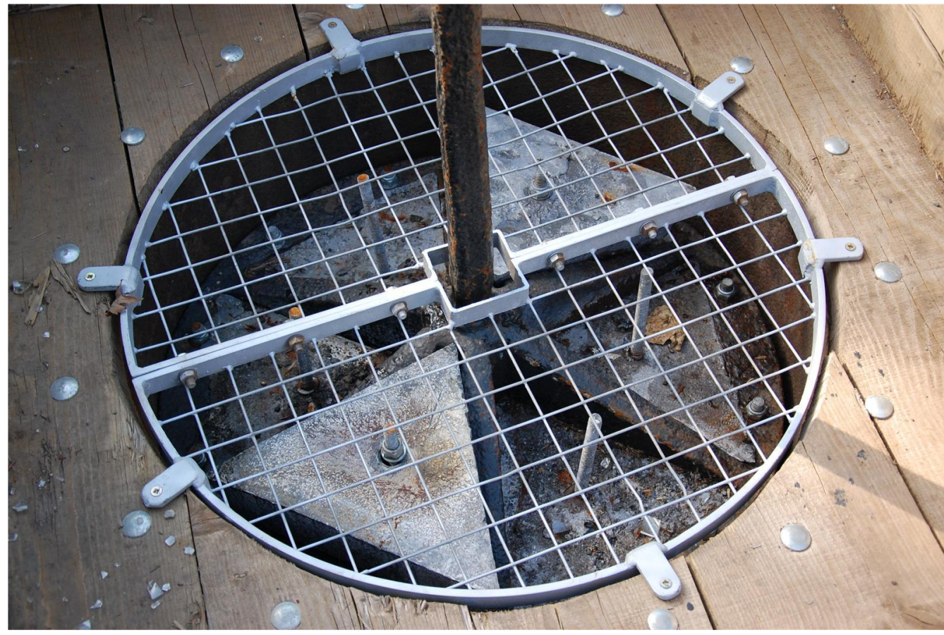
Fig 72 02/06/2011 Cast lead Counterbalance weight set within and on top of the original Valve Frames and Pump cylinders.
