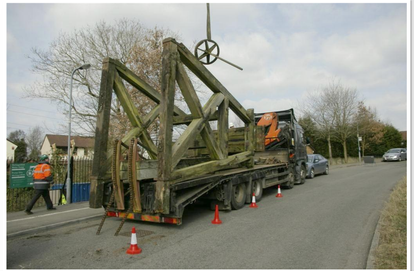
Fig 10 11/03/2010 Pump Valve and Lifting Rod being loaded onto transport.
