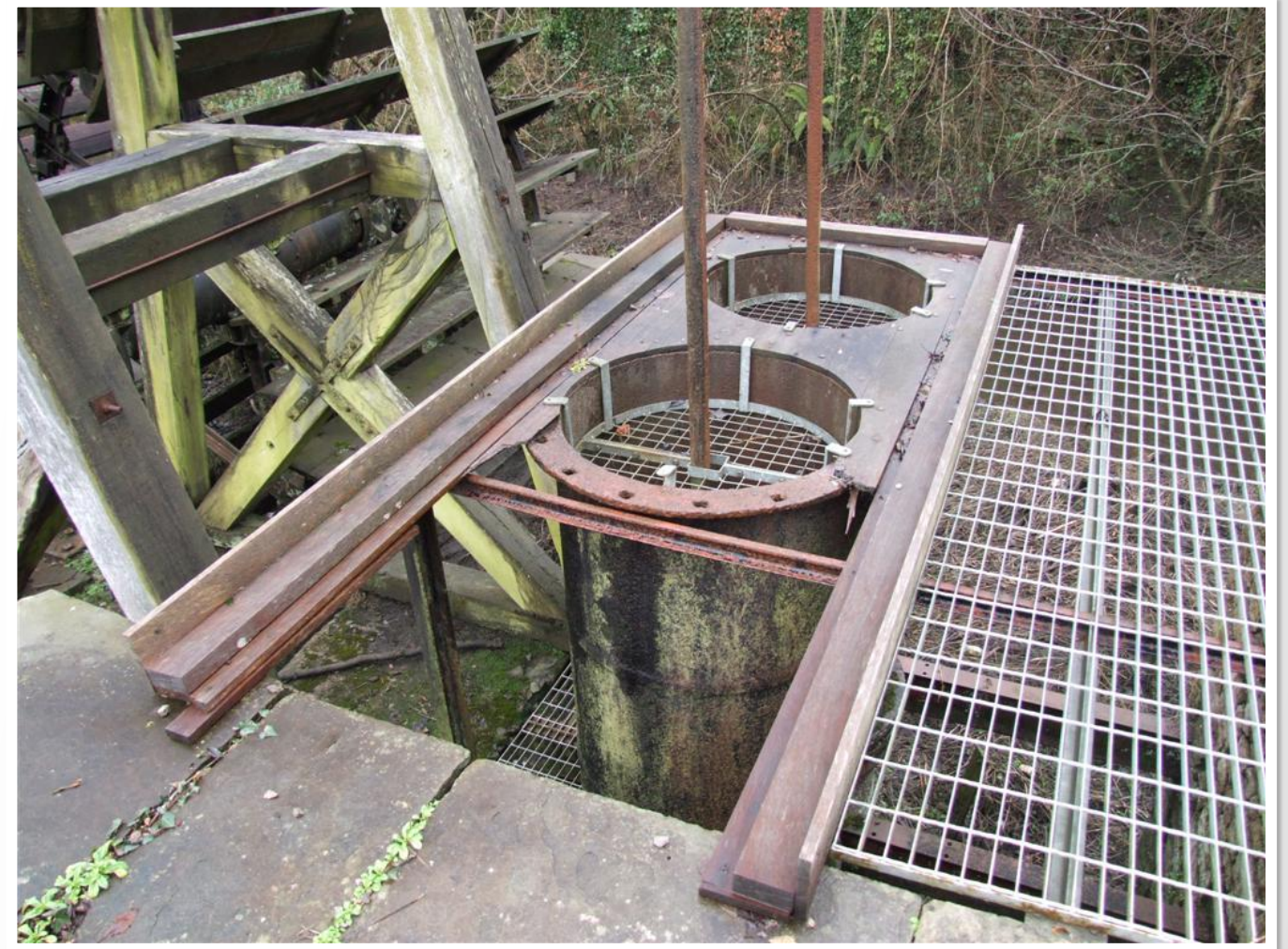
Fig 2 14/01/2009 Remains of the original timber Launder above the Pump cylinders.
