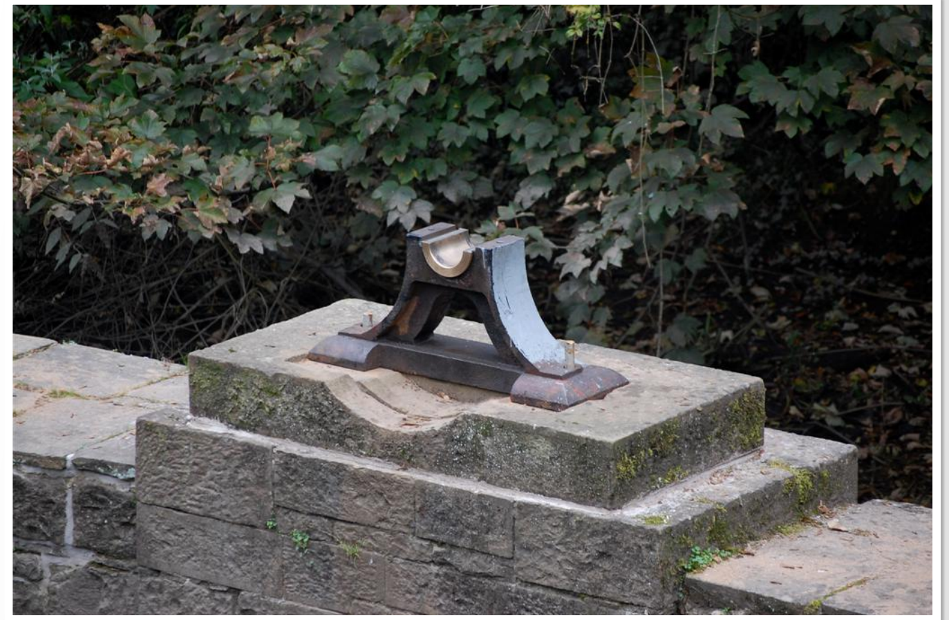
Fig 47 14/10/2010 Far-side bearing pedestal lowered into position. Note new bronze bearings.
