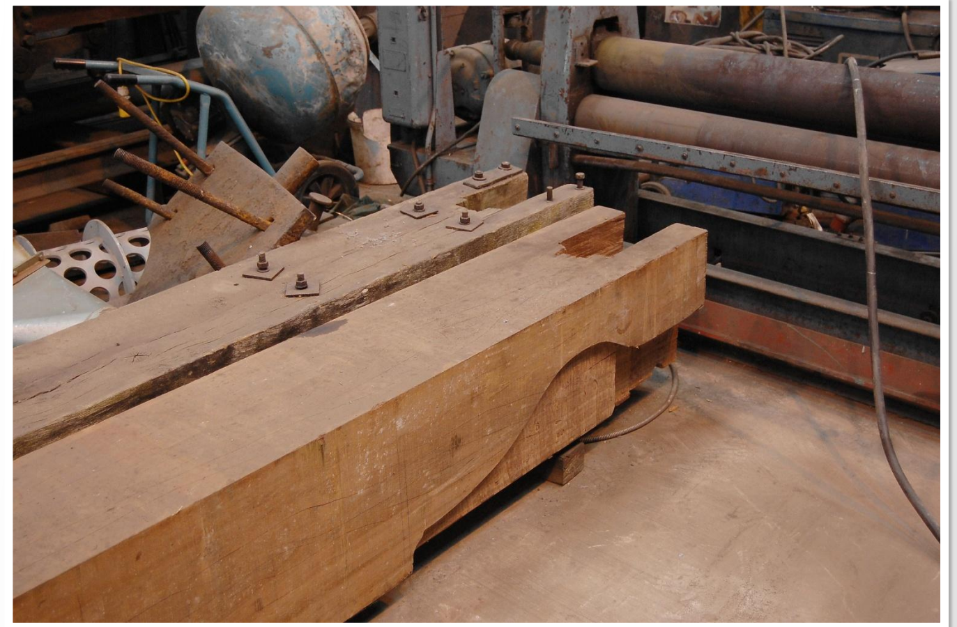
Fig 37 03/09/2010 Replacement Rocker Beams machined to accept Connection Rod bearing metalwork to original details.
