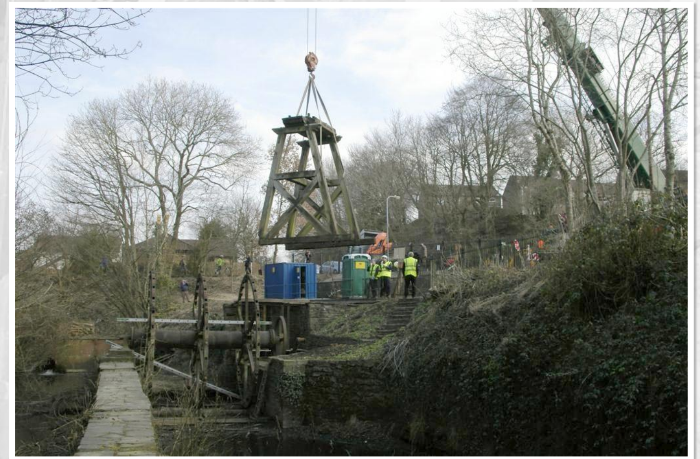
Fig 8 11/03/2010 A-frame being lifted out in one piece.
