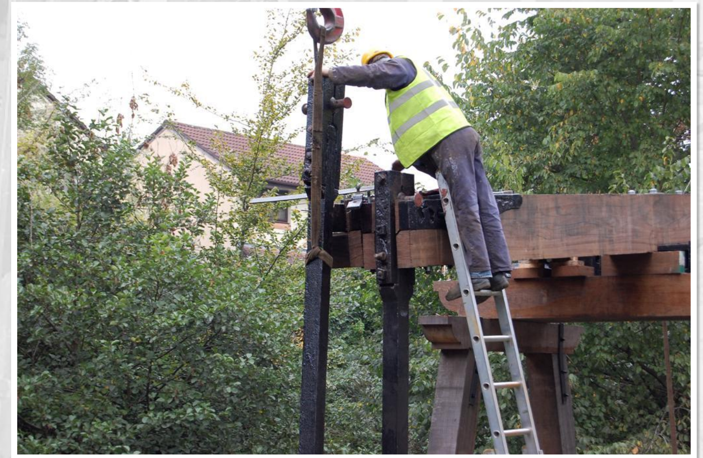
Fig 57 14/10/2010 Connection Rods lowered into position within bearing housings.
