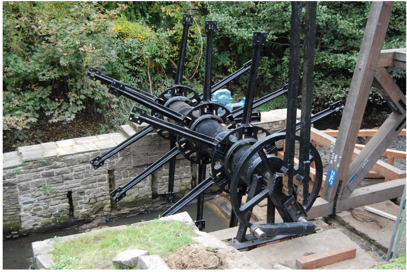
Fig 58 15/10/2010 Wheel spokes being attached to the axle and hubs.
