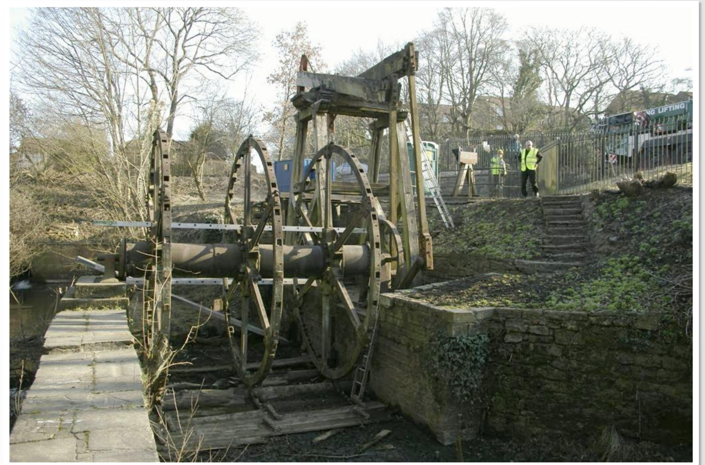
Fig 6 11/03/2010 View of Wheel and Pump from Island wall.
