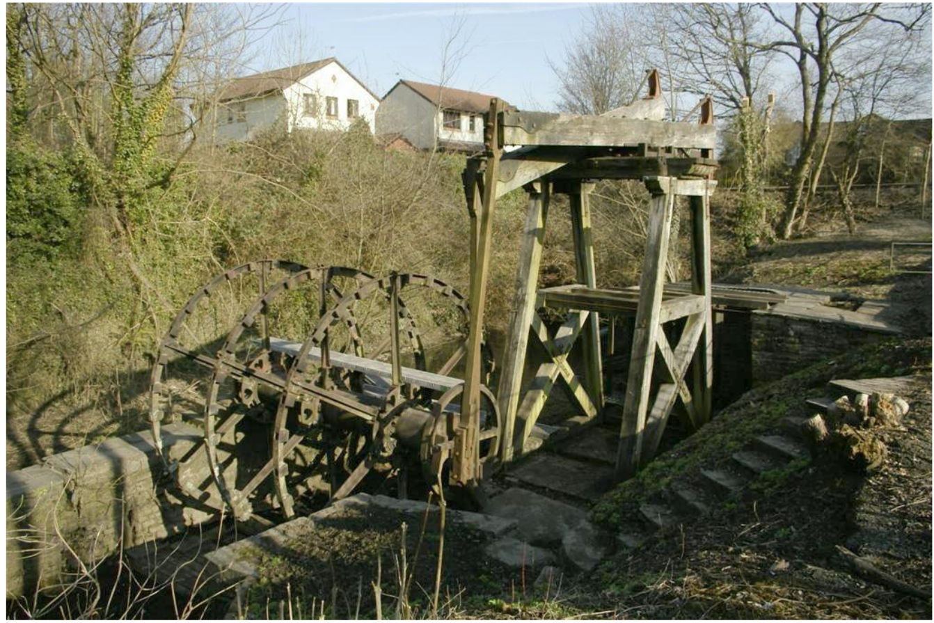
Fig 5 11/03/2010 View of Wheel (and Pump) with paddles blades removed, ready for lifting out.
