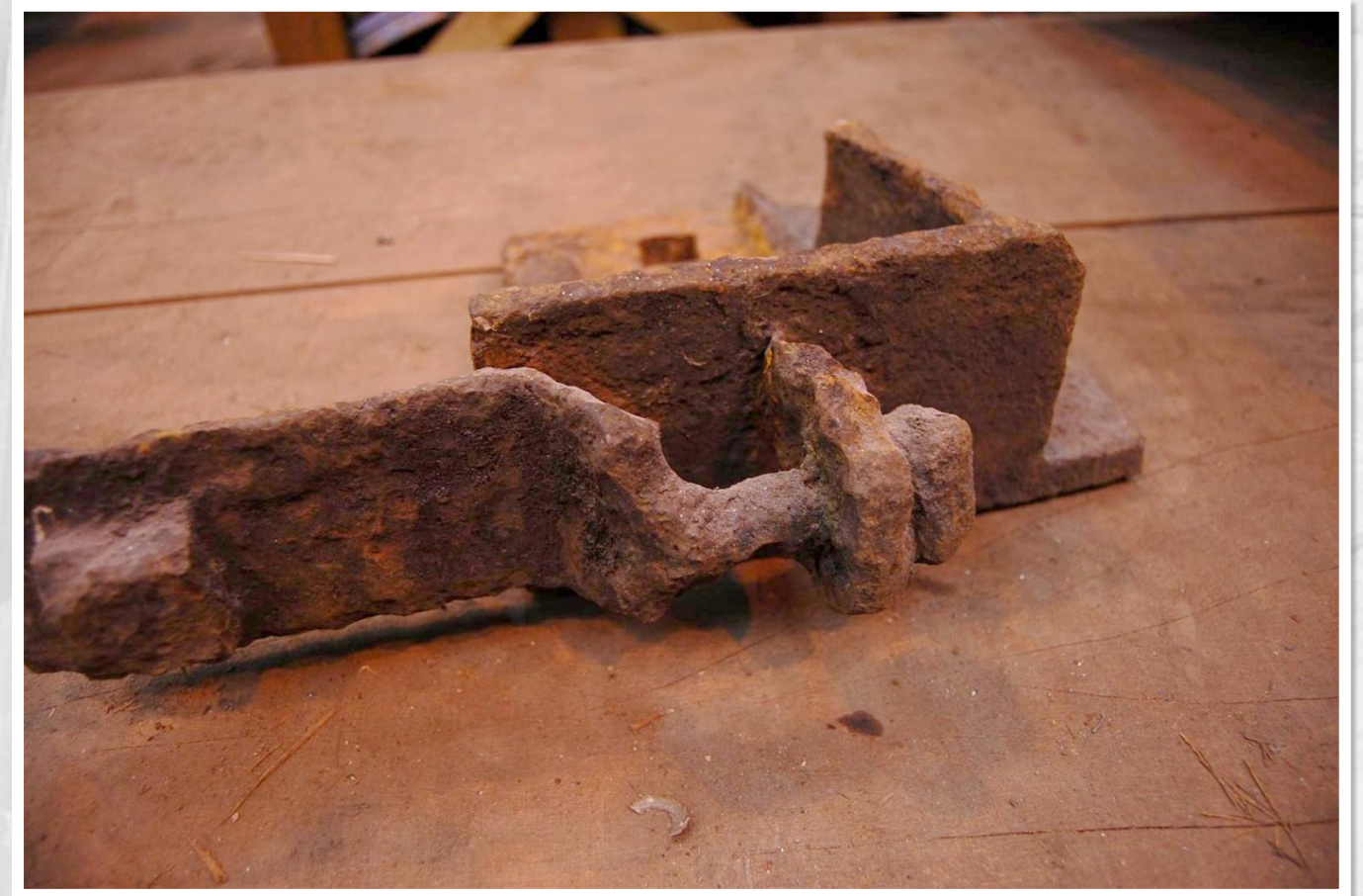
Fig 25 11/05/2010 Remains of Wheel Rim segment with original segment tie. Ties exhibit loss of section and heavy corrosion. Note part remains of original square-head bolt. All Ties subsequently replaced with new to match original details.
