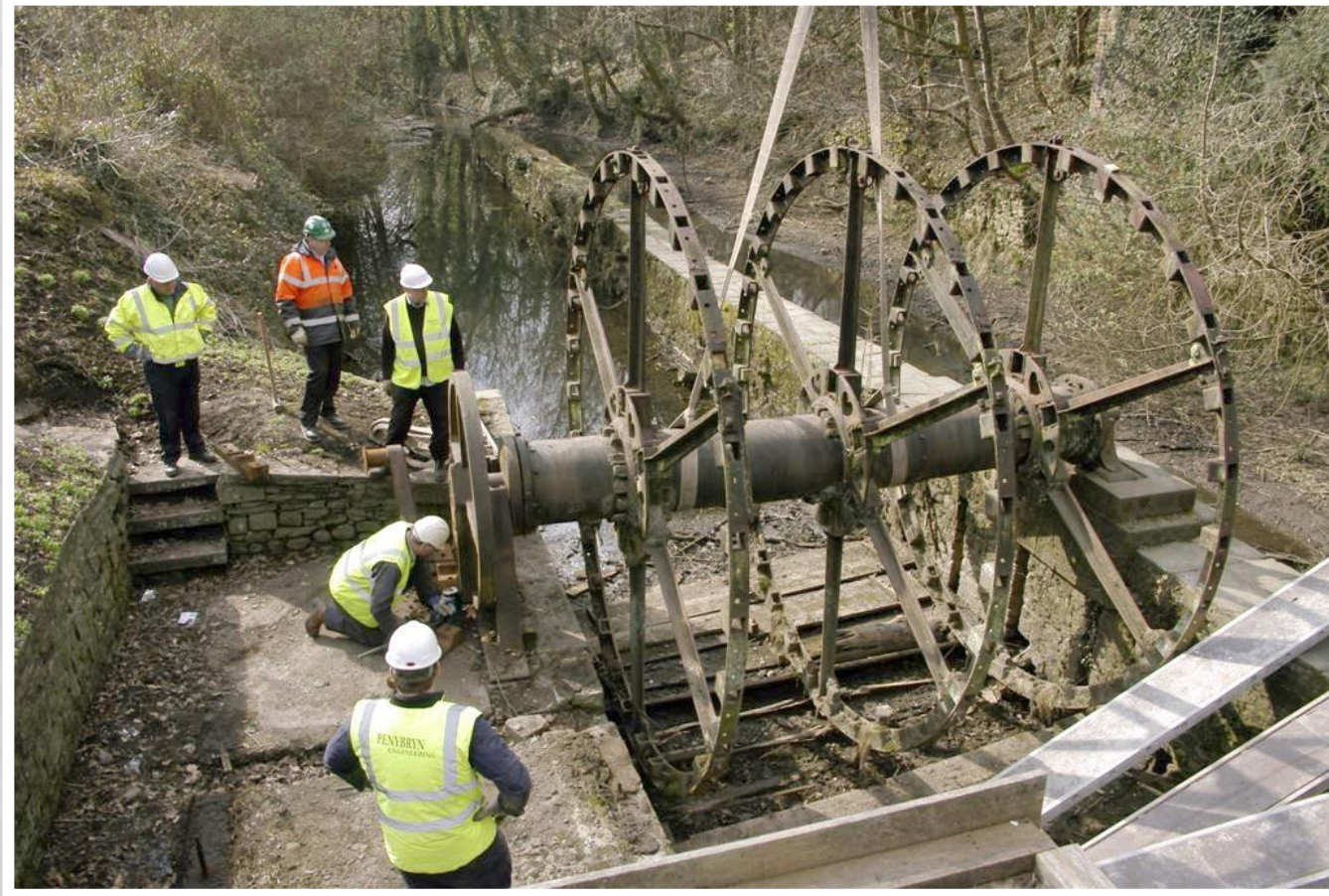
Fig 11 11/03/2010 Wheel and axle being prepared for lifting off its bearings.
