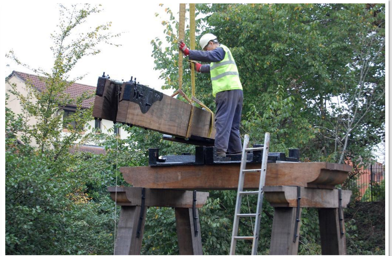
Fig 55 Far-side Rocker Beam lowered in position on bearing saddle.
