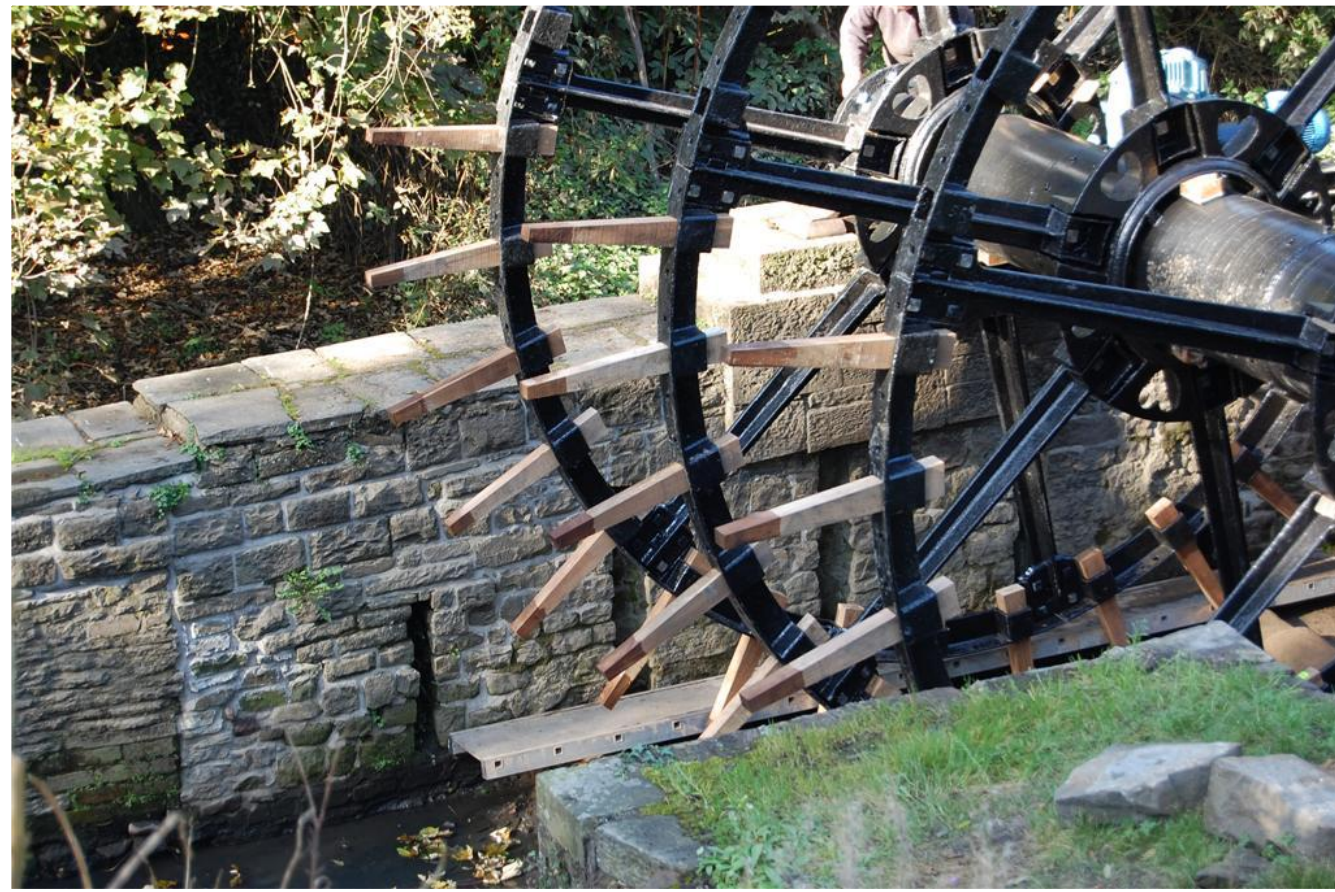
Fig 60 21/10/2010 Elm Blade Brackets being attached to the Wheel Rims.
