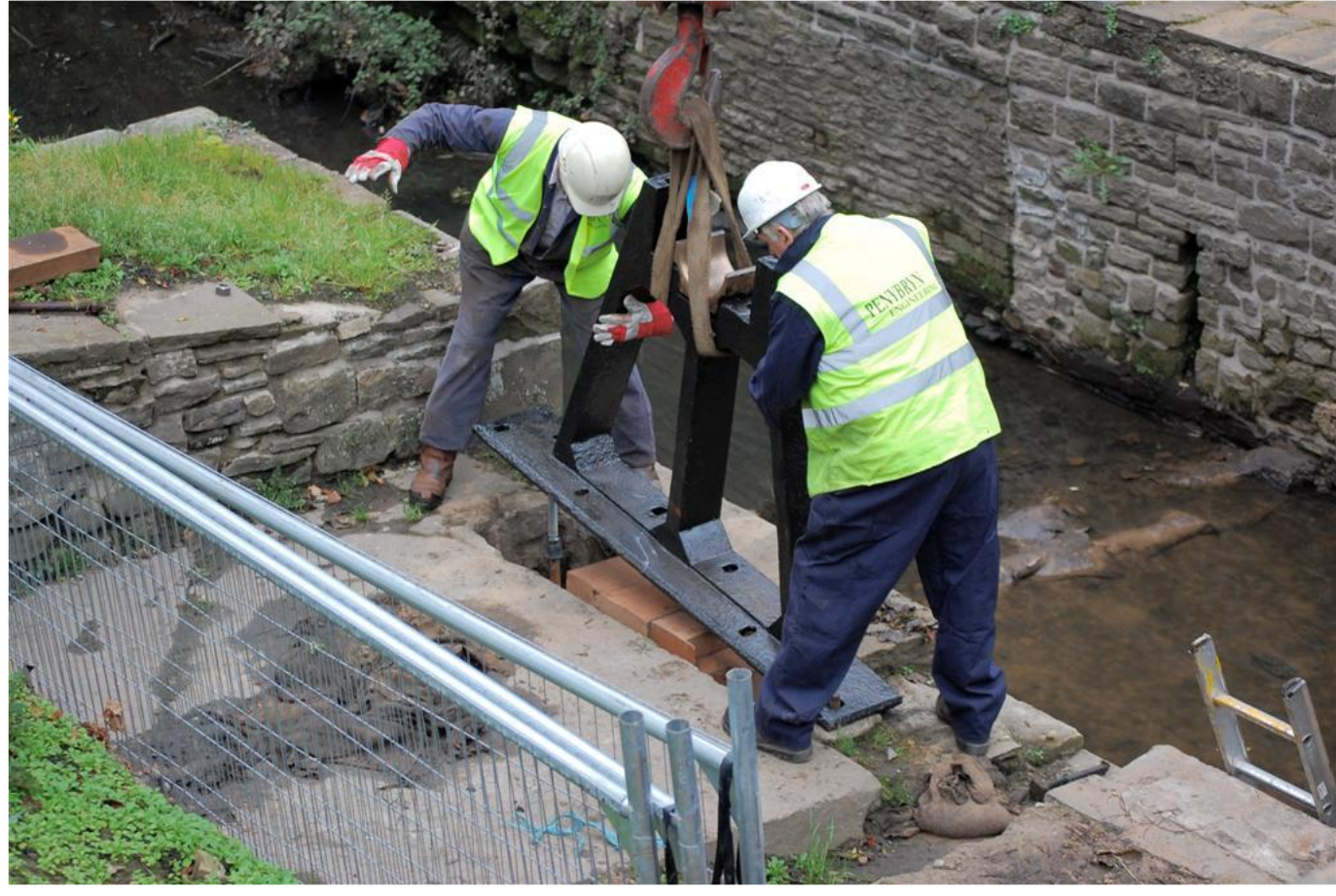
Fig 46 14/10/2010 Near-side bearing pedestal lowered into position. Note new bronze bearings.
