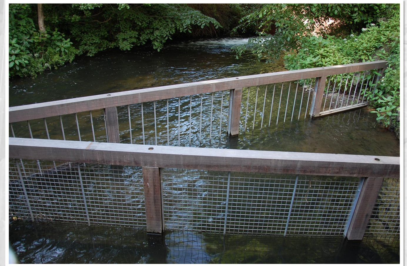
Fig 65 02/06/2011 Completed Filter Screens in position across Head-race.
