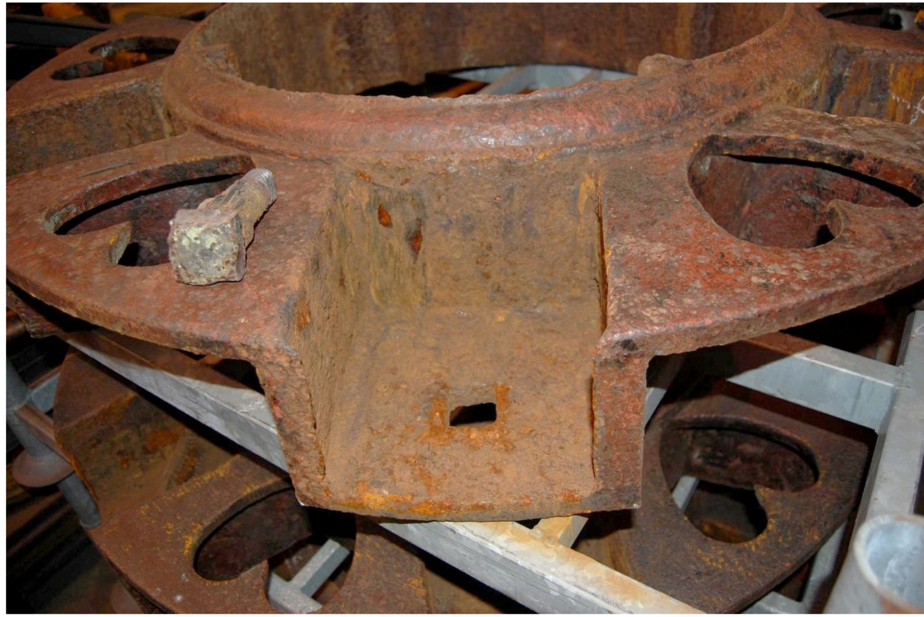
Fig 26 11/05/2010 Typical Wheel Hub. Found to be in good condition requiring cleaning by hand to remove loose metal and rust.
