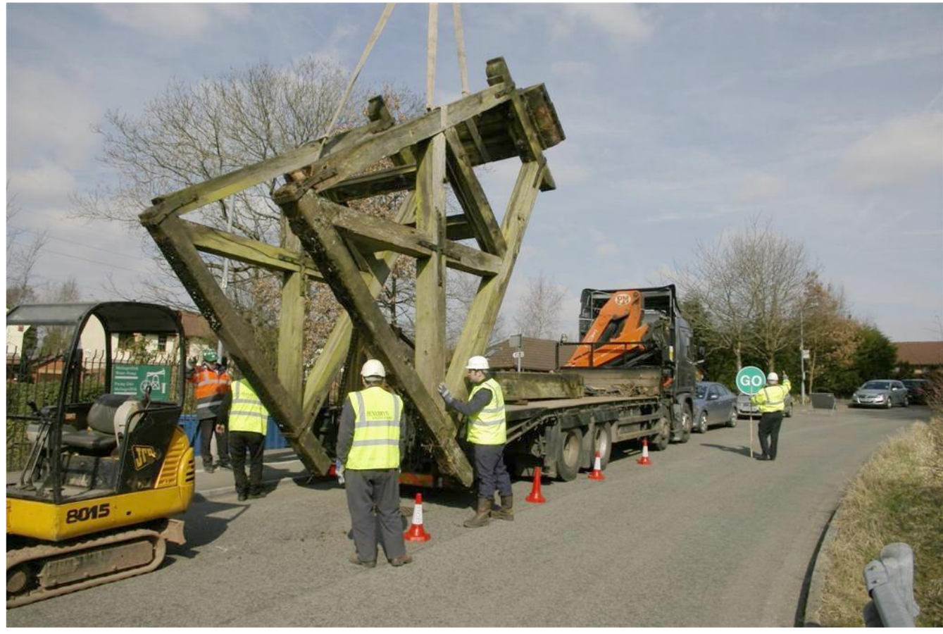
Fig 9 11/03/2010 A-frame being loaded onto transport. Rocker Beams already loaded.
