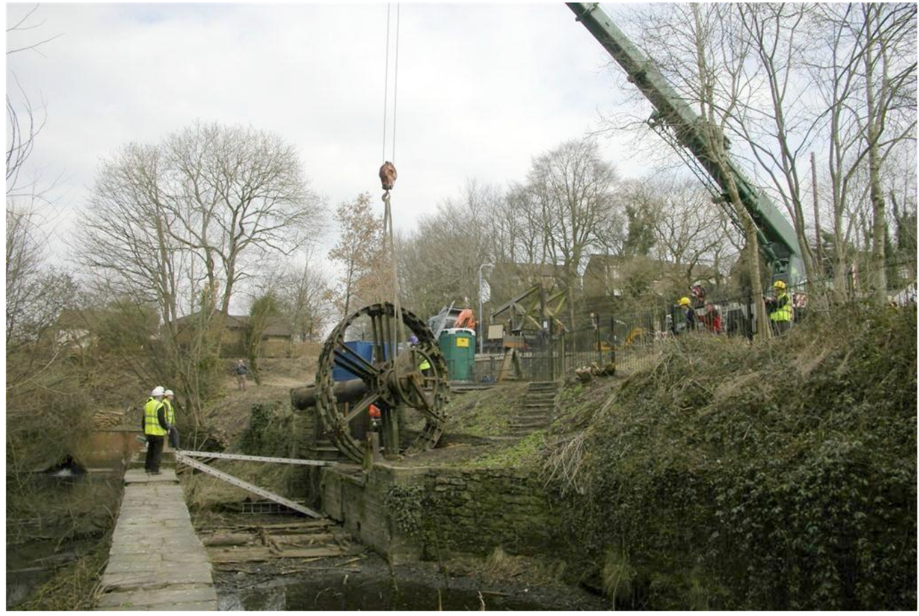
Fig 13 11/03/2010 Wheel rims, axle and crank arms lifted away in one piece.
