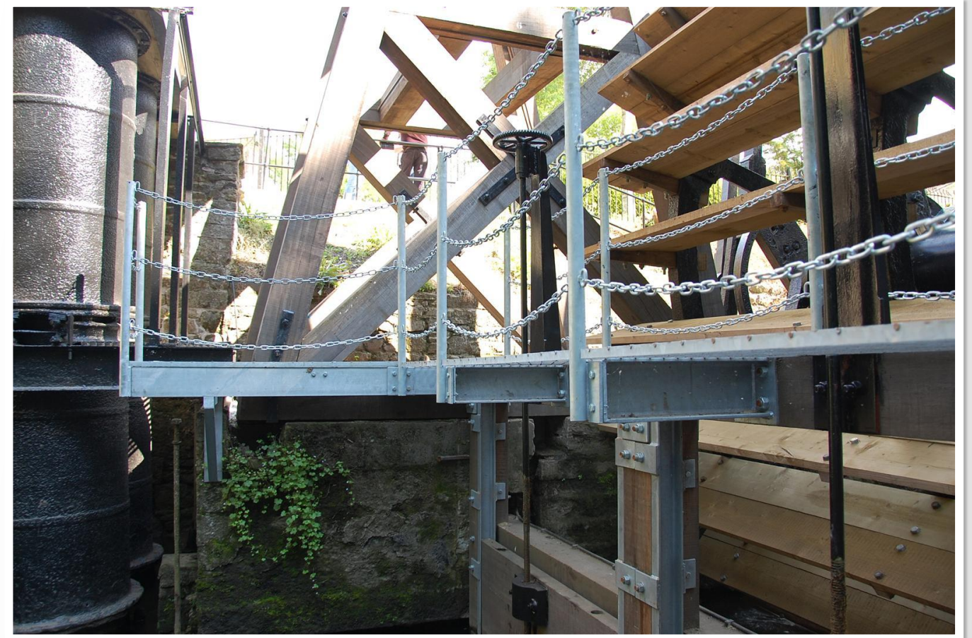
Fig 67 02/06/2011 Walkway support steelwork fixed to Sluice Gate frame and masonry wall.
