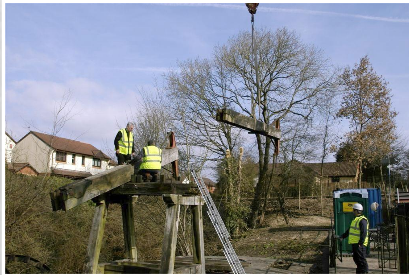
Fig 7 11/03/2010 Rocker Beam being lifted away, the other being prepared for lifting.
