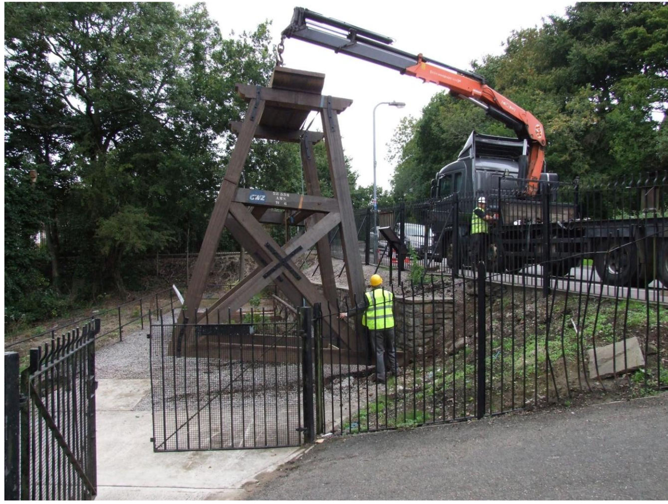
Fig 42 15/09/2010 Replacement A-frame lowered to temporary location in advance of main lift.
