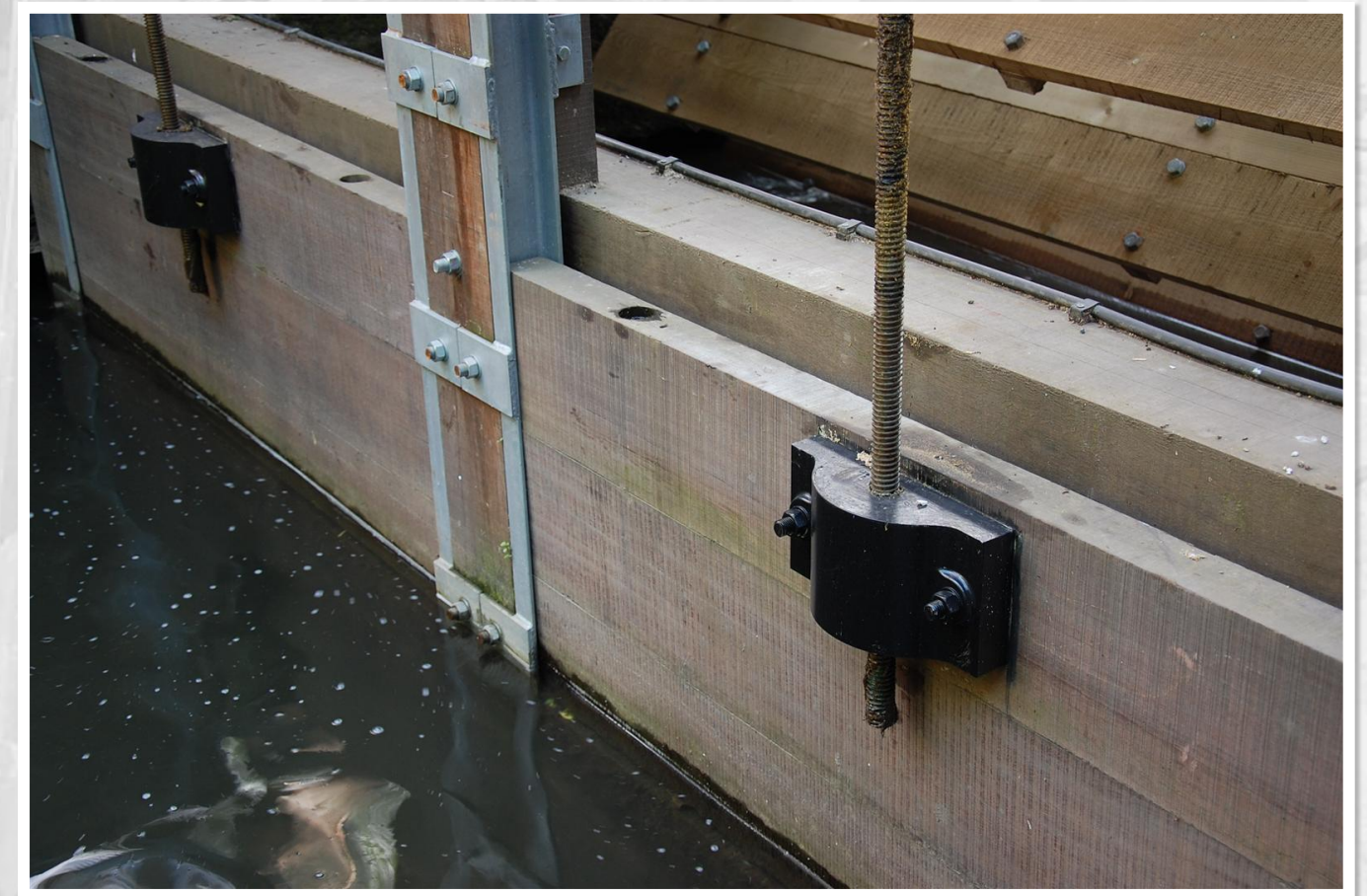
Fig 69 02/06/2011 View showing lifting Sluice Gate mechanism details below access walkway.
