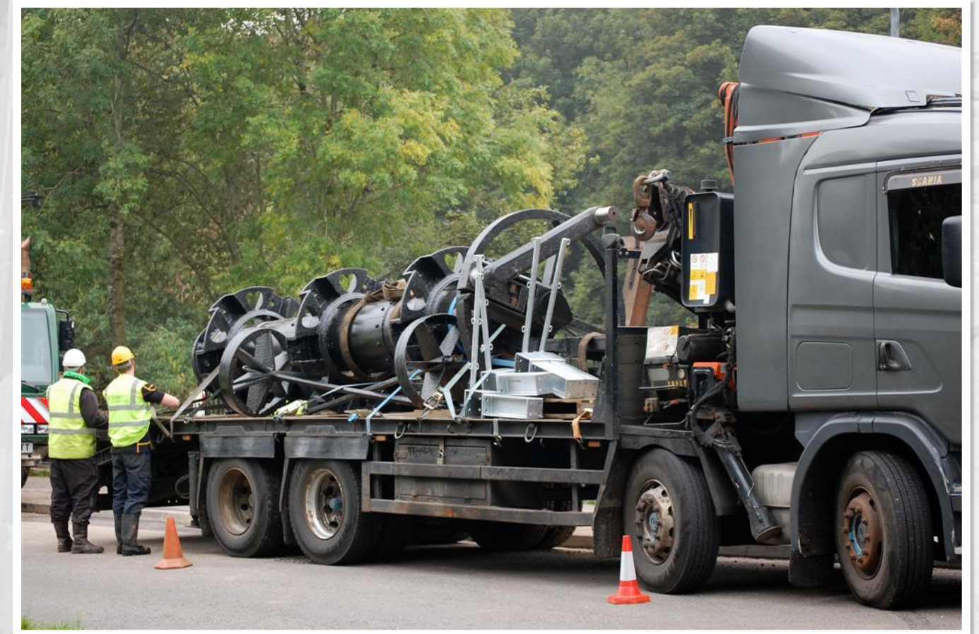
Fig 45 14/10/2010 Wheel components delivered to site to be lifted into position.
