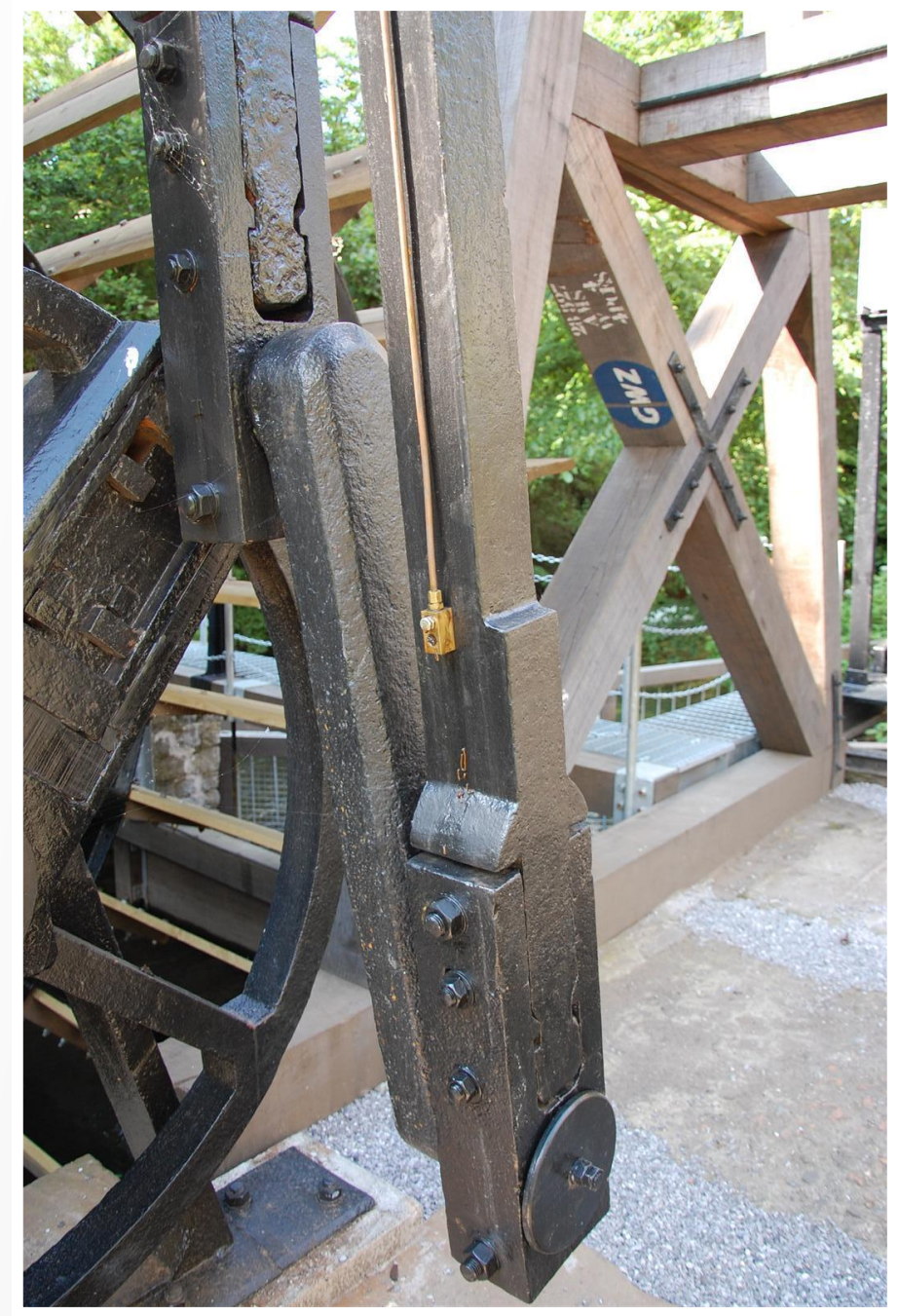
Fig 63 02/06/2011 Lubrication access point to upper Connection Rod bearings. Lower bearing lubrication point on reverse face.
