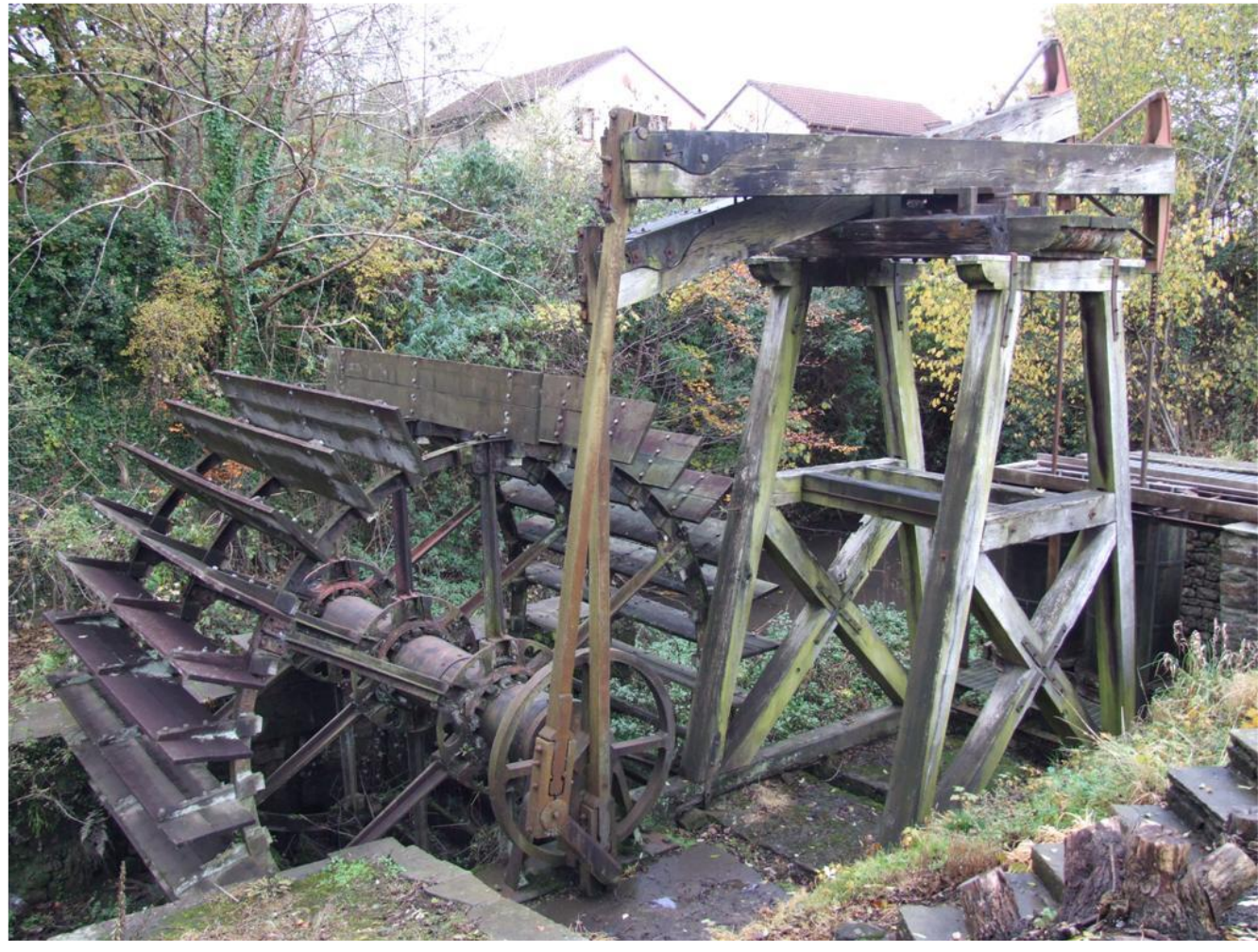
Fig 1 04/09/2008 View of the Wheel and Water Pump showing general dilapidated state of repair.
