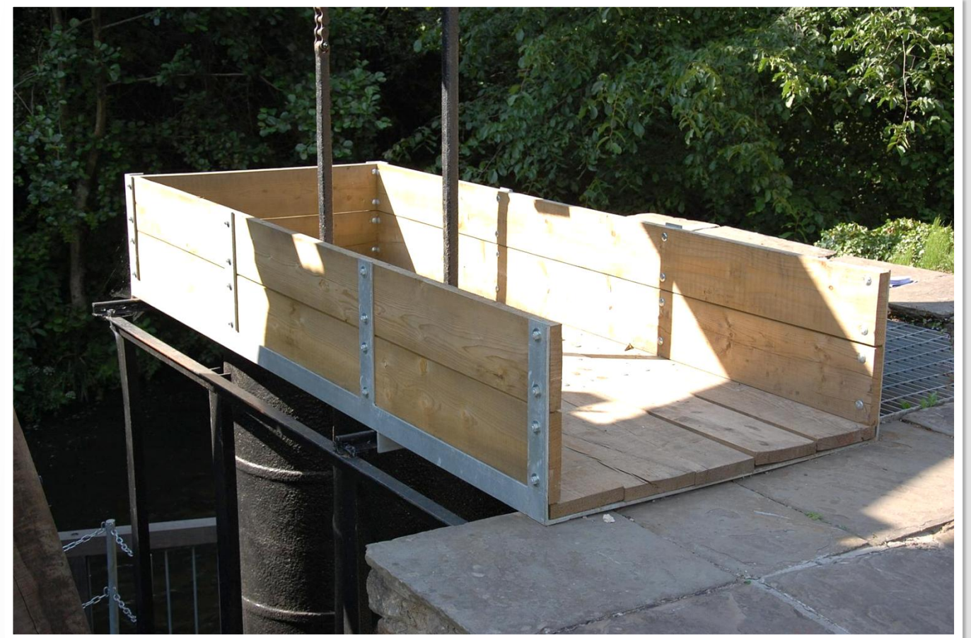
Fig 71 02/06/2011 View of the replacement timber Launder.
