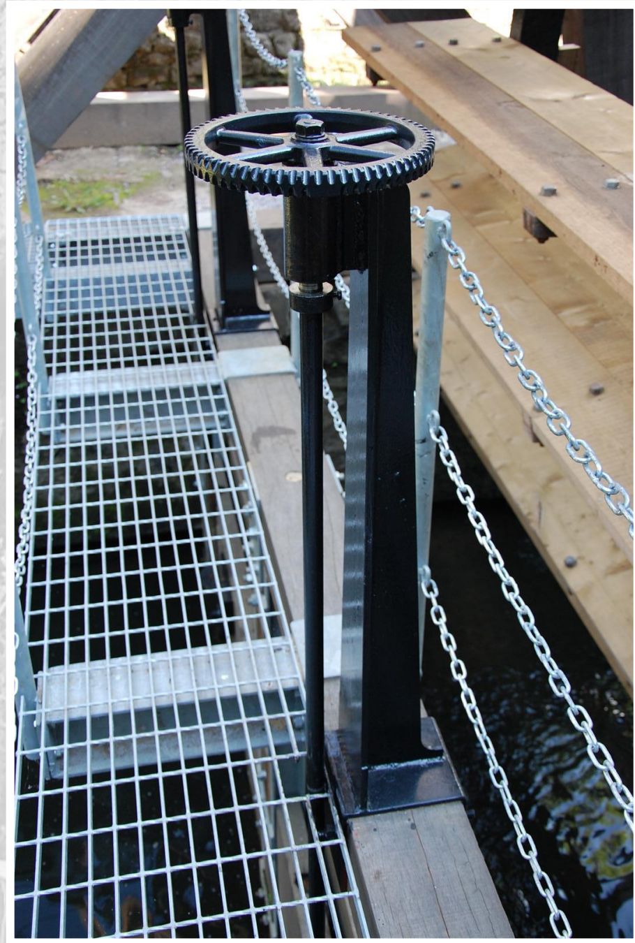
Fig 68 02/06/2011 Detail of lifting mechanism and pedestal.
