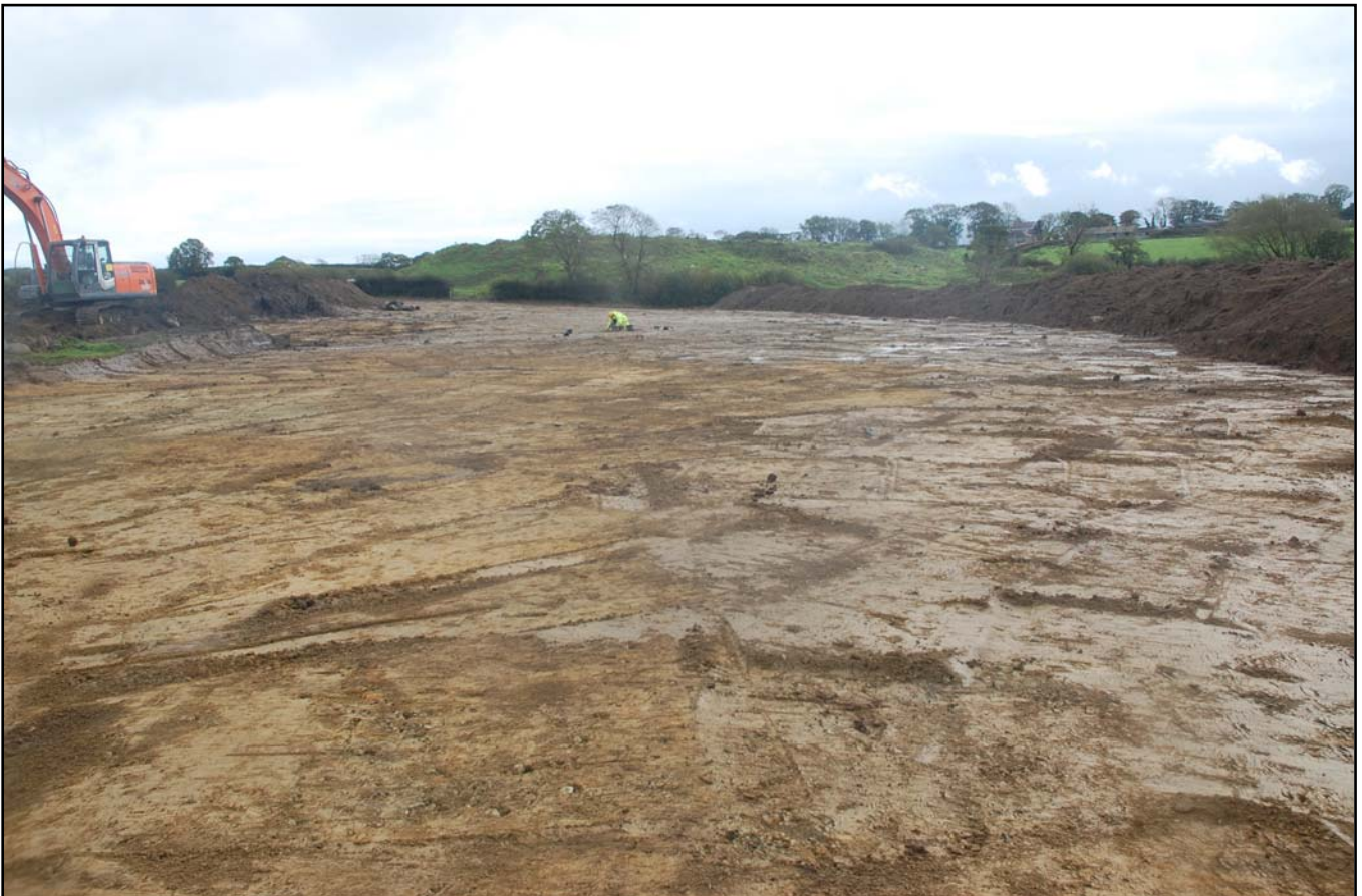
Plate 02: Stripped 1.6ha area. Photograph taken from the west.
