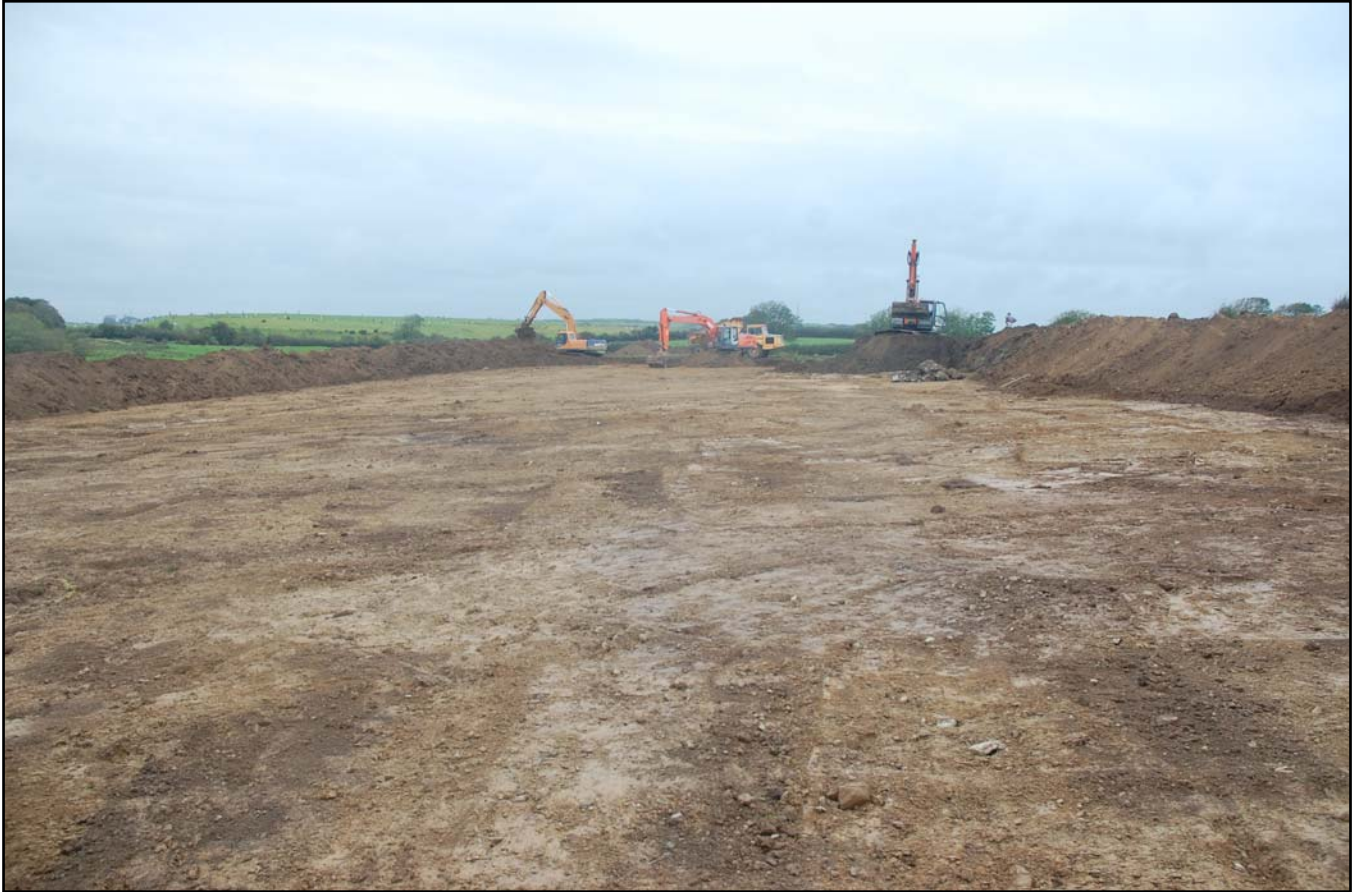
Plate 01: Stripped 1.6ha area. Photograph taken from the east.
