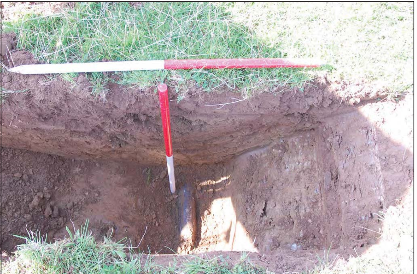
Plate 12 - Excavated section of TH15, water mains at base of trench.
