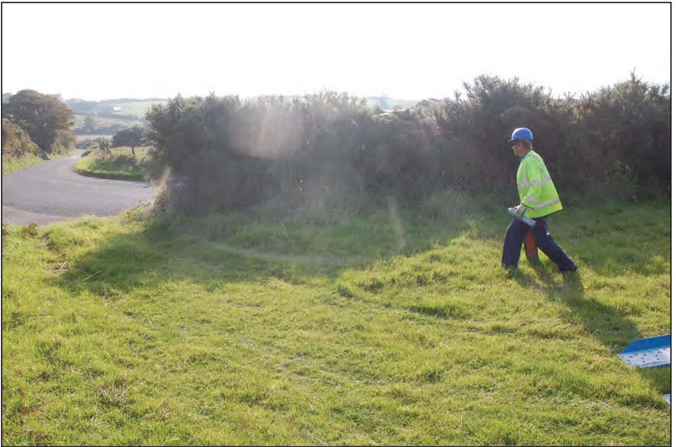
Plate 09 - Location of TH14 at the entrance to Cae'r Eglwys Farm at the left hand side of the road..
