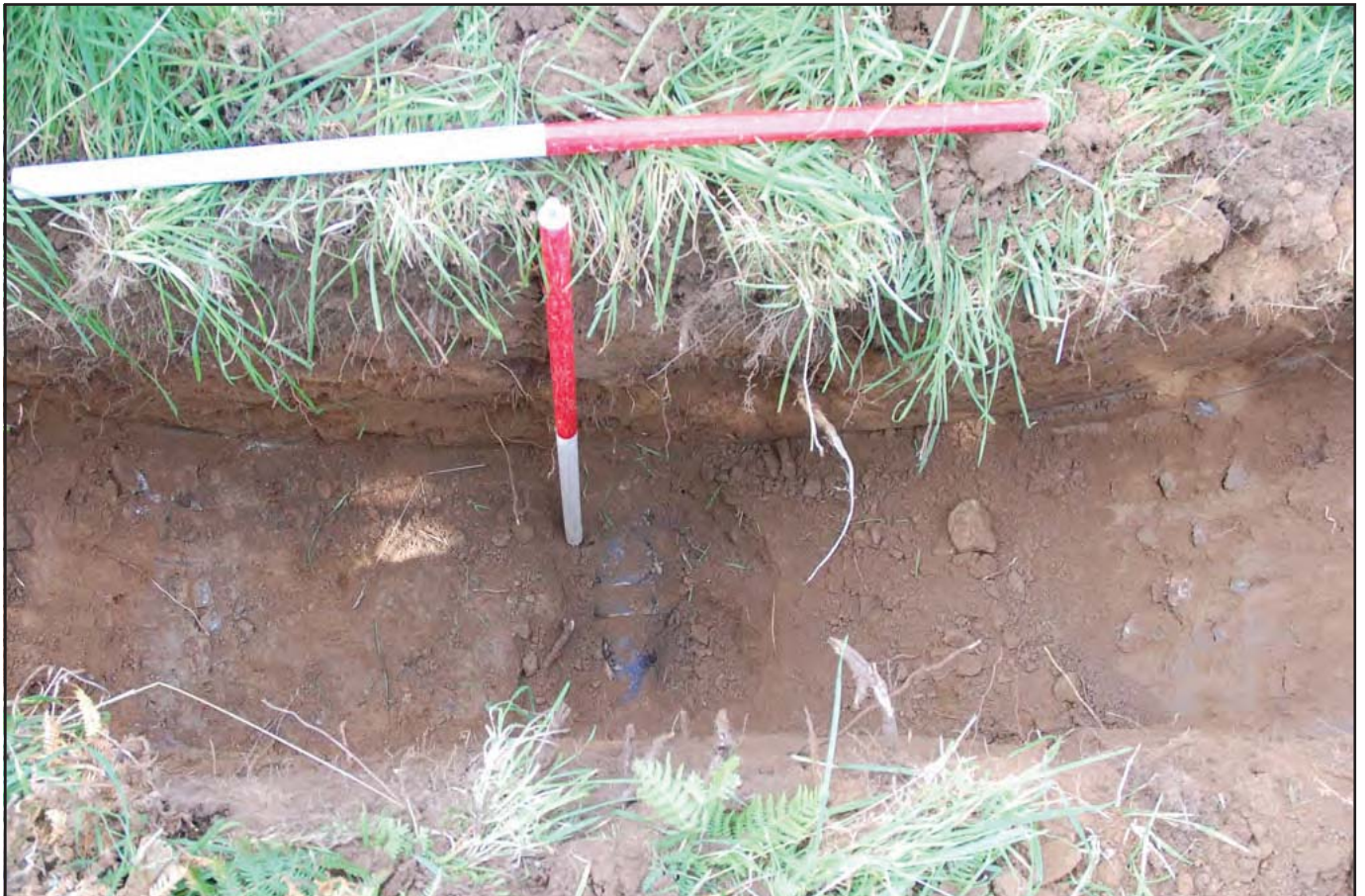
Plate 06 - Excavated section of TH11 with exposed water main.
