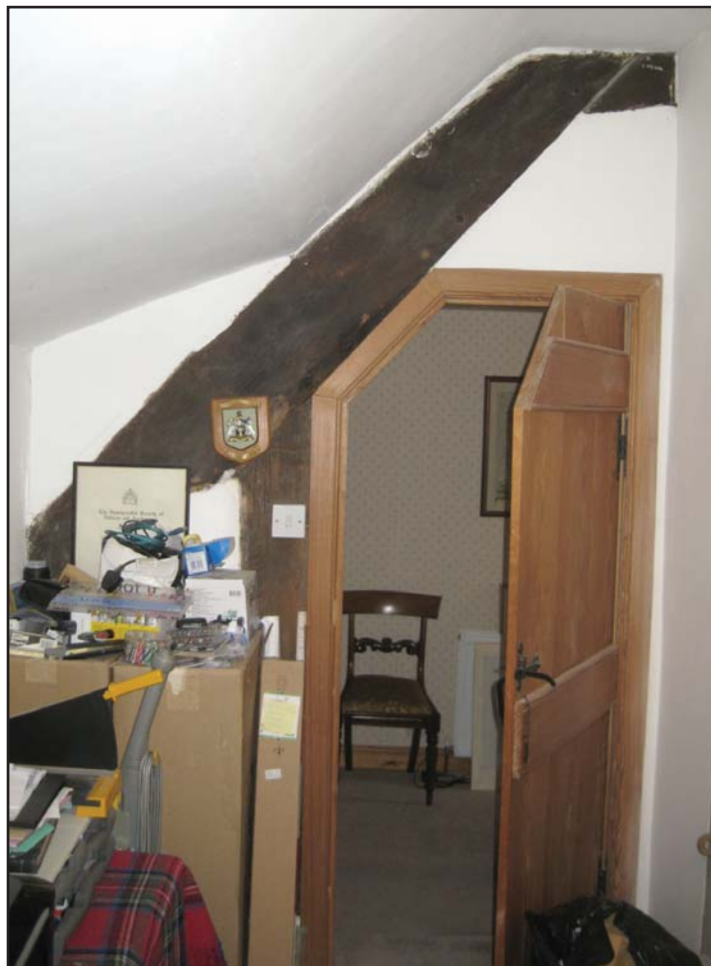
Plate 08: The western side of the southern face of the central cruck which forms the south side of the screens passage
