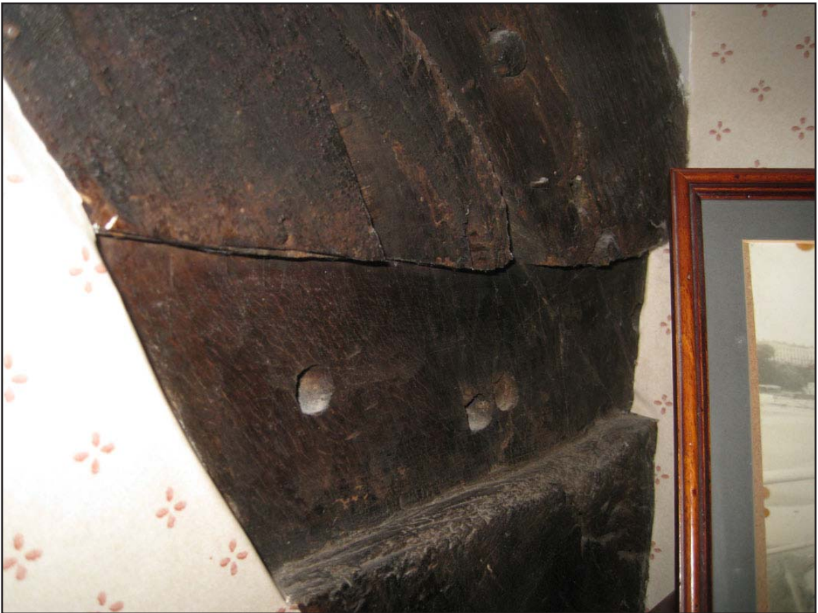
Plate 12: Close up of the housing for a tie beam on the eastern side of the southern face of the northern cruck, which forms the southside of the screens passage; view from the south.
