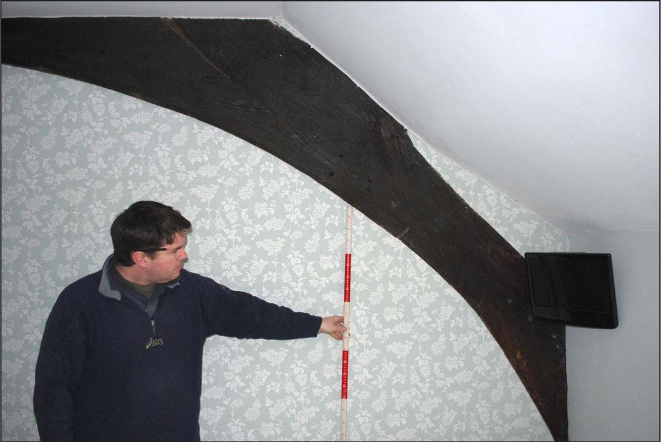
Plate 3: The eastern side of the southern face of the southern cruck which divides the hall; view from the south.
