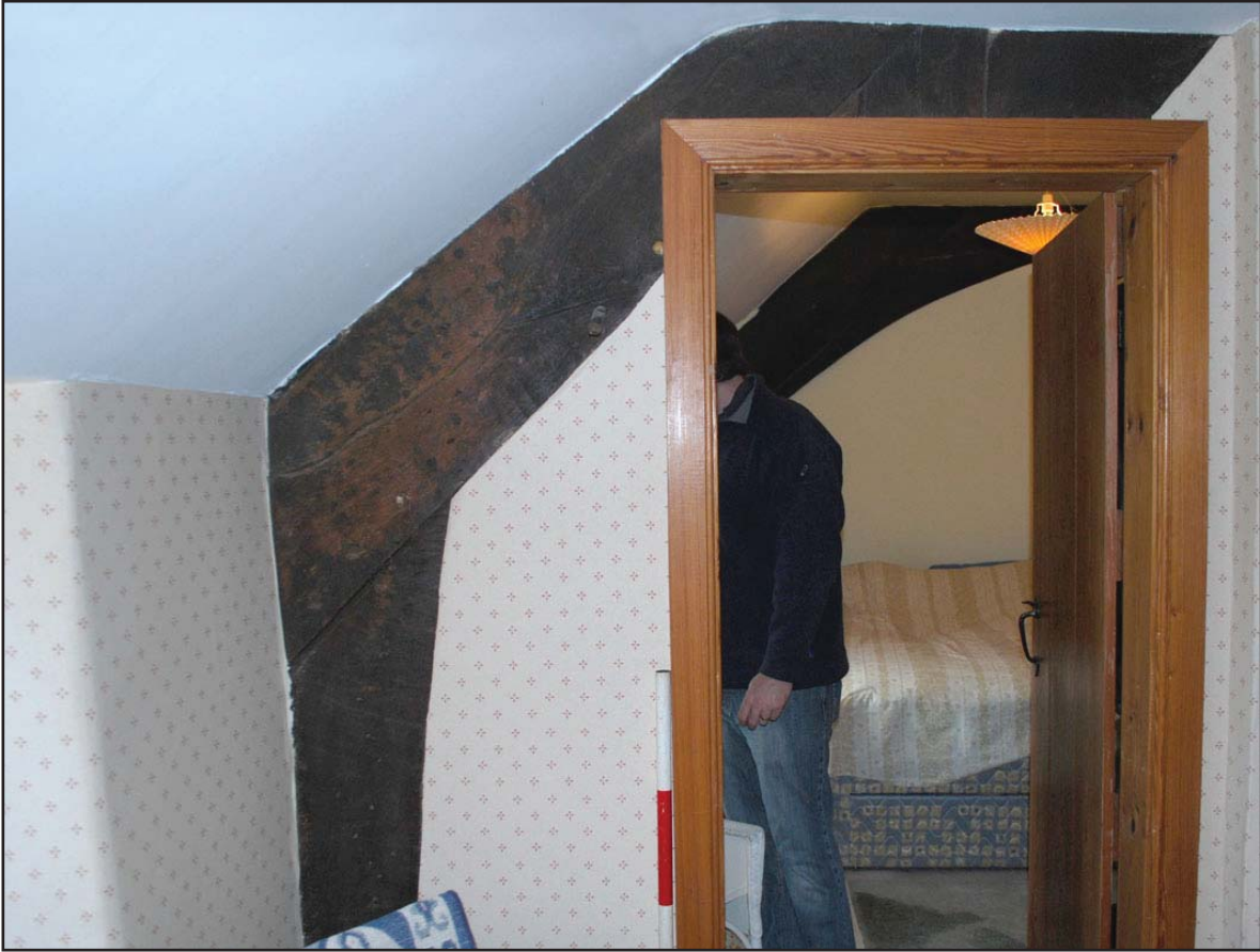
Plate 9: The eastern side of the northern face of the central cruck which forms the southside of the screens passage; view from the north.
