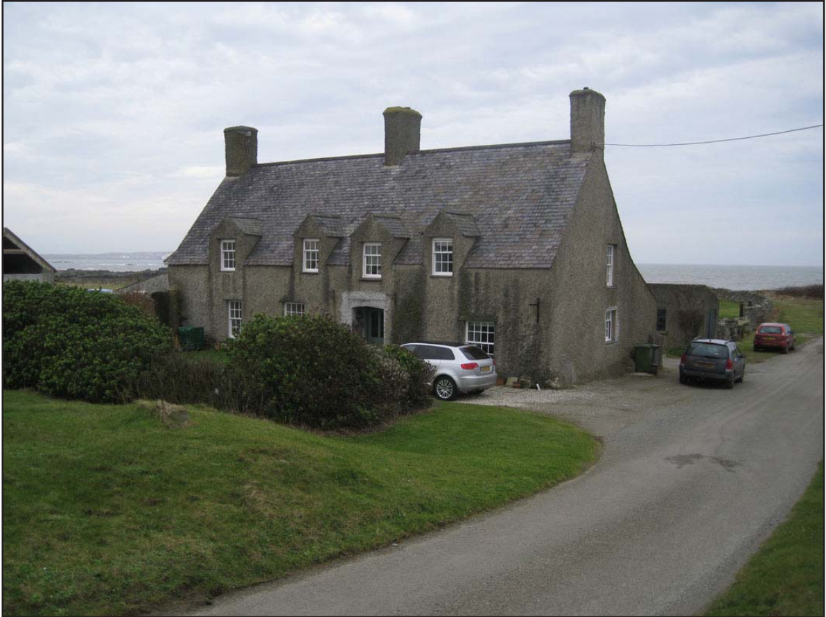
Plate 01: The eastern elevation of Trefadog; view from the northeast.
