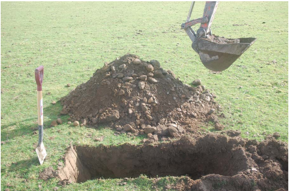
Plate 2 Test Pit 11 under excavation
