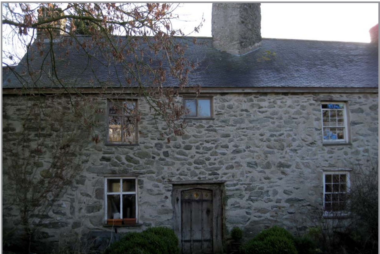
Plate 2: Gronant west facing elevation of building A, showing doorway which leads into the west passage, which retains its original frame supporting a Tudor arched lintel
