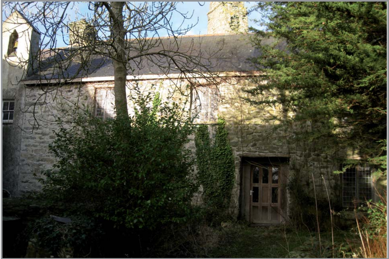
Plate 11: Gronant east facing elevation of building A
