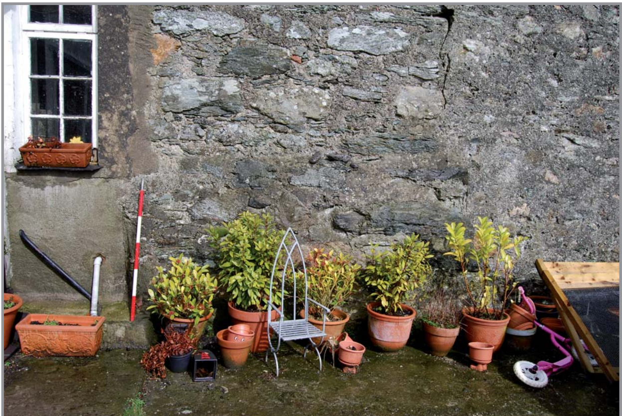
Plate 6: Gronant south facing elevation of building B, showing possible original foundations
