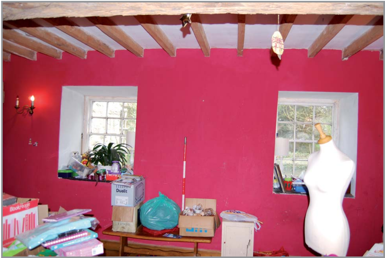
Plate 15: Gronant building B living room facing south showing two 12 pane sash windows
