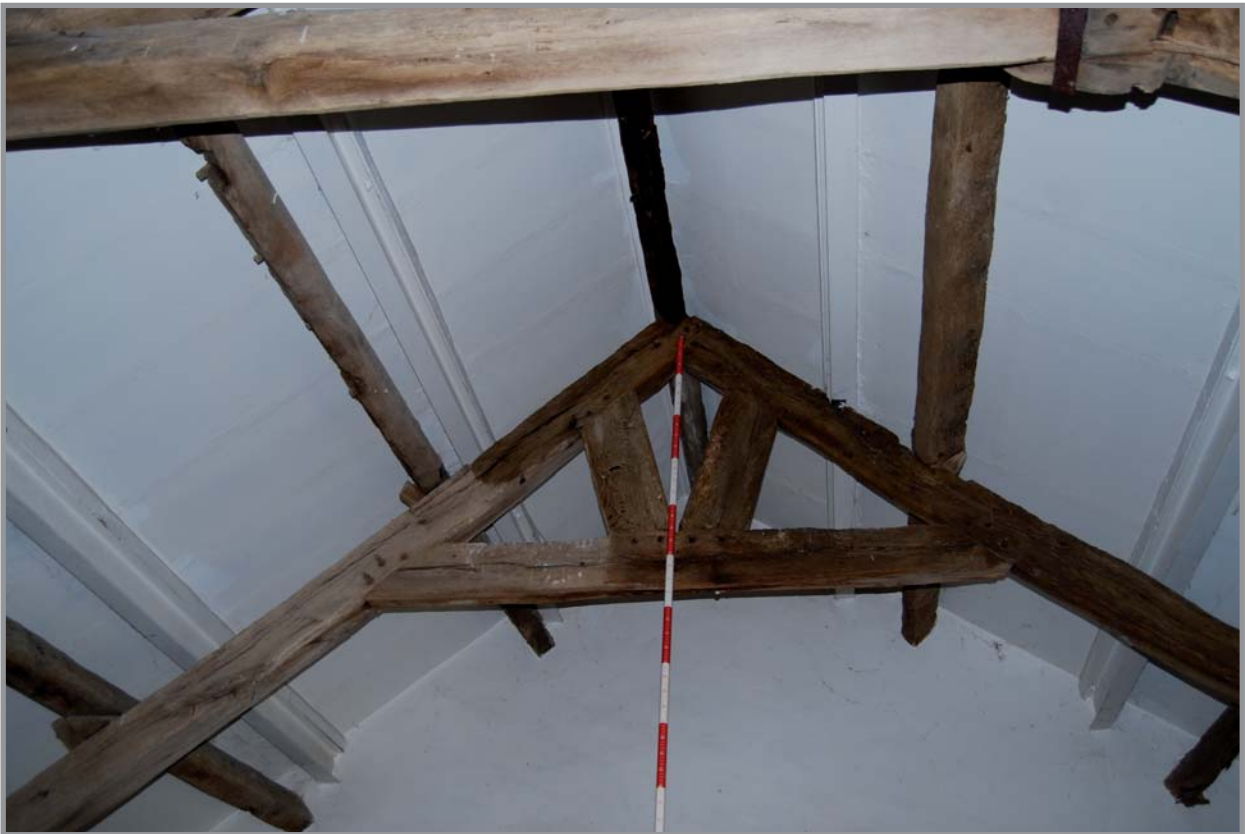
Plate 28: Gronant building A, first floor. Truss 2 facing north
