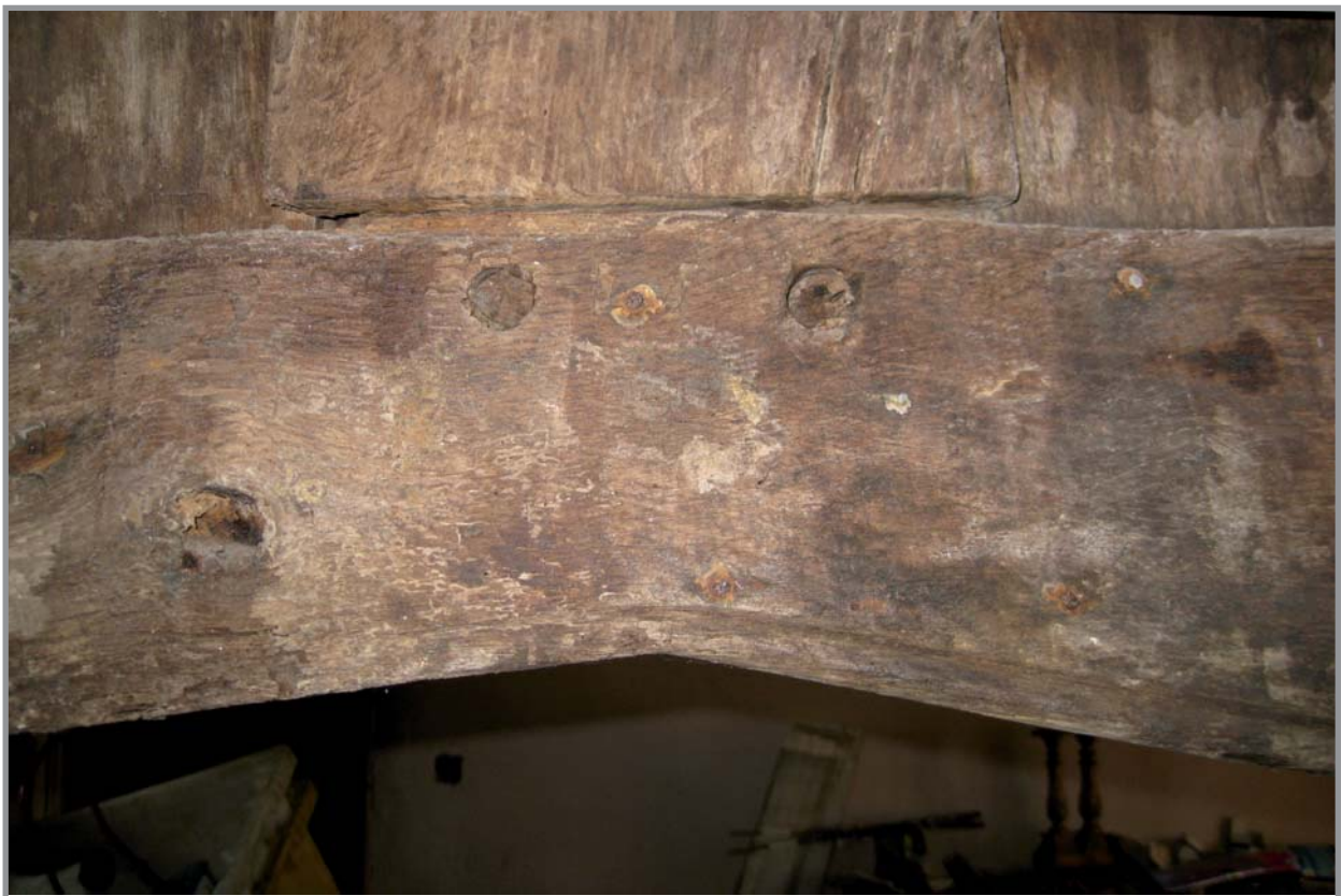
Plate 20: Gronant building A. Post and panel screen, detail
