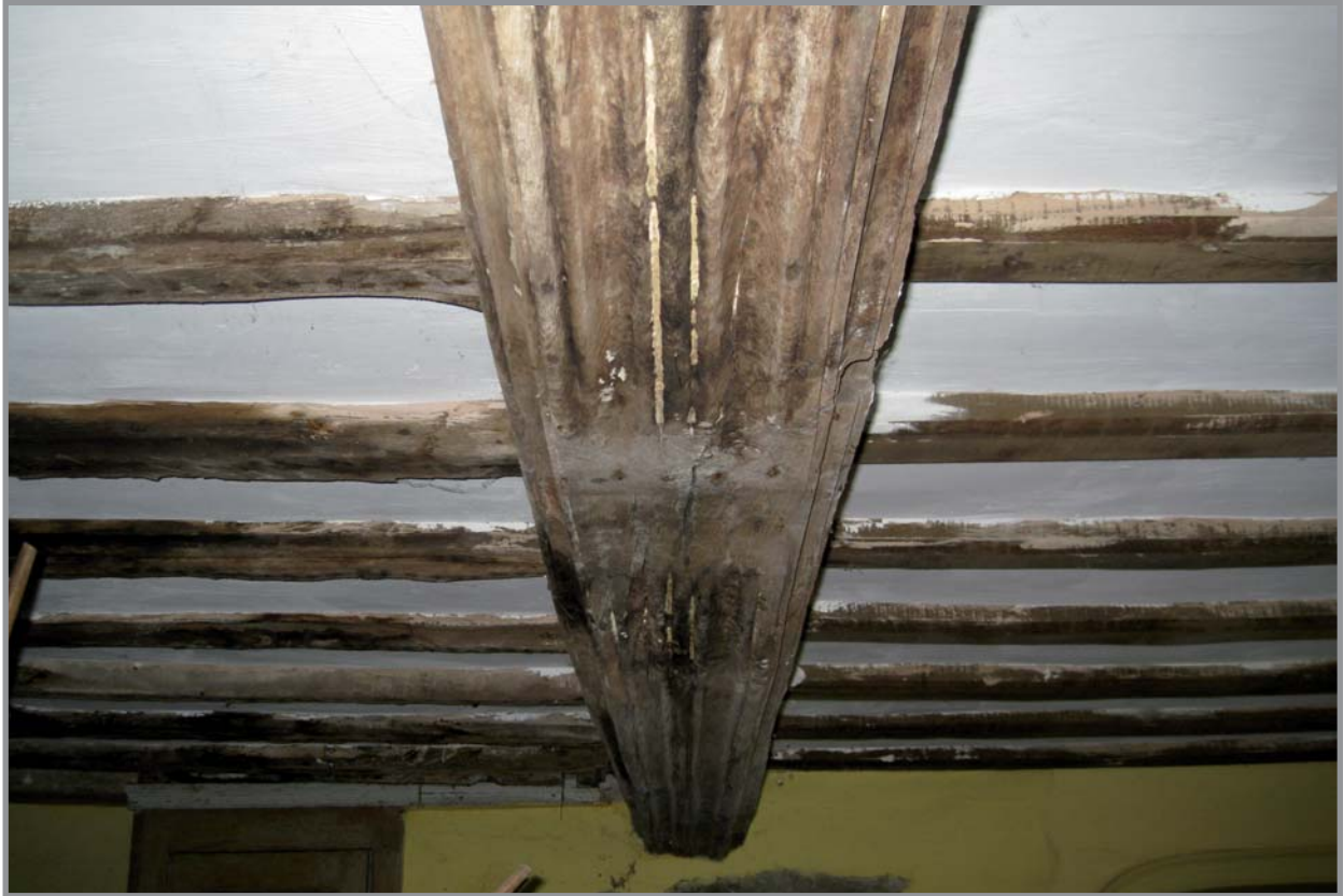
Plate 23: Gronant building A. Heavily moulded beam
