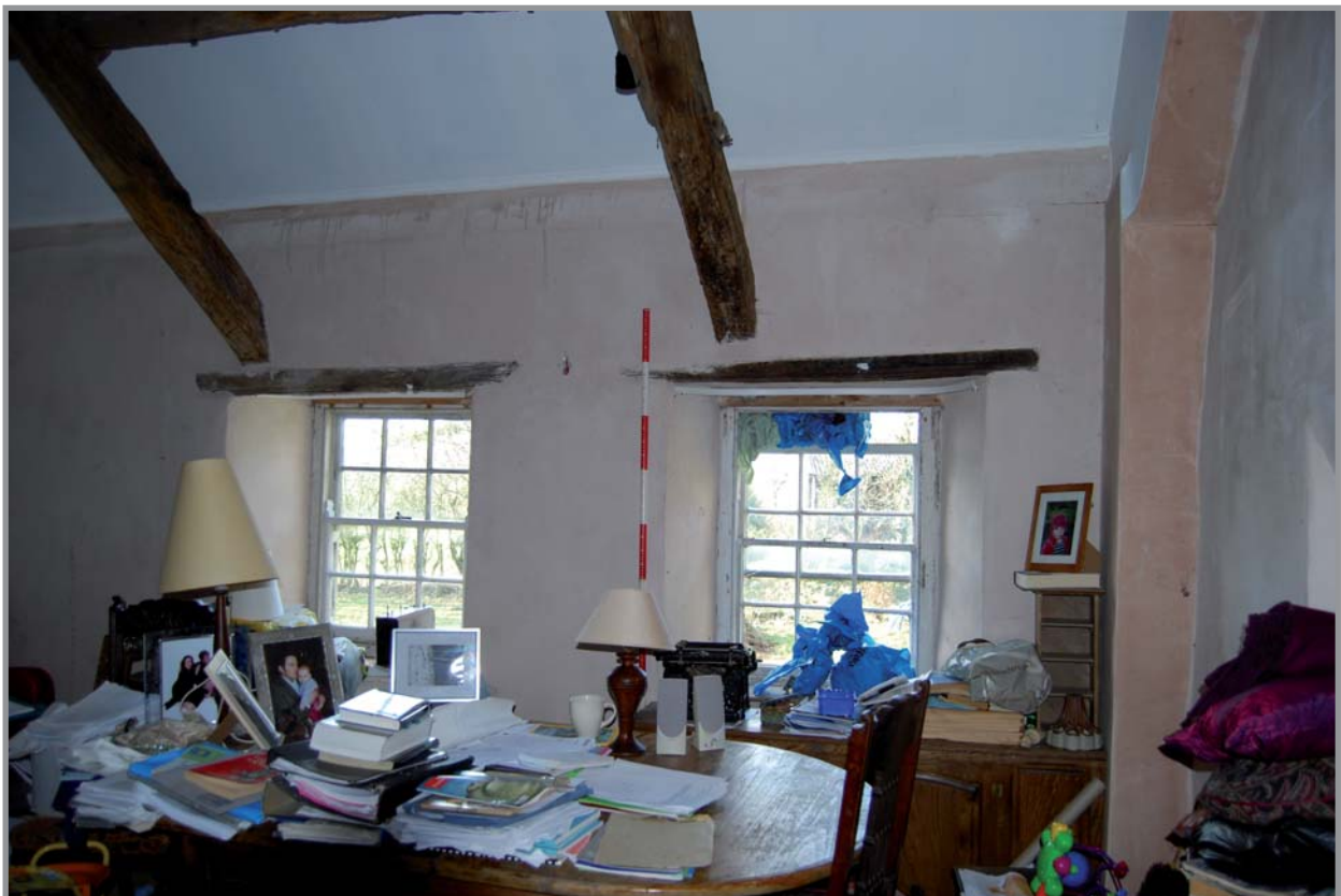
Plate 24: Gronant building A, first floor 12-pane sash windows facing east
