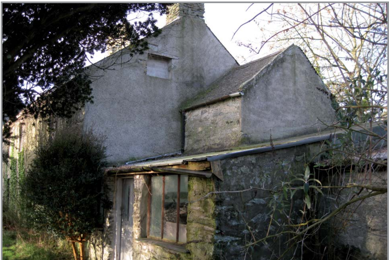
Plate 12: Gronant south-west facing image showing later extensions to building A
