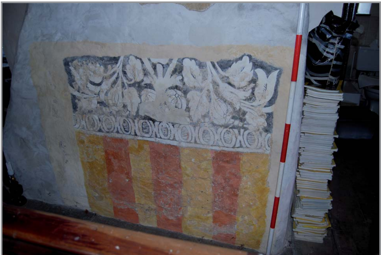
Plate 26: Gronant building A., first floor. Wall paintings discovered and restored in c. 1986. Facing west.
