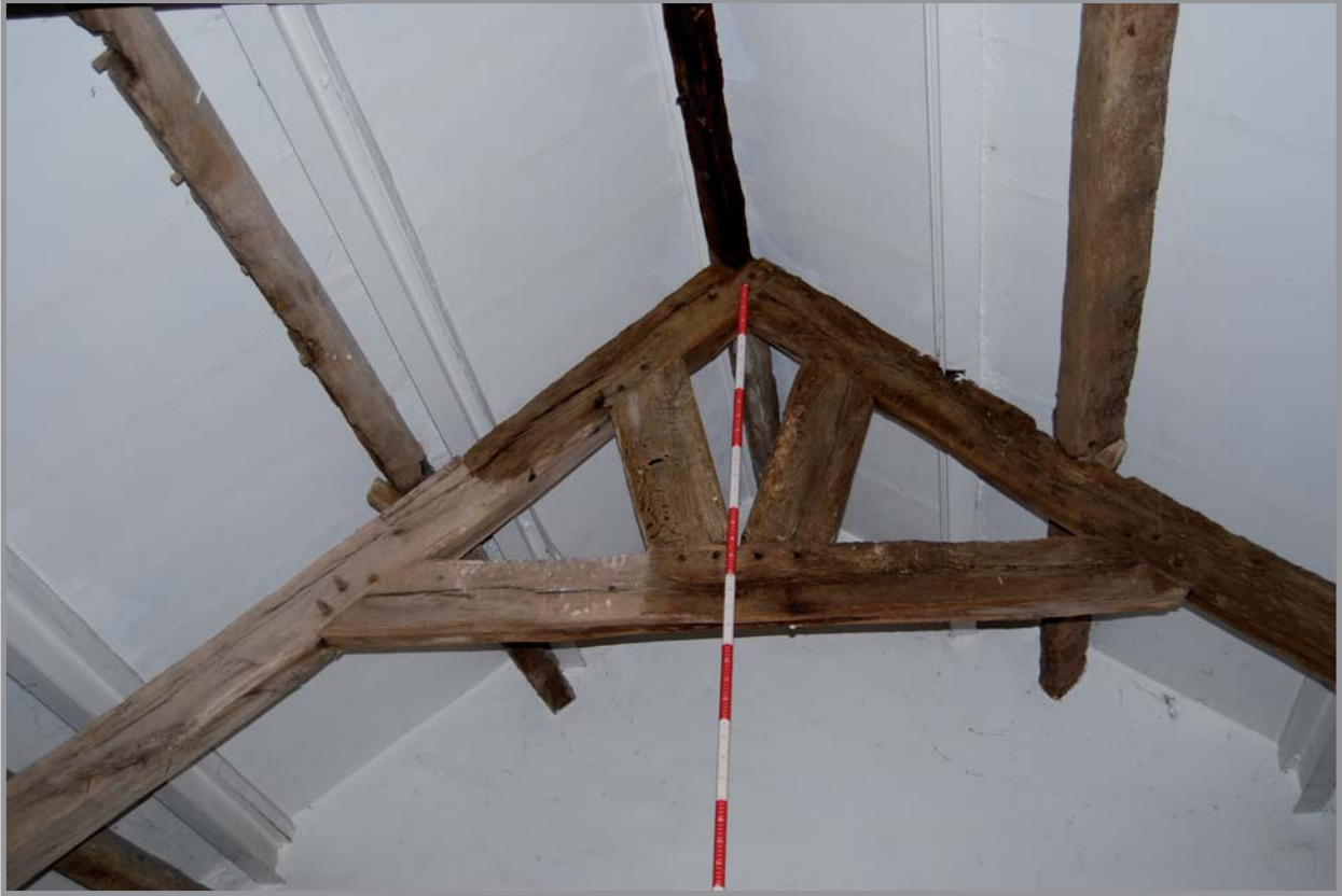
Plate 27: Gronant building A, first floor. Truss 1 facing south
