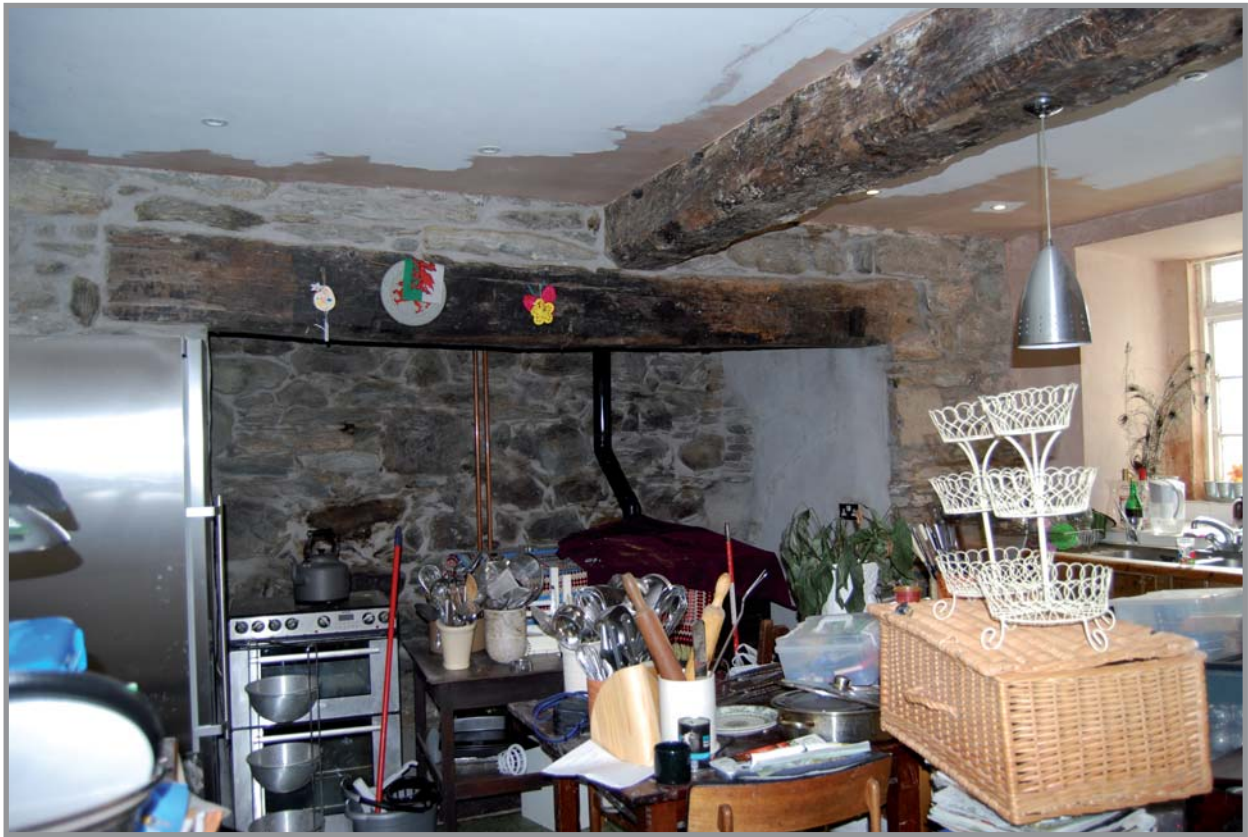
Plate 13: Gronant building B kitchen facing south west showing a large fireplace and axial beam
