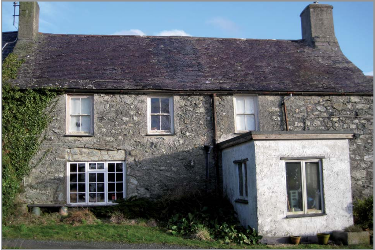
Plate 5: Gronant south facing elevation showing building B and the modern porch
