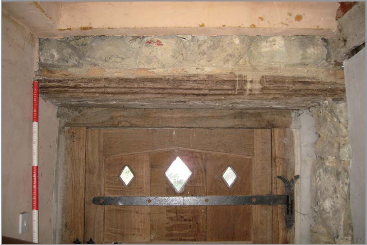
Plate 21: Gronant building A. West passage door detail facing east.
