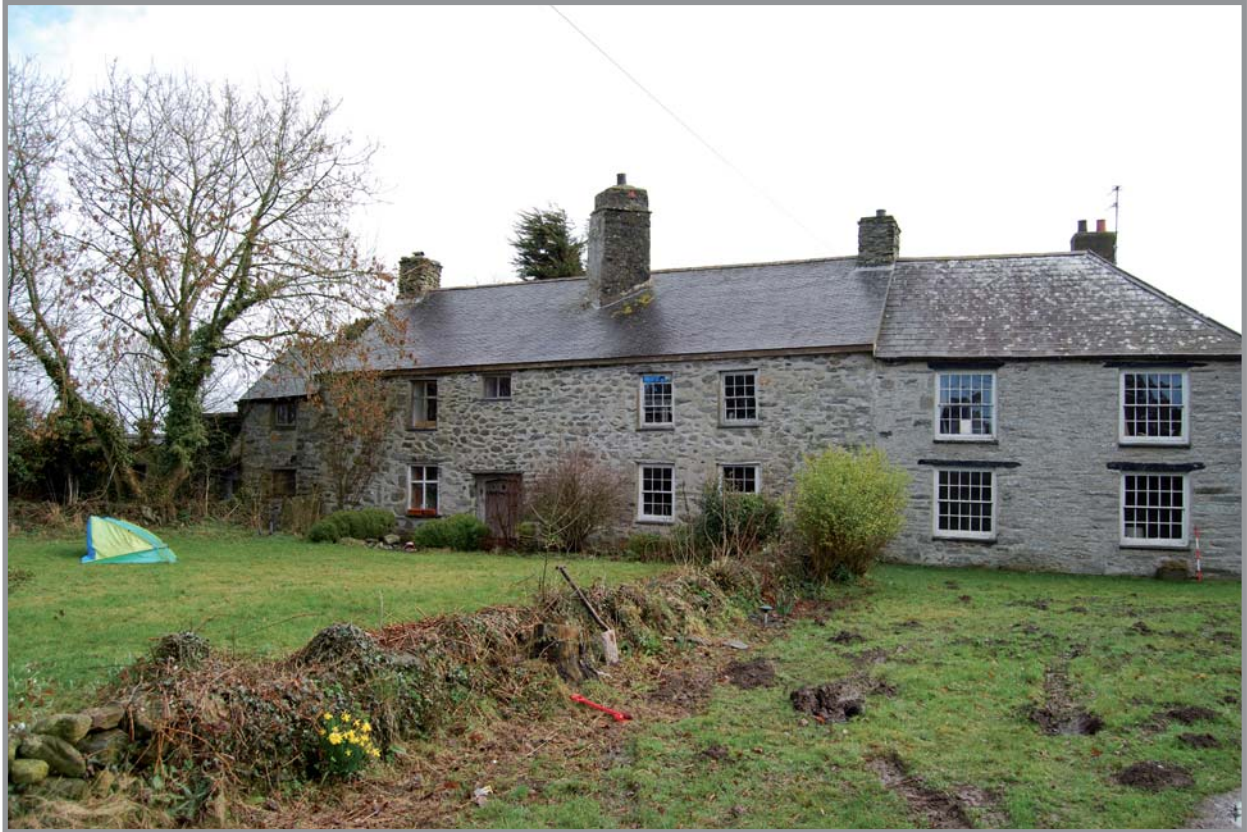
Plate 1: Gronant west facing elevation showing building A to the north and the 19th century infill extension to the south.
