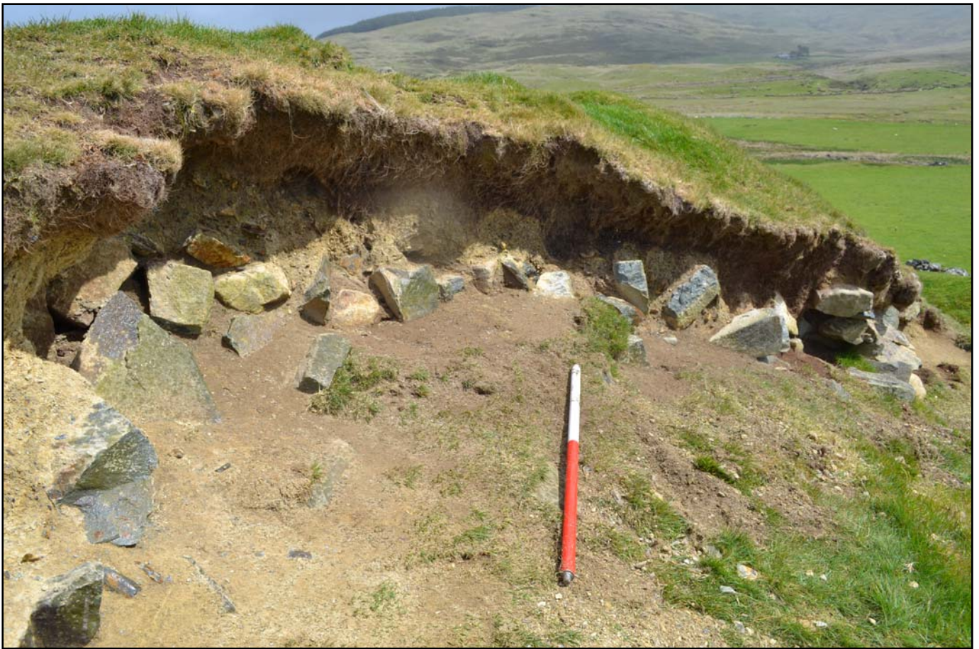
Plate 3: Erosion scar [001] from the west
