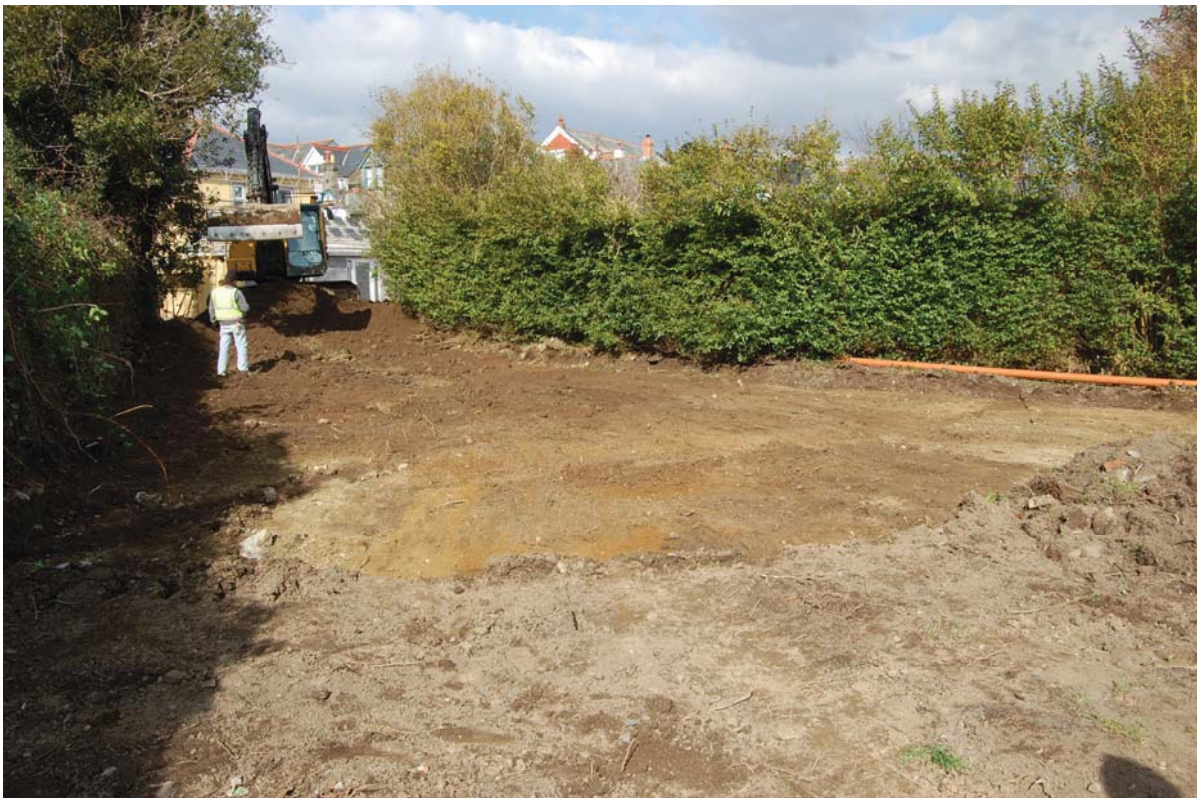
Plate 4 Stripping Area B, view from the East South East
