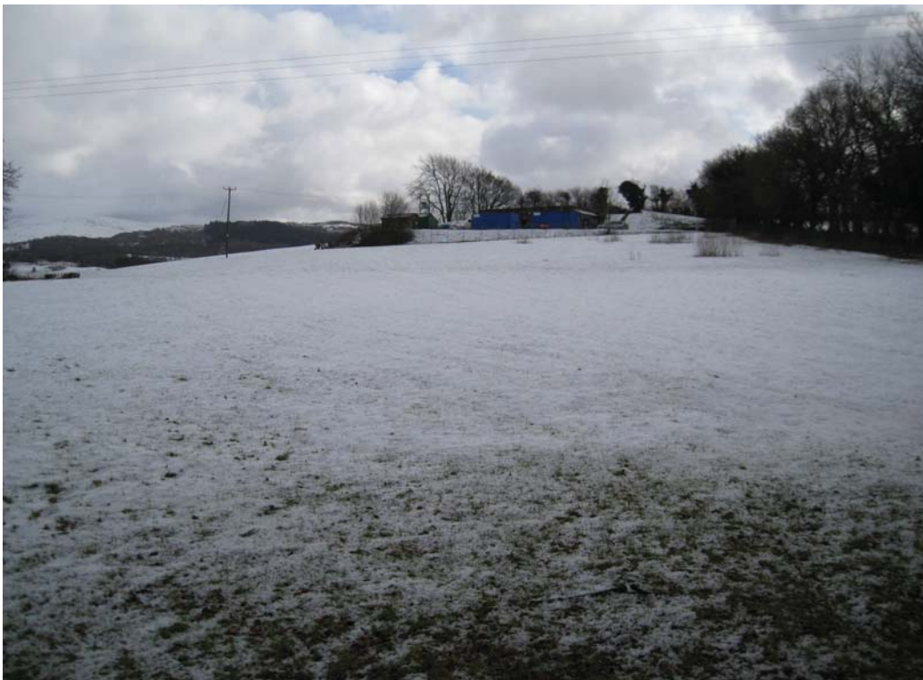
Plate 4 The Water Treatment Works looking south, showing the proposed development area in the foreground, in the field known as 'Cae Hir'
