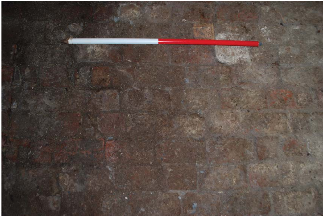
Fig. 9 Detail showing character of brick flooring. Scale 1m with 50cm divisions
