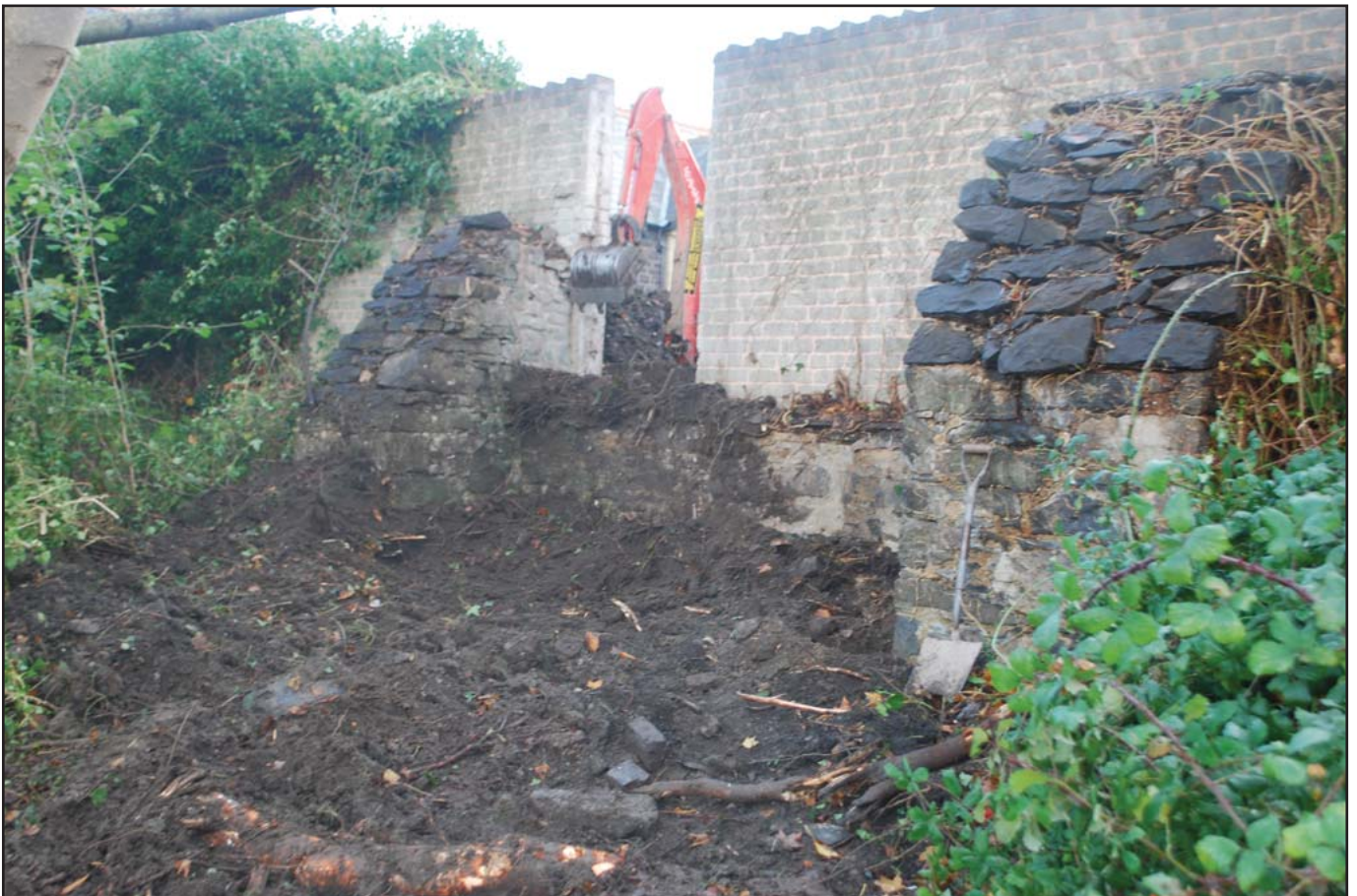
Plate 8: General view of wall area during excavation of soil build up
