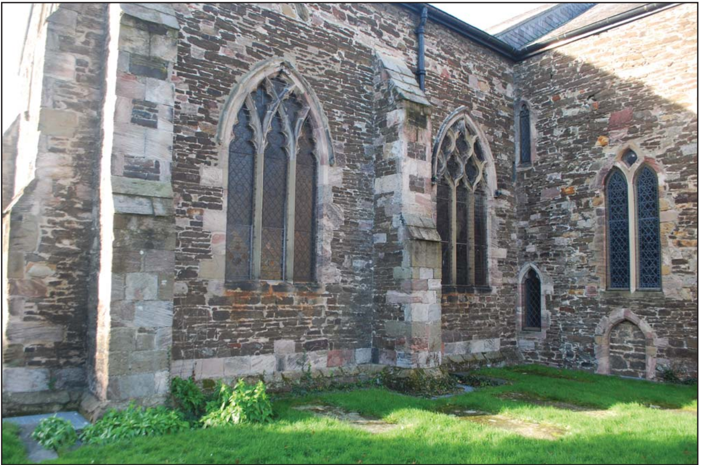
Plate 1: South East corner of South transept of St. Mary's church
