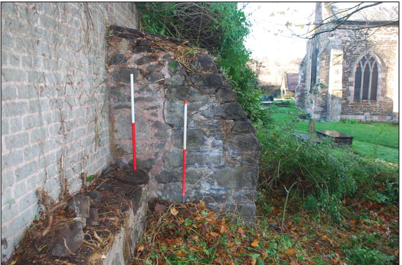
Plate 4: Buttress detail - View from South East - Scales 1m
