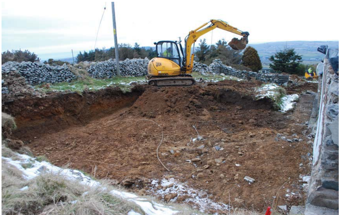
Plate 2 The development plot from the south-west
