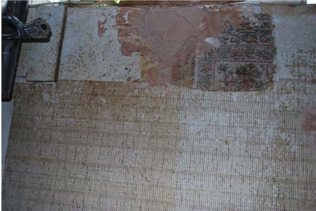
Plate 29 Evidence of early decorative wallpapering scheme in room 1
