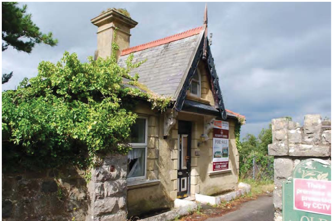
Plate 14 General shot of the Abbey Lodge from the north-east
