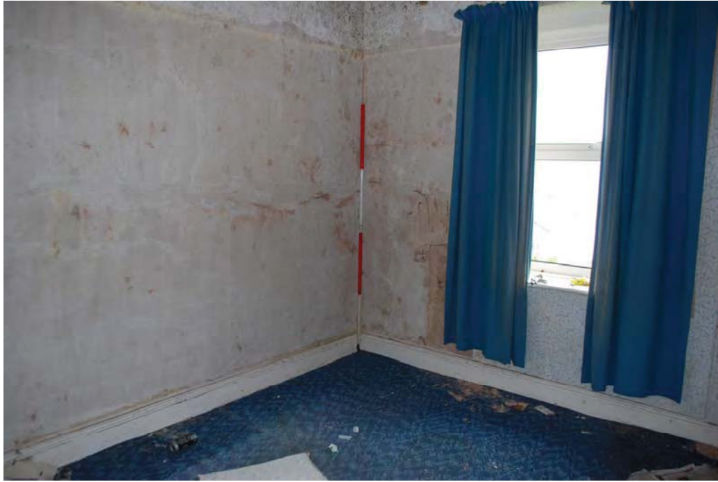
Plate 21 Room 4 with uPVC window. Scale 2m
