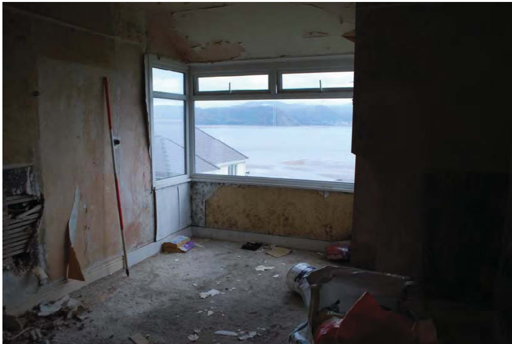
Plate 20 Bay window in Room 3. Scale 2m
