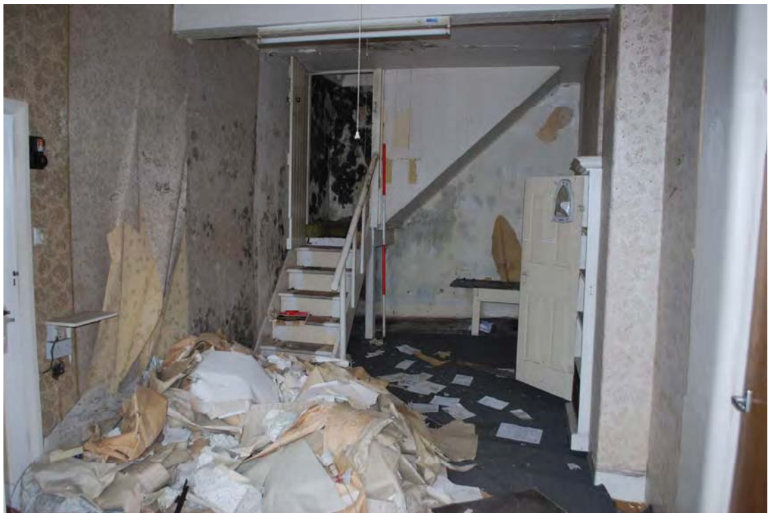
Plate 22 Room 5 showing late 19 th century stair and cupboard
