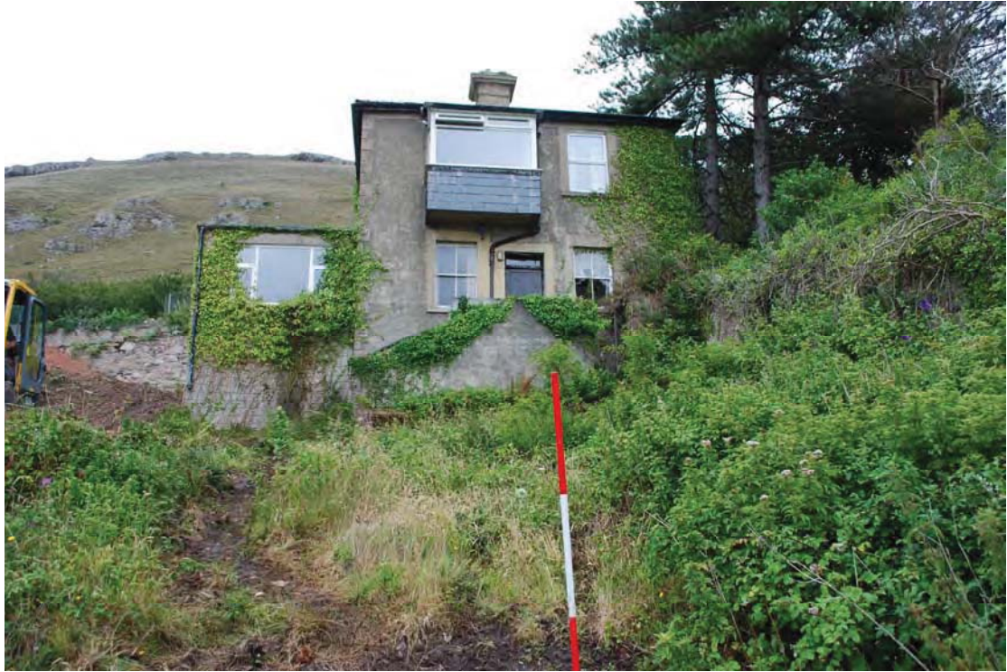
Plate 31 The rear, south facing elevation to the Abbey Lodge. Scale 2m
