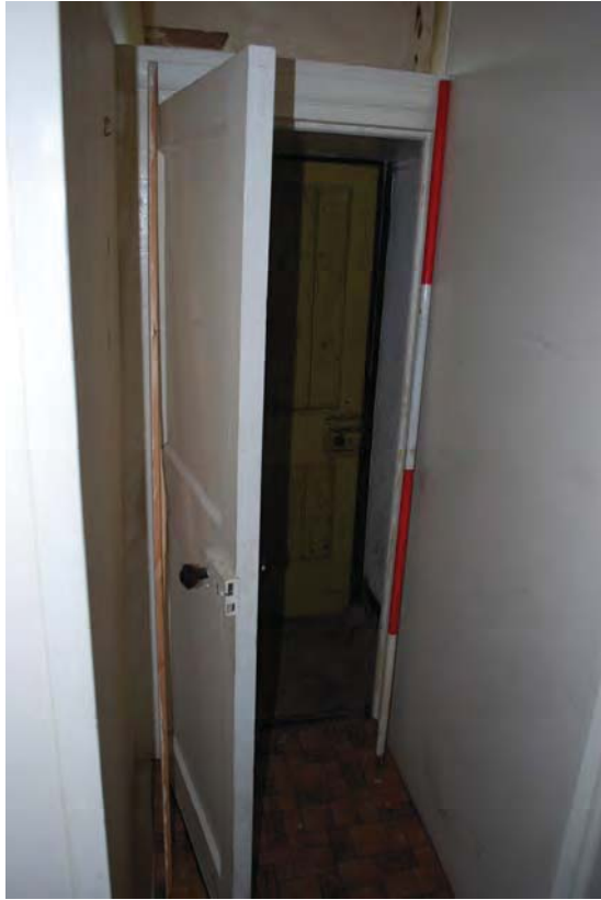
Plate 27 The rear door to the Abbey Lodge. Scale 2m
