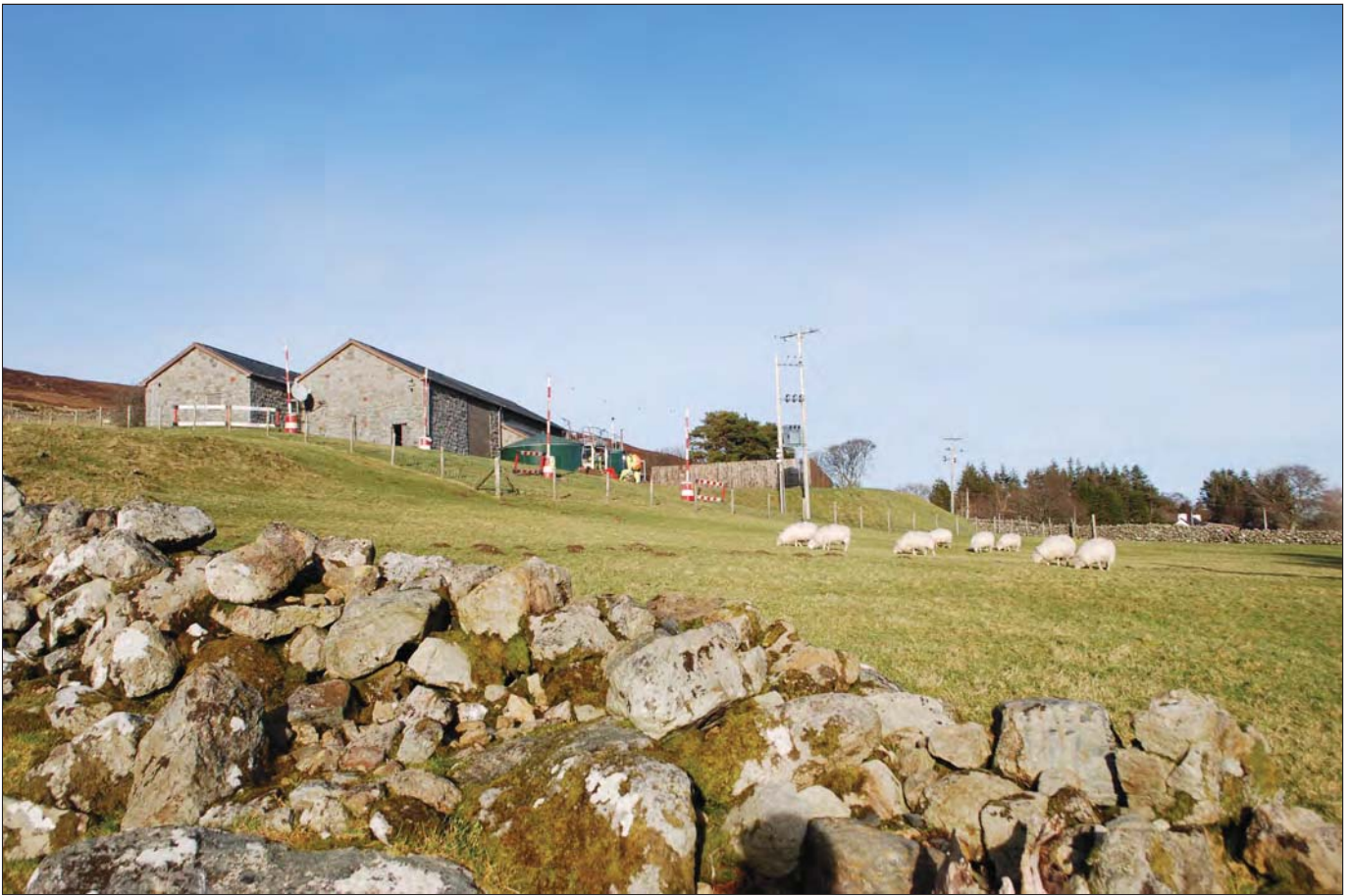
Plate 5 View of the Water Treatment Works from the west showing north-south slope and terracing, with Feature 3 in the foreground. Scale 1m
