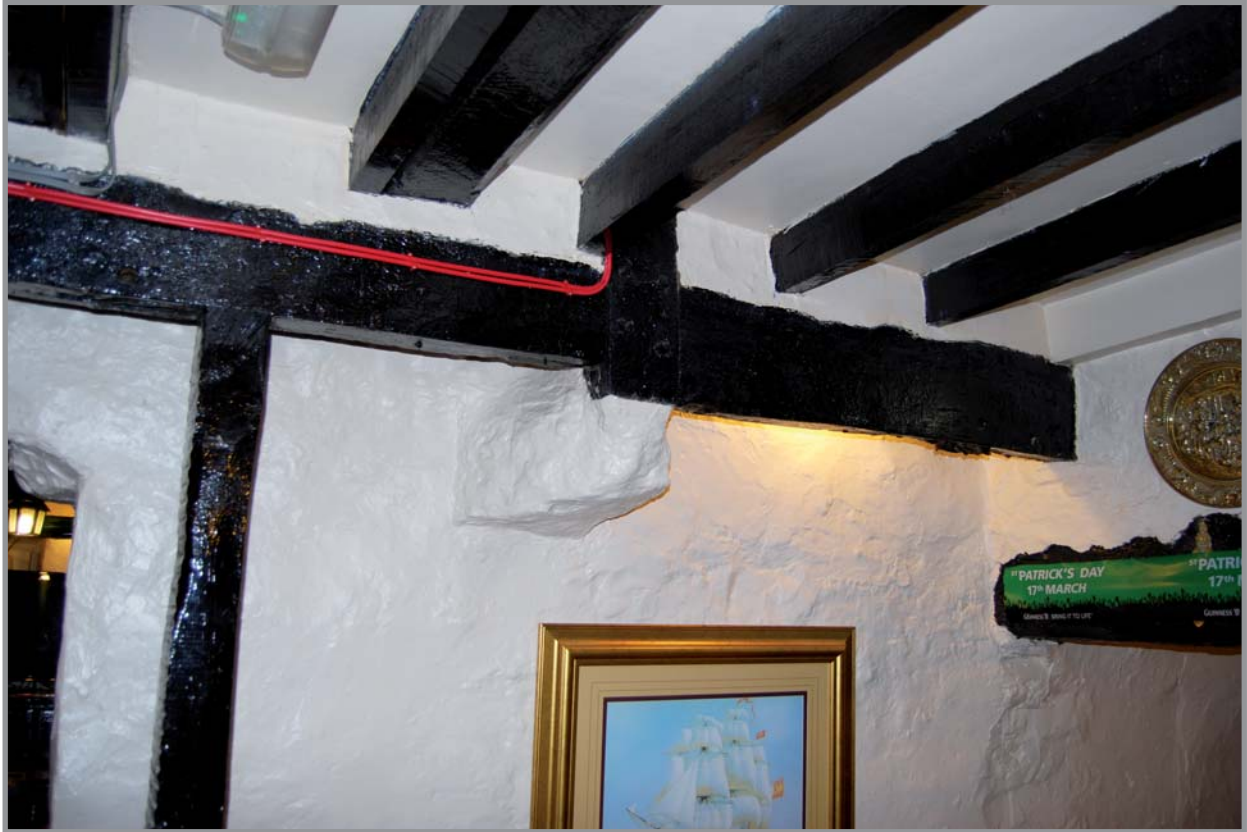
Plate 15: Stud wall with wall plate supported on stone corbel, facing east
