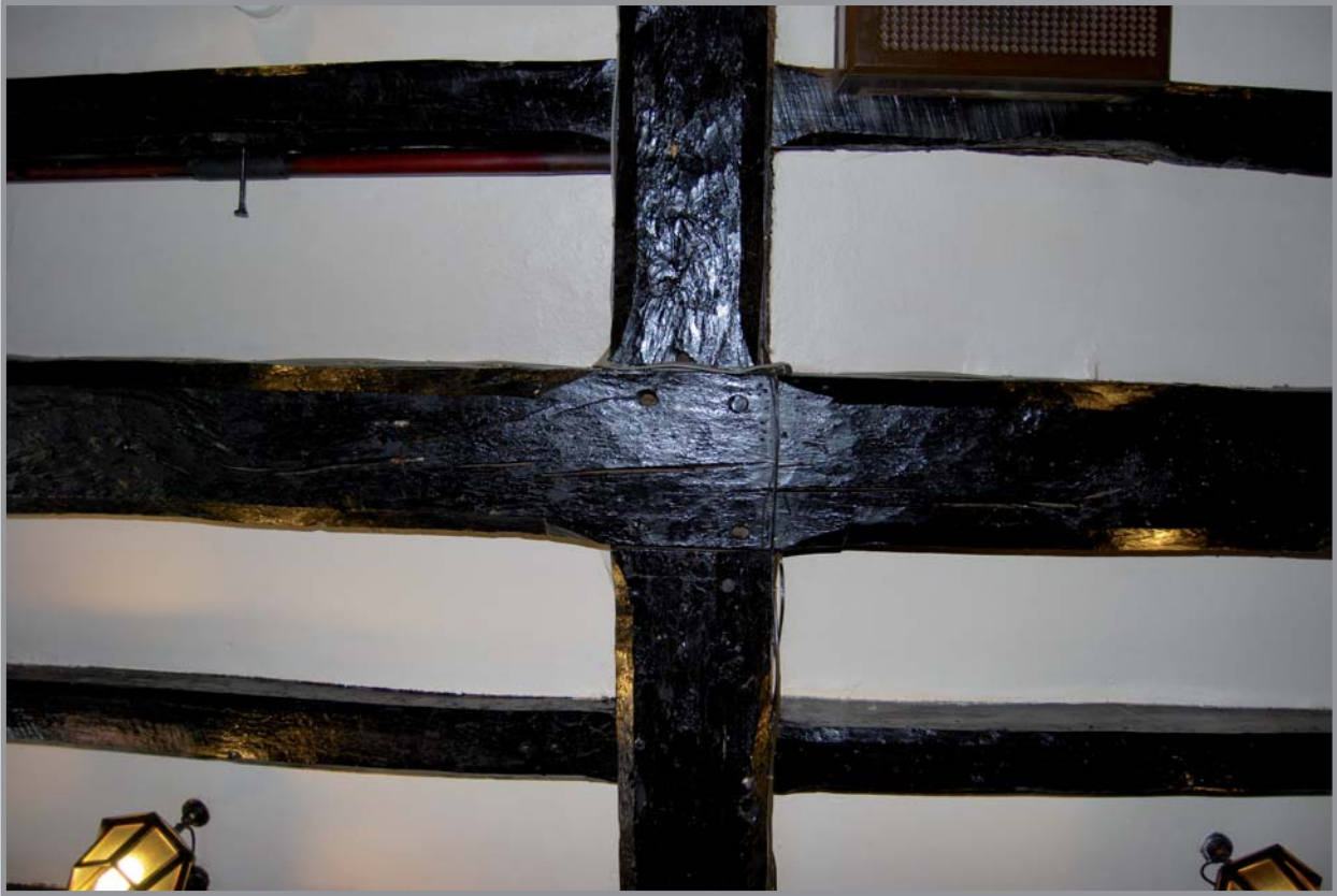
Plate 11: Image showing axial beam and transverse beam
