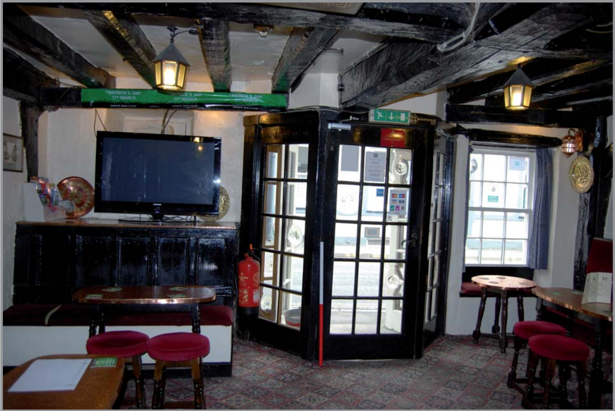
Plate 9: East elevation, showing transverse beam 1, axial beam, blocked window and modern door.
