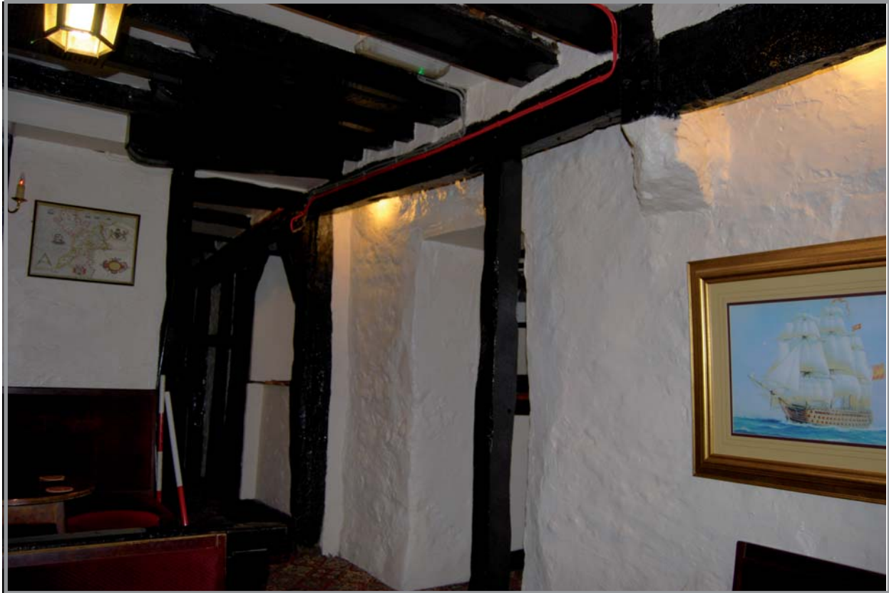
Plate 13: Image showing stud wall with protruding jetty beams above, facing north
