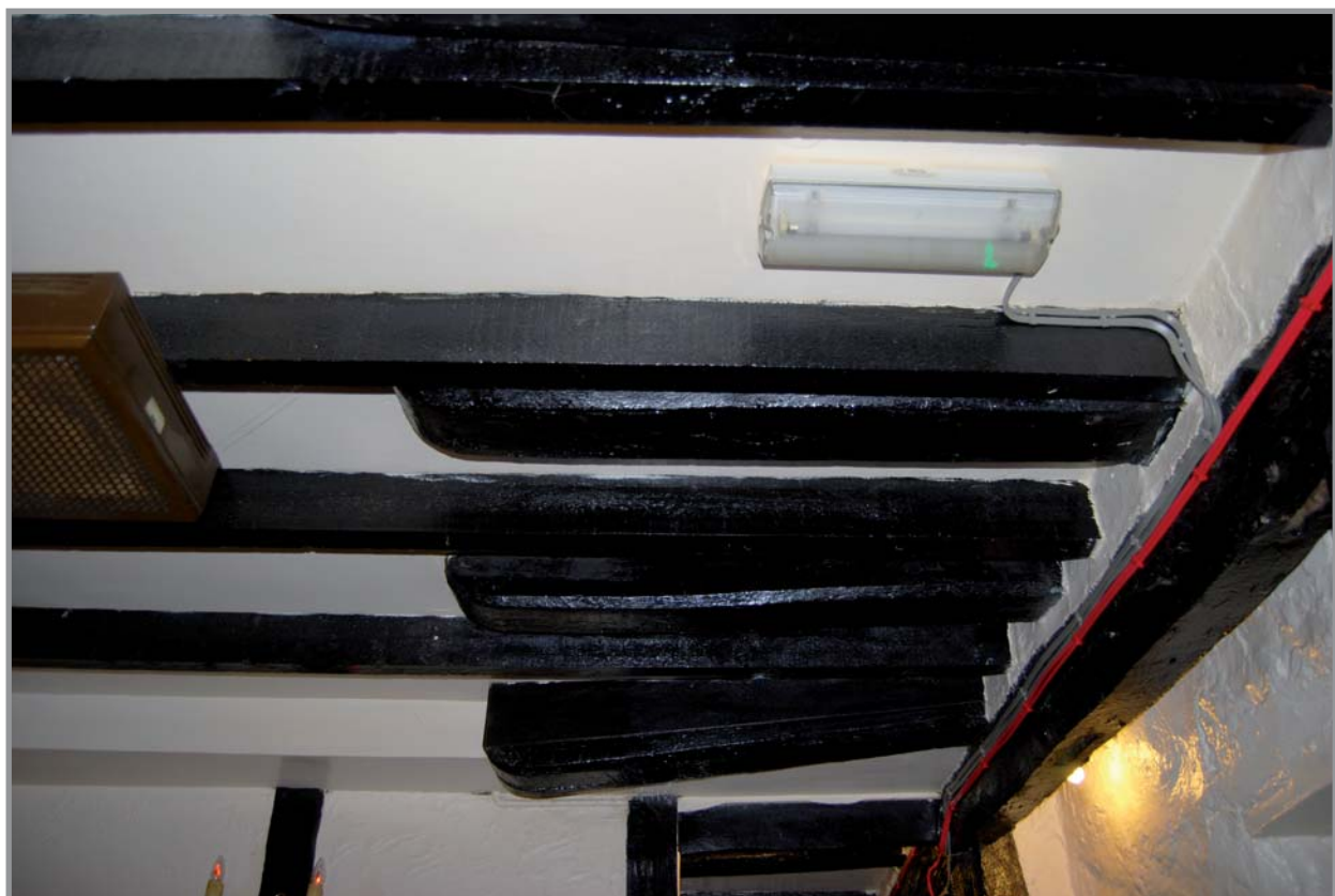
Plate 14: Jetty beams
