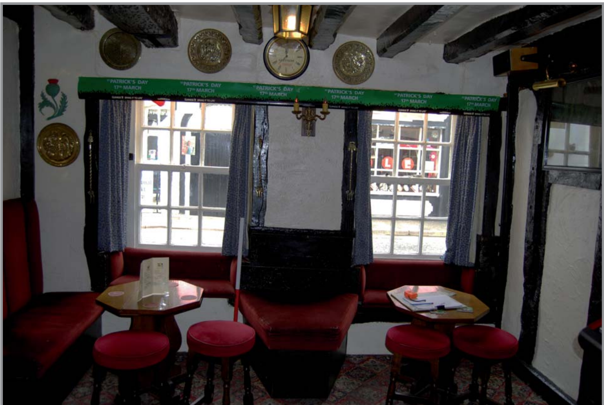
Plate 6: West elevation showing two 12-pane sash windows. Facing east
