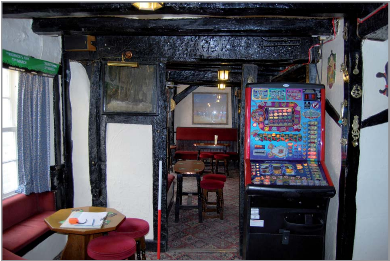
Plate 7: Original wall division between the southern and northern properties, showing original wattle and daub and curved bracket. Facing south
