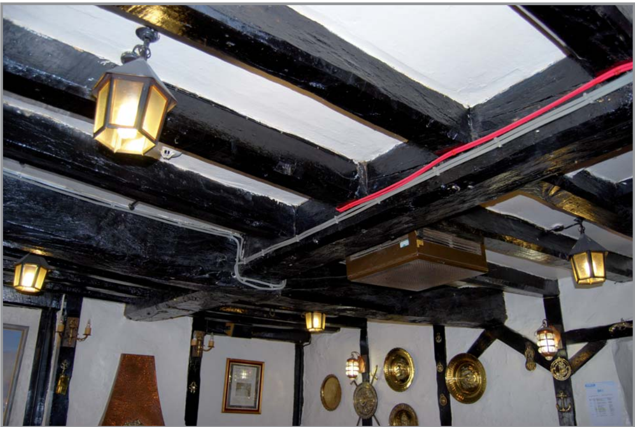
Plate 12: Image showing axial beam
