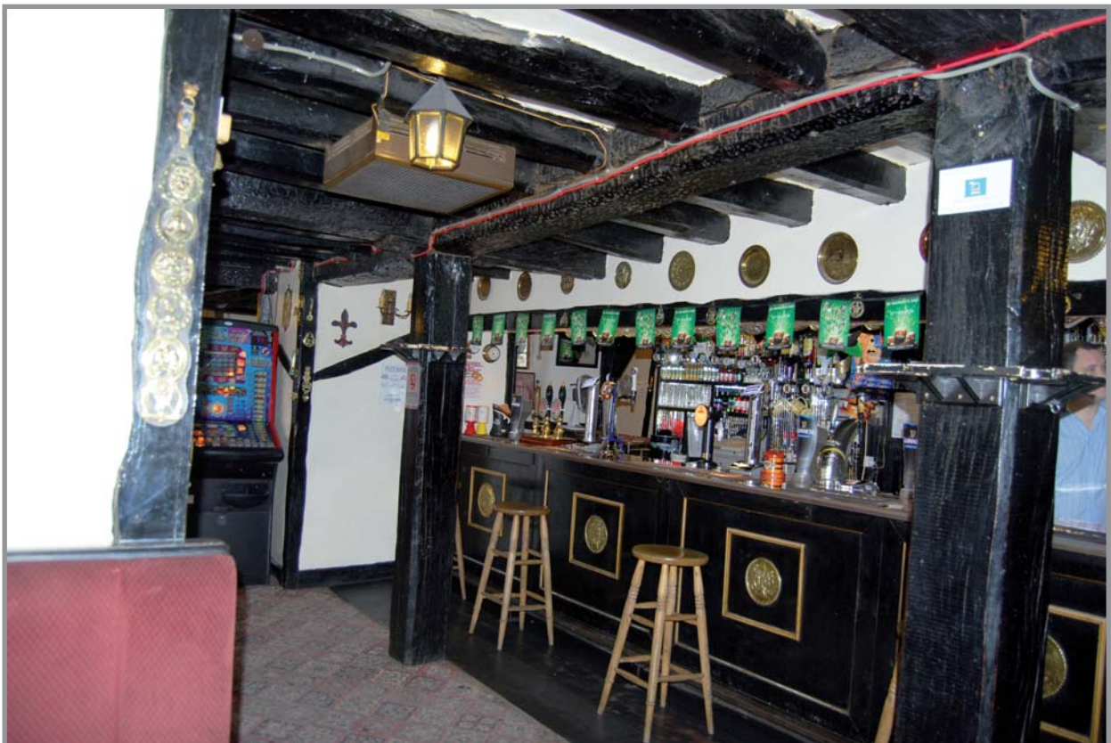
Plate 4: Image showing upright posts supporting axial beam. Facing south-west
