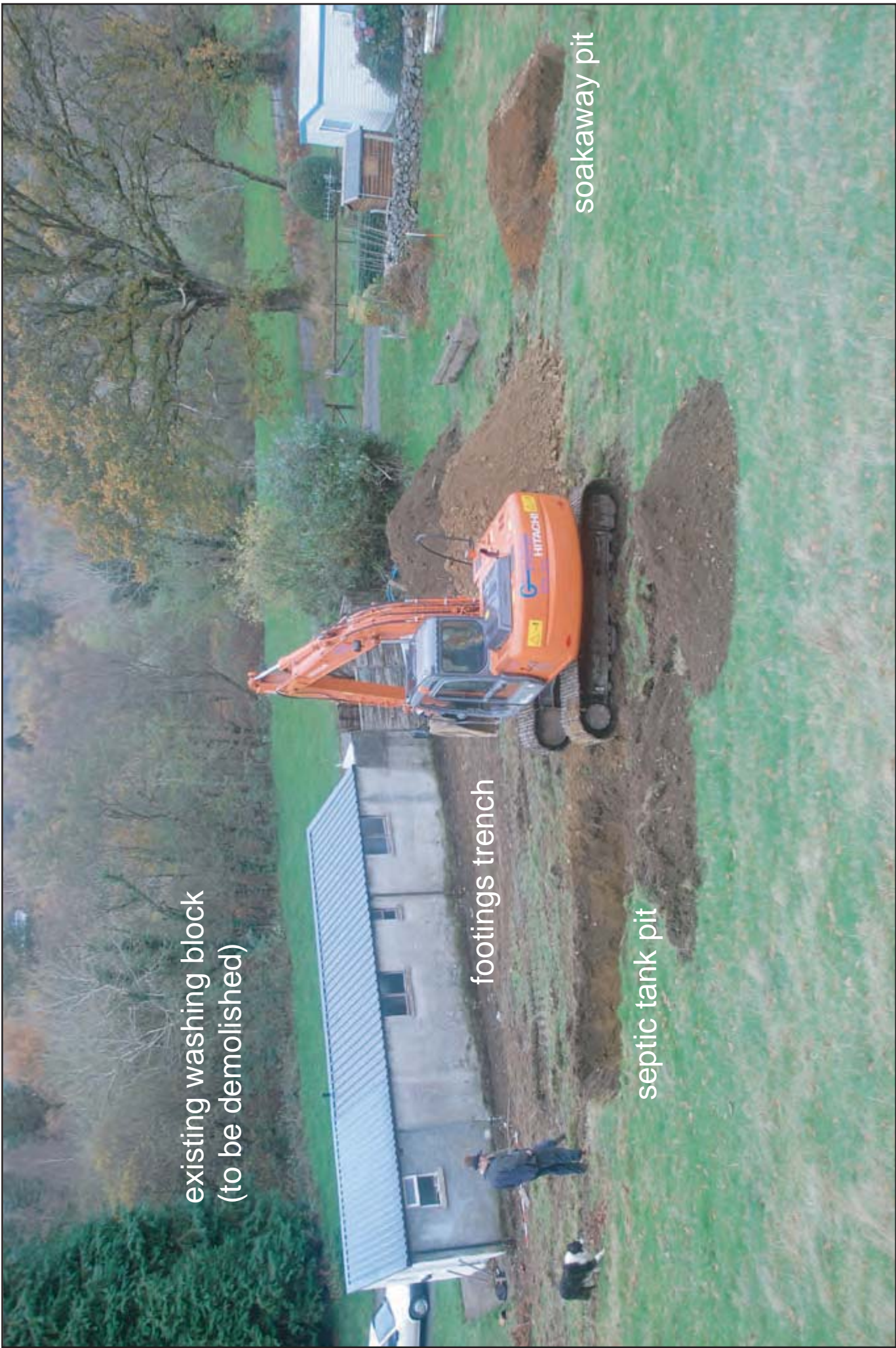
Plate 01: view northwest of development area, detailing extent of groundworks monitored by the watching brief. The existing washing block demolition does not form part of the watching brief. A service trench will also be dug between the septic tank pit and the soakaway pit.
