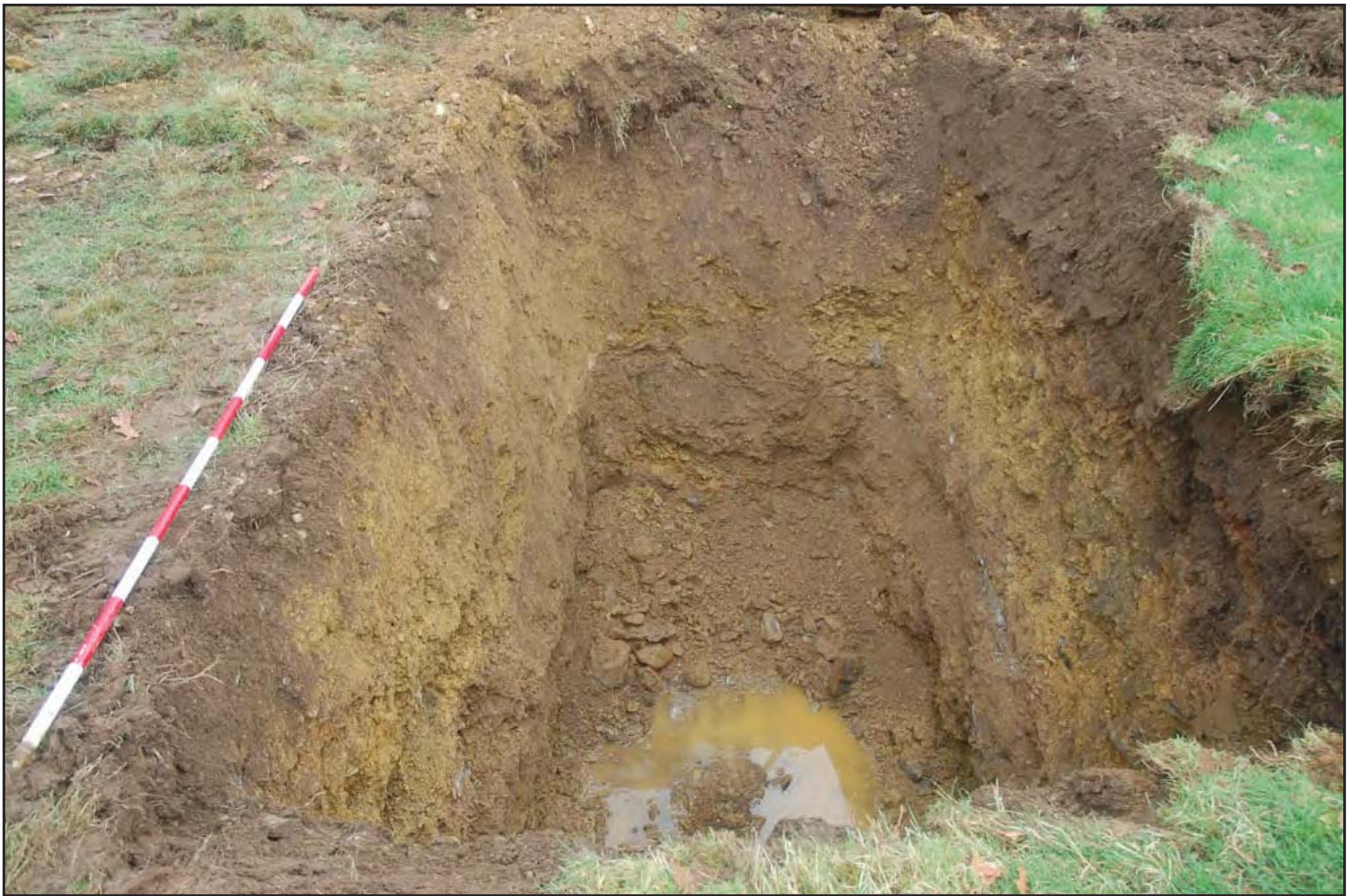
Plate 04: view north of the septic tank excavation detailing limit of excavation. The pit was excavated into a slope and comprised topsoil of varying thickness followed by two distinct glacial deposits (ranging pole: 2.0m)
