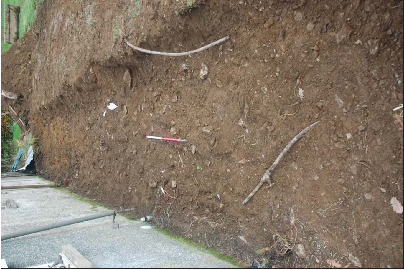
Plate 02: view north of washing block footings during excavation. Note the modern disturbance associated with the construction of the existing block (ranging pole: 1.0m)
