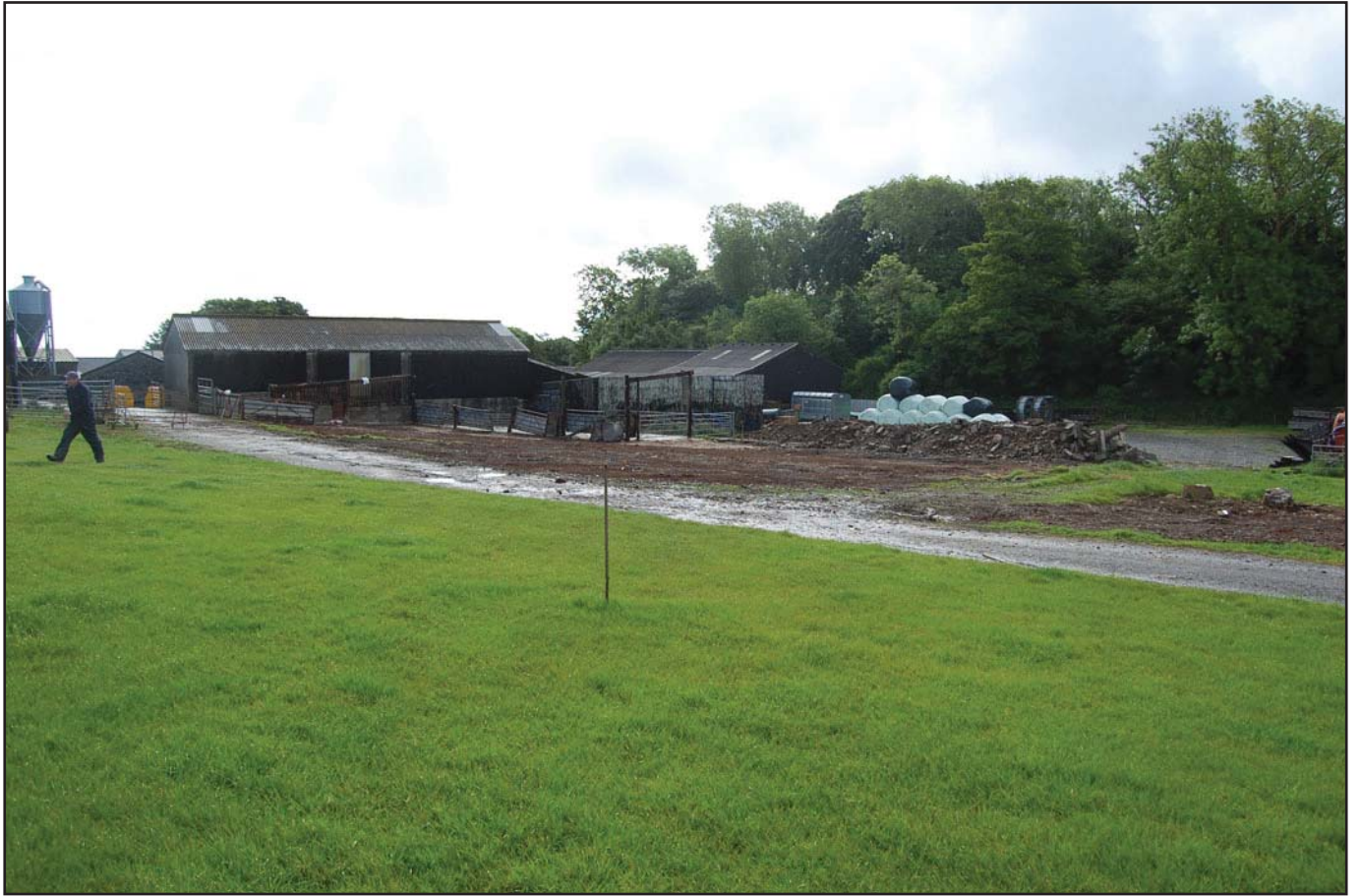
Plate 2: Pre-excitation shot of the site following the removal of the previous structure (view from the east).
