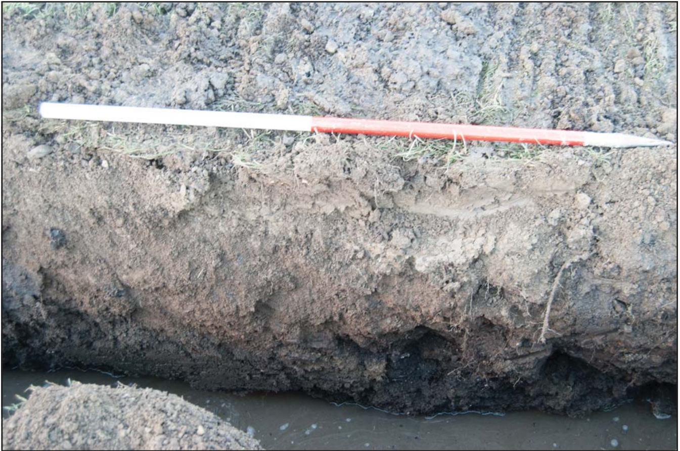
Plate 03: South facing section of trench by first transformer (east side of site). View from south;1x1m scale.
