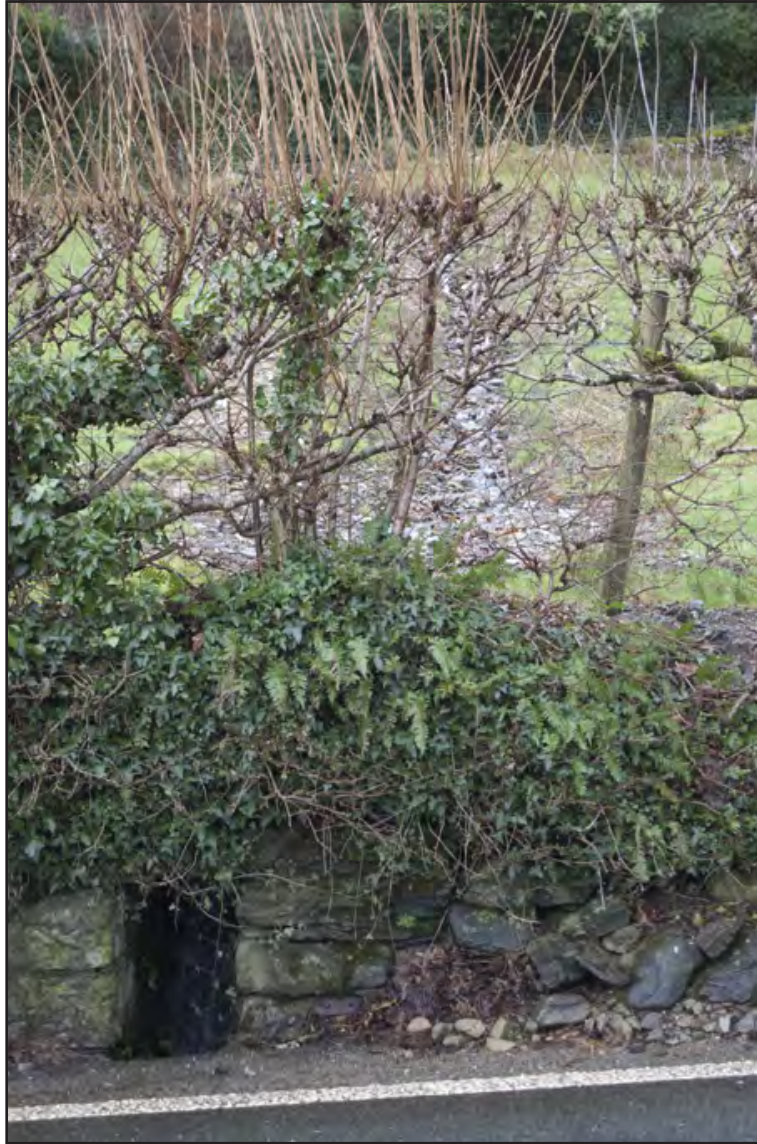
Plate 09: Section B-C: View southwest of modern drainage channel [Feature 3]
