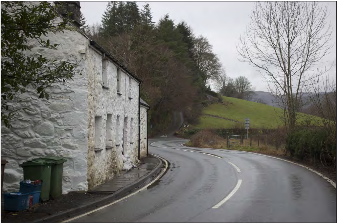
Plate 11: Section B-C: View west along street showing pipeline route in pavement, showing point where route crosses sloping field
