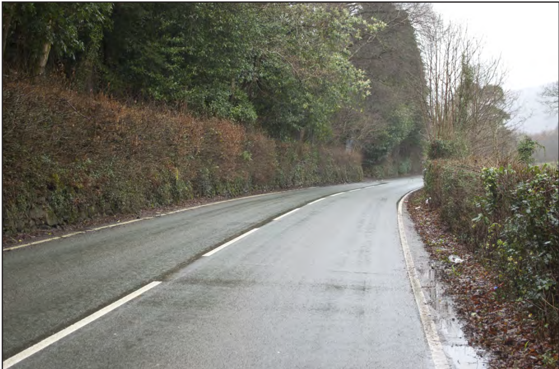
Plate 10: Section B-C: View west along street showing pipeline route in pavement
