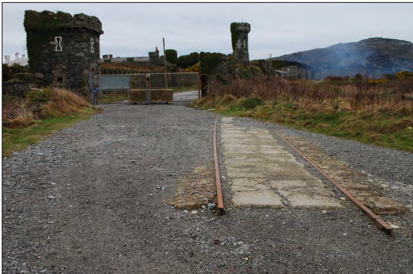
Plate 17: Holyhead Breakwater - view from northeast detailing surviving remnant of rail at landward end of hardstanding/building area (archive image: G2498_001).
