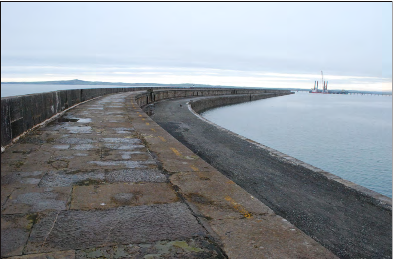
Plate 16: Holyhead Breakwater - general view from the southwest looking from the upper parapet (archive image: G2498_047).
