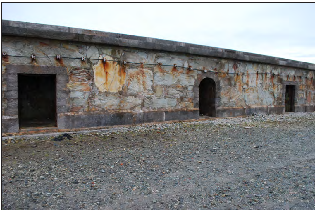
Plate 20: Holyhead Breakwater - view from southwest of three barrel vaulted refuge chambers (archive image: G2498_010).
