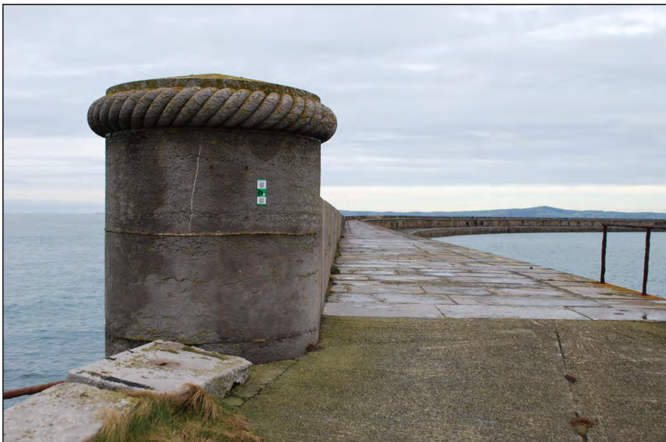
Plate 18: Holyhead Breakwater - view from southeast of large stone drum with roped design at end of the parapet (archive image: G2498_003).
