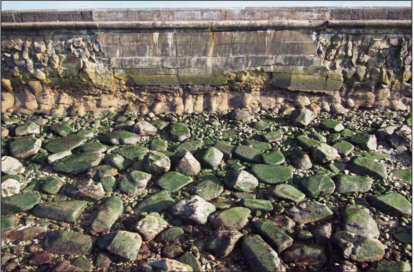
Plate 07: View of mid - 20th century concrete repairs to the seaward side of the breakwater, with the upper slabs molded to resemble original ashlar masonry of the parapet (sourced from Civil Engineering Solutions: 20150928 Holyhead Breakwater 193.jpg).
