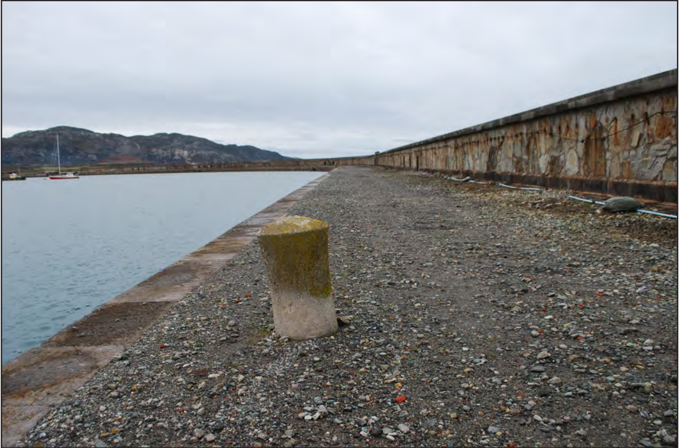
Plate 21: Holyhead Breakwater - view from east of bollard for tying up vessels; located along lower breakwater walkway (archive image: G2498_013).
