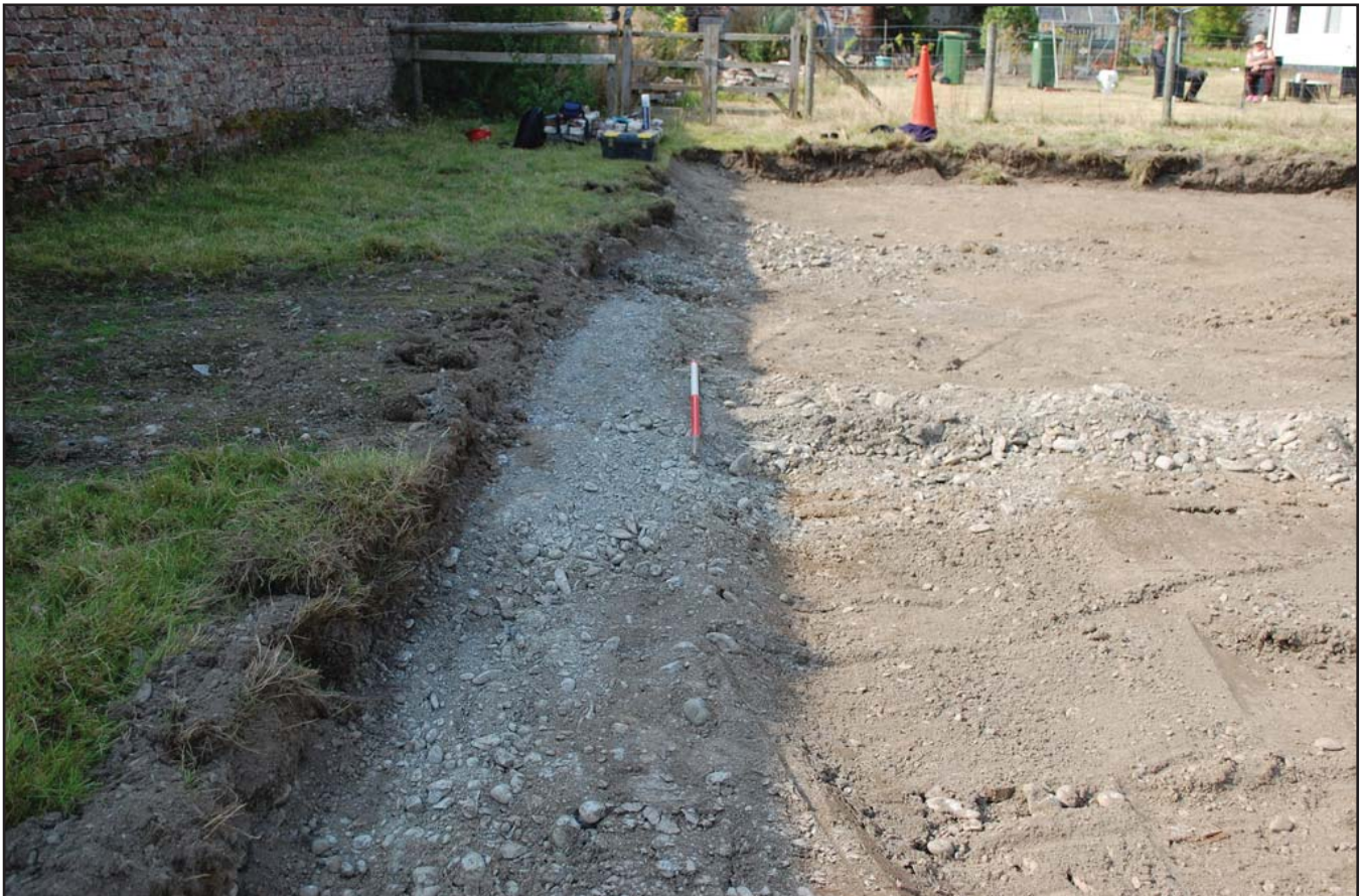
Plate 12: Garden path, context [003]. Scale 1m, viewed from the south-east.
