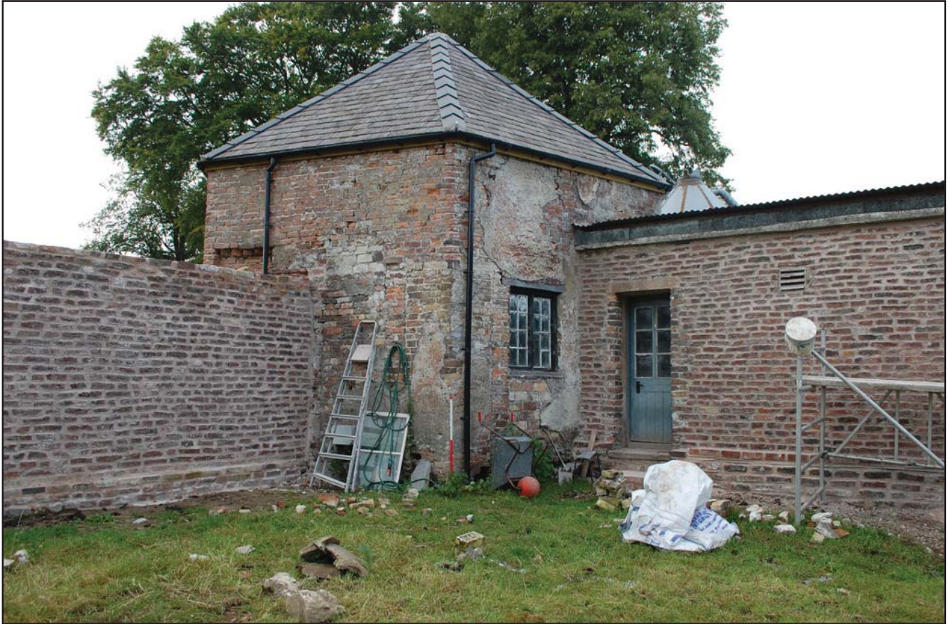
Plate 07: Square in plan building. Scale 1m, viewed from the north.
