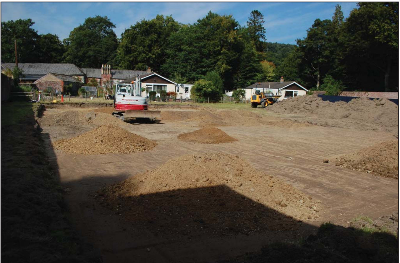
Plate 16: Area of tennis court levelled, viewed from the south-east.
