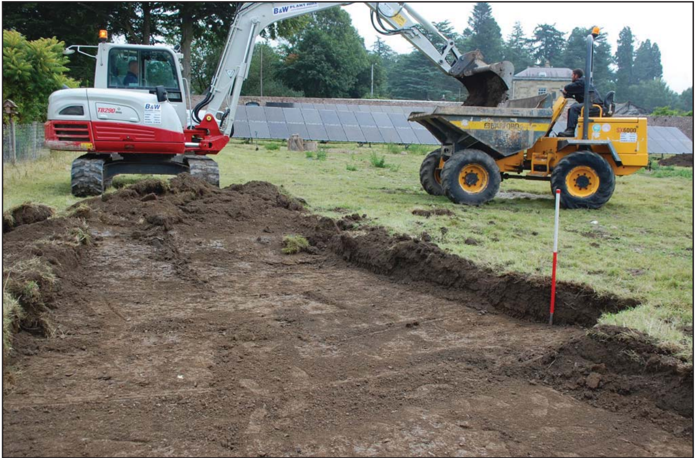
Plate 11: Topsoil strip of tennis court. Scale 1m, viewed from the south-west.
