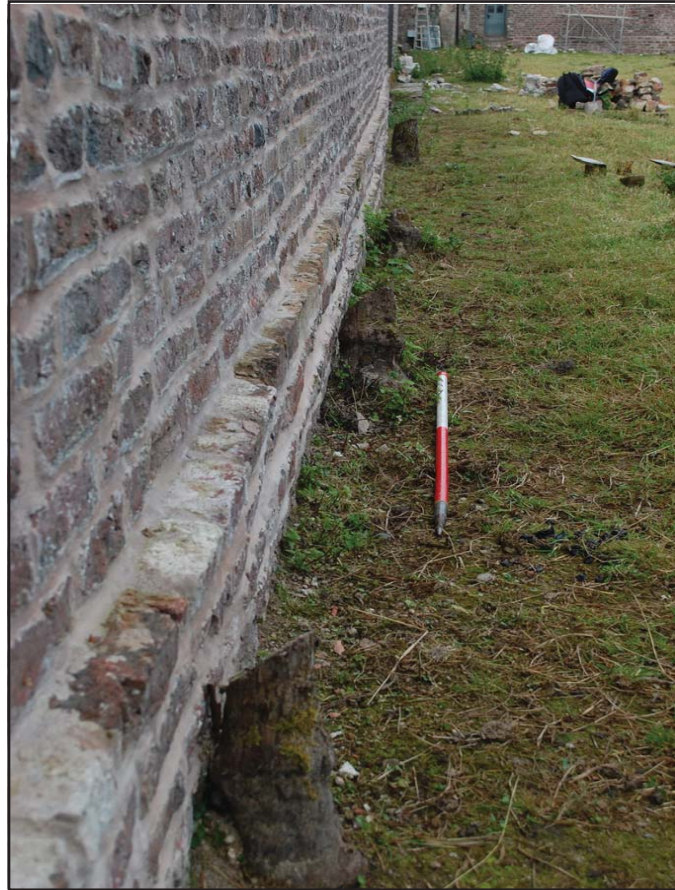
Plate 03: Tree stumps along the base of the eastern wall. Scale 1m, viewed from the north-east.
