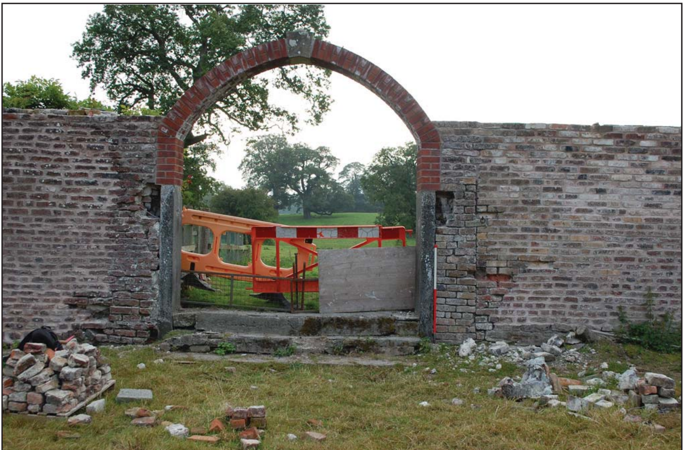
Plate 04: Arch within the eastern wall. Scale 1m, viewed from the north-west.
