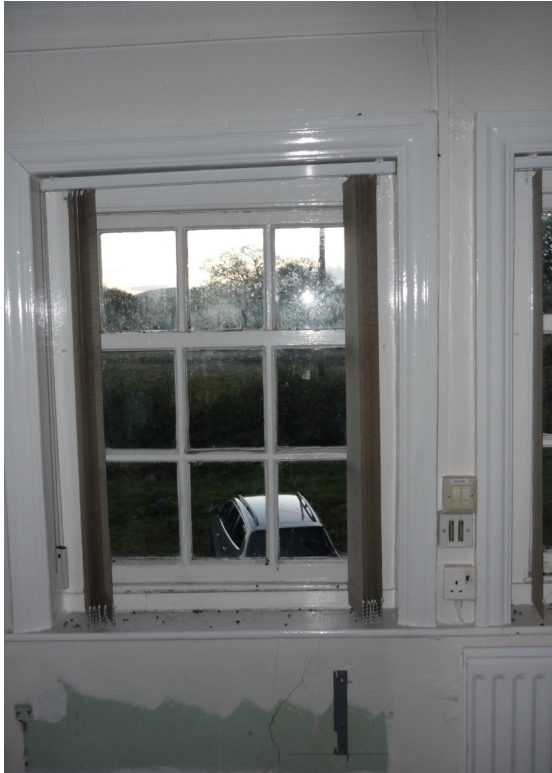
Typical First Floor Window (17)
