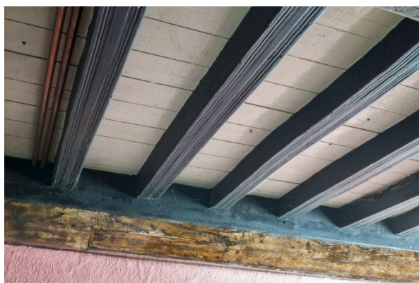
Figure 5 – Reed Moulded Joists to floored hall DS2014_112_014 (Crown Copyright. All rights reserved)
