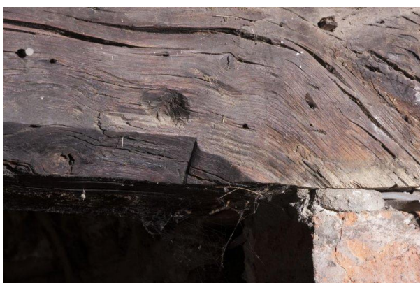
Figure 8 - Chamfer and Ogee stop to bressummer DS2014_112_013 (Crown Copyright. All rights reserved)
