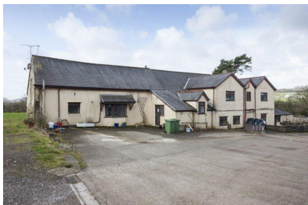
Figure 19 – Rear elevation of Tal-y-fedw and barn. DS2014_112_001 (Crown Copyright. All rights reserved)
