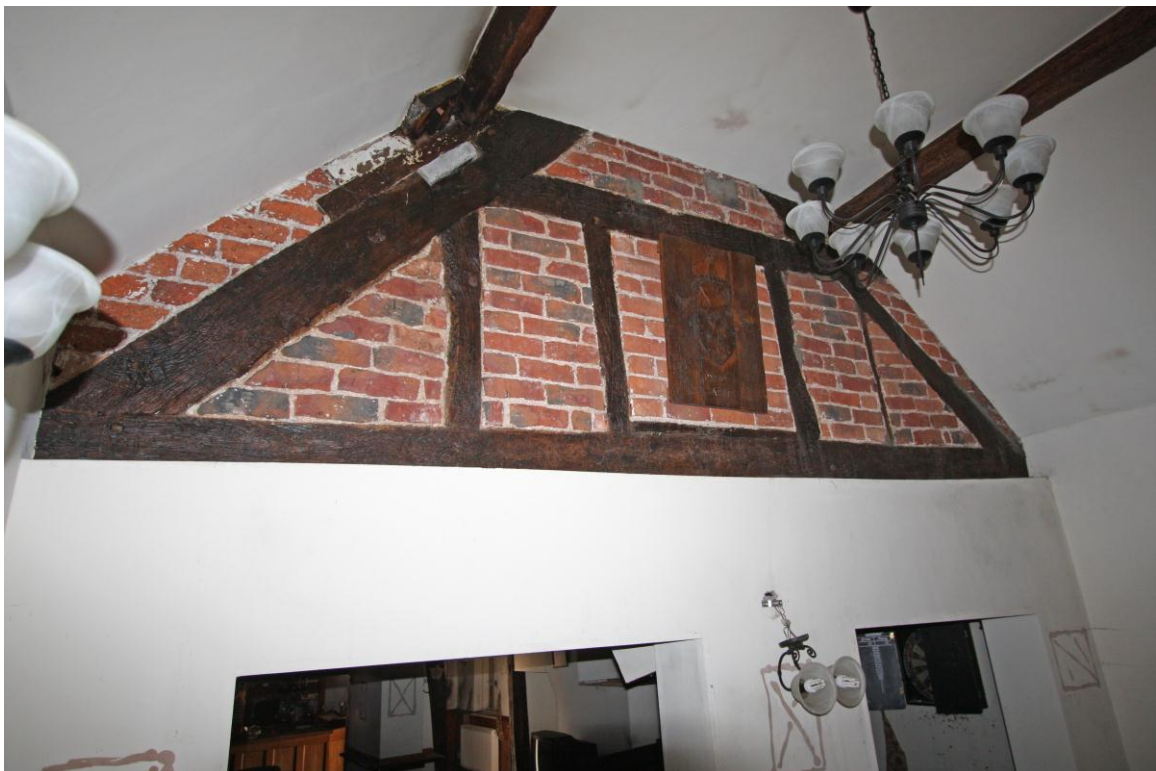
Cowhouse/stable end truss, from former outside.
