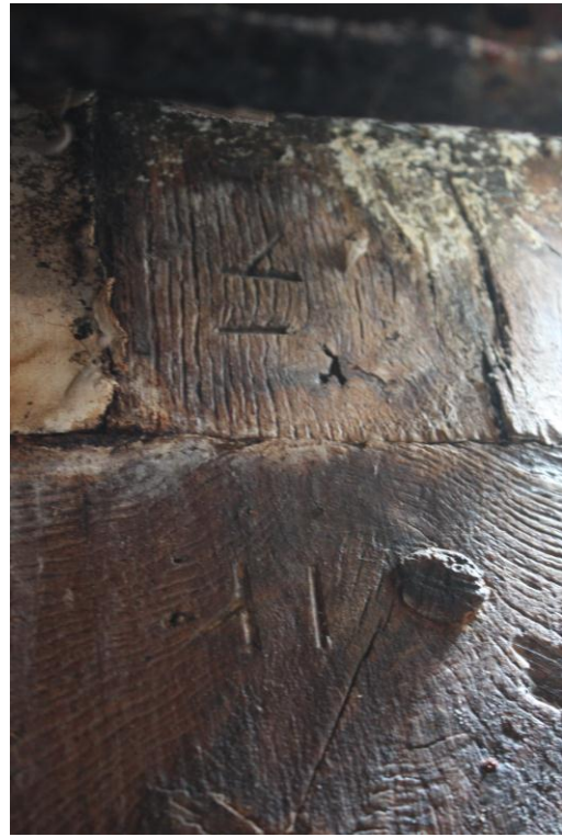
Assembly marks to truss partition in hall
