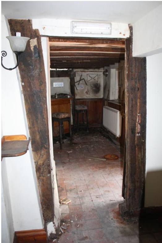
Re-used timber studs, in doorway beside fireplace, viewed from former cow-house/stable, and to right hand, stud with groove for wattle, with head mortices for a doorway.
