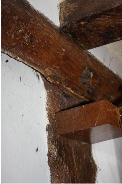
Hall side beam supporting joists.
