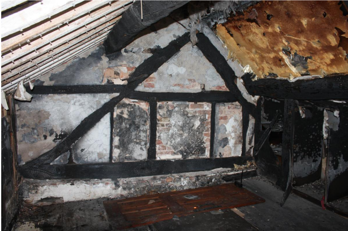
Cowhouse/stable end truss, from inside.
