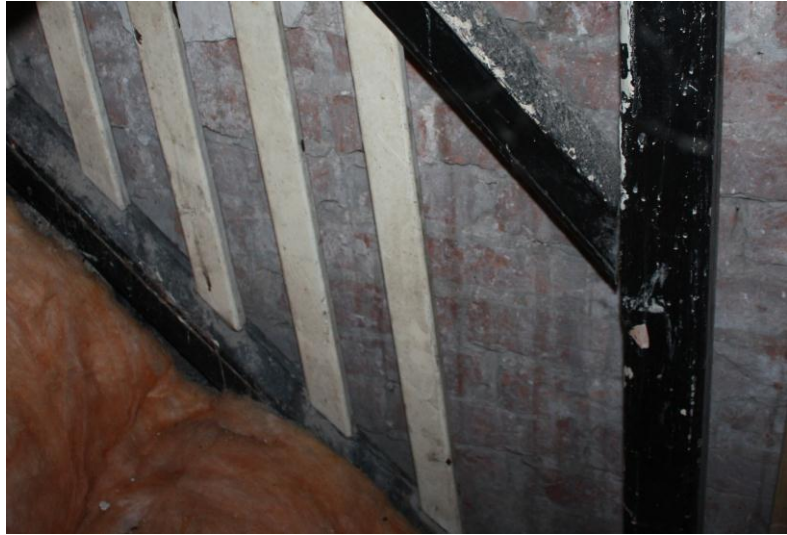
Stair in former cow-house/stable, against the front wall.
