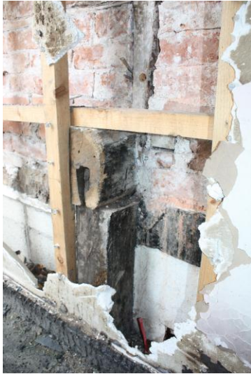
Post & cut-back tie-beam.
