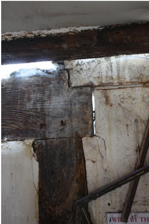
Chamfered doorway to stud in partition.
