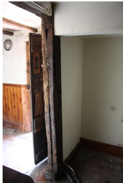
Re-used timber studs, in doorway beside fireplace, viewed from former cow-house/stable, and to right hand, stud with groove for wattle, with head mortices for a doorway.
