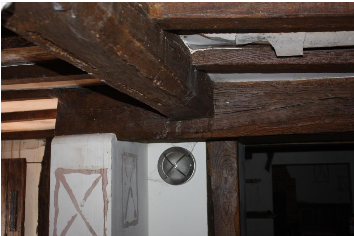
Hall fireplace bresummer, with ceiling-beam and joists
