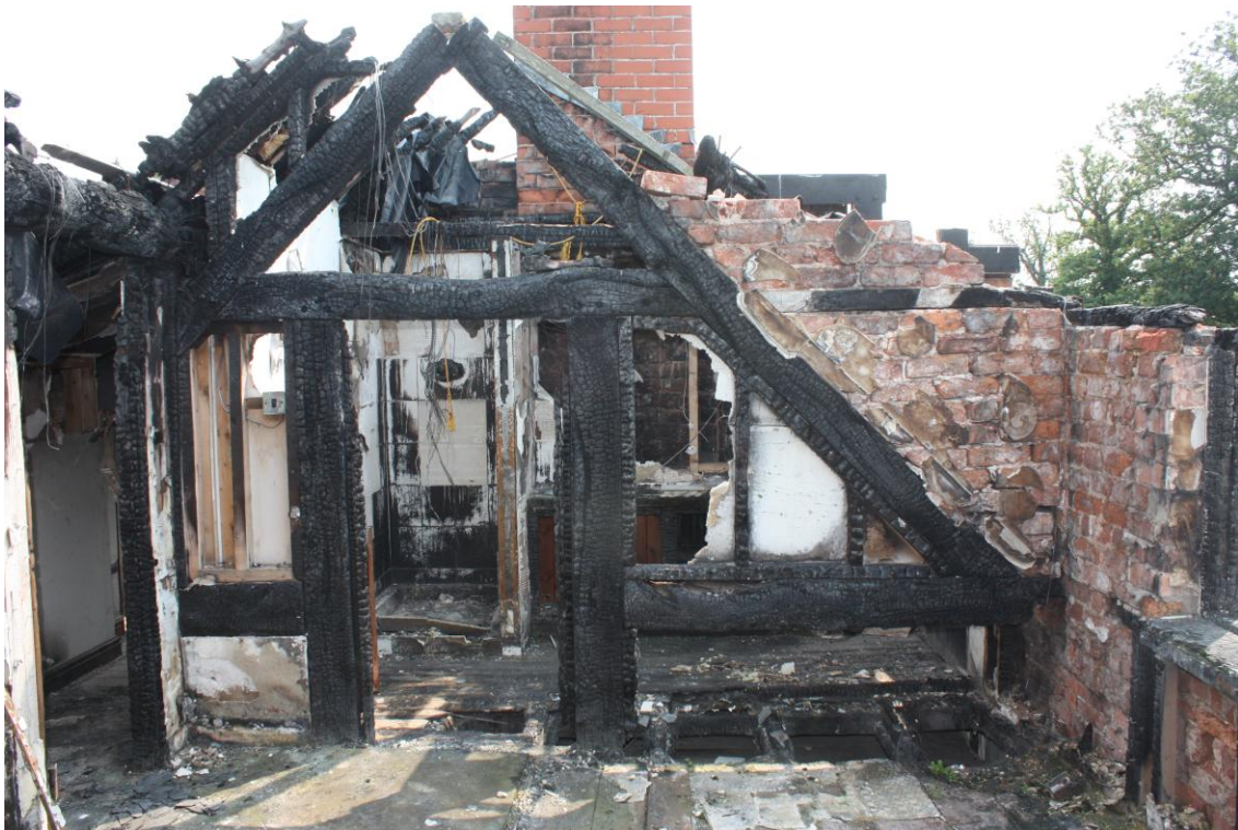
Interrupted tie-beam truss between hall and inner-room at first-floor.
