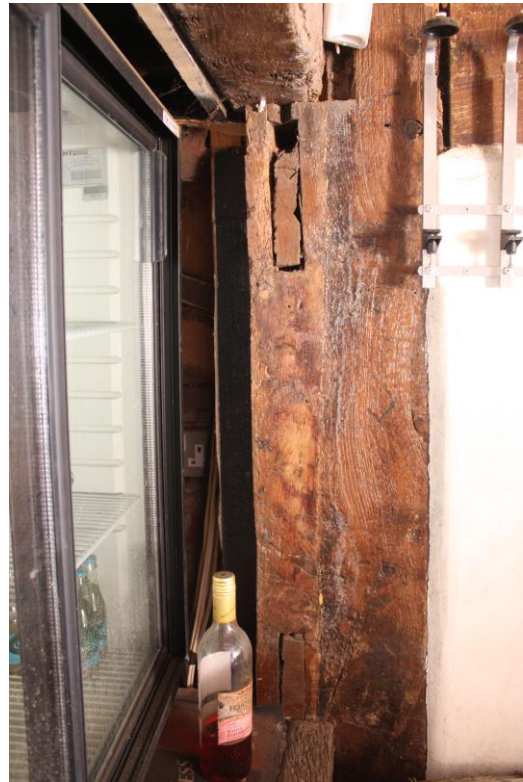
Partition post with mortises to square framing.
