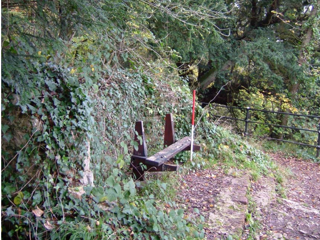
Photo. 1. The Alcove with modern bench inside the historic structure.
