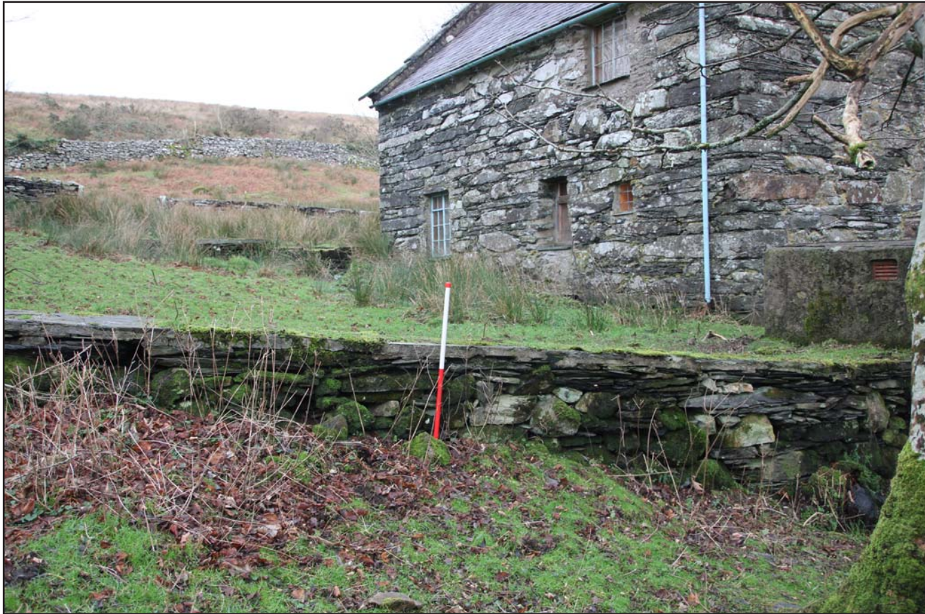
Plate 07: Revetment wall feature 3, from the southeast. Scale 1.0m.
