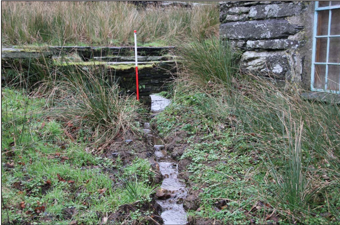
Plate 08: Run-off from Pool 1 to Pool 2 (feature 4), from the southeast. Scale 1.0m.
