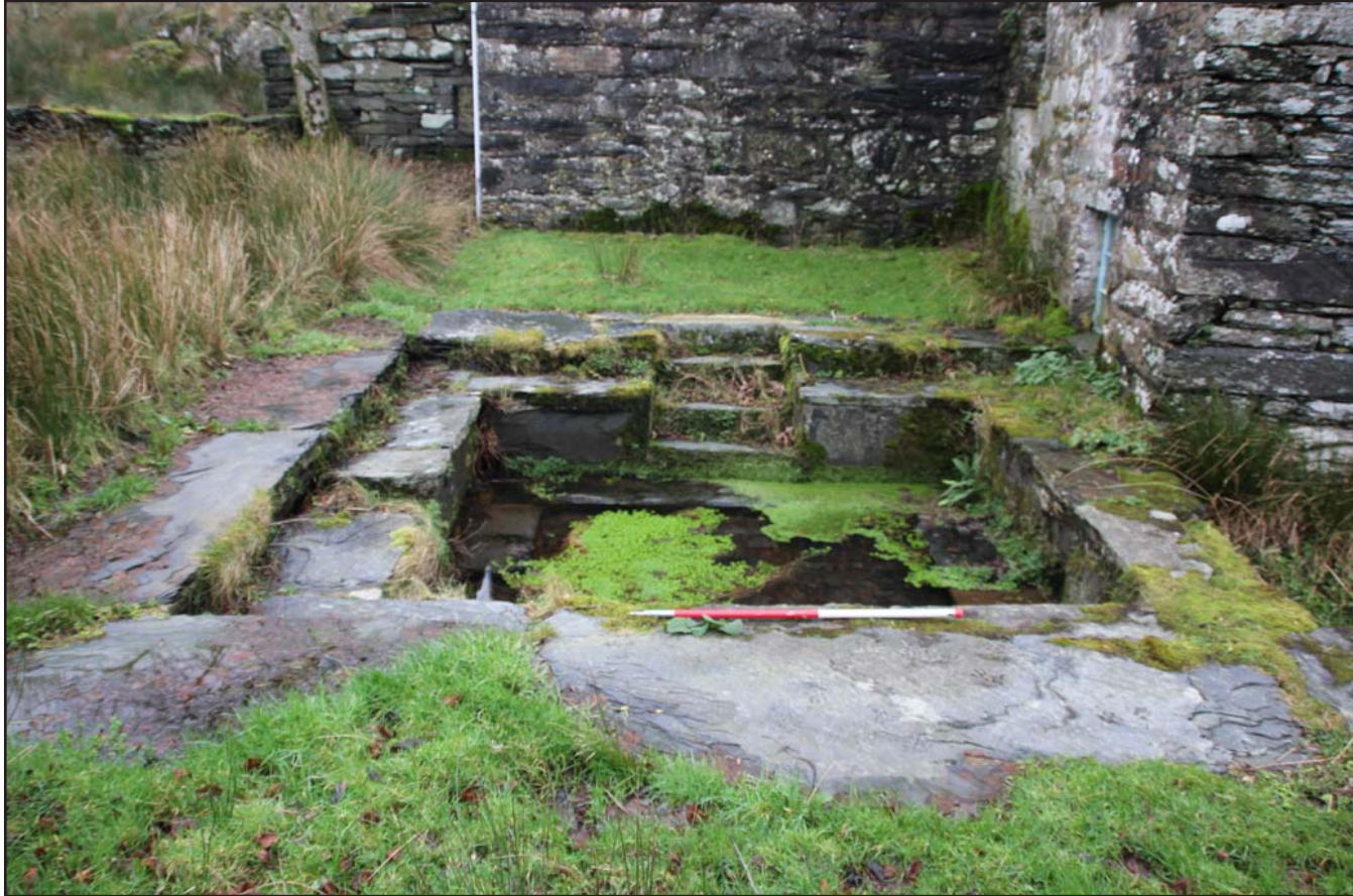
Plate 02: Square pool 1 from the southwest. Scale 1.0m.
