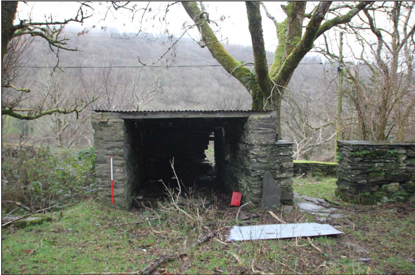
Plate 12: Garage feature 8, from the northwest. Scale 1.0m.
